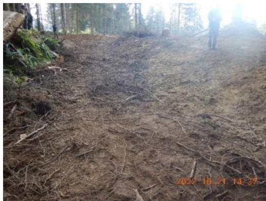
Figure 51. The new road construction to area F not only pushed fill further towards the watercourse, but also cut down into the adjacent hillsides. View looking upslope into clearing, spanner is on the left of photo.
