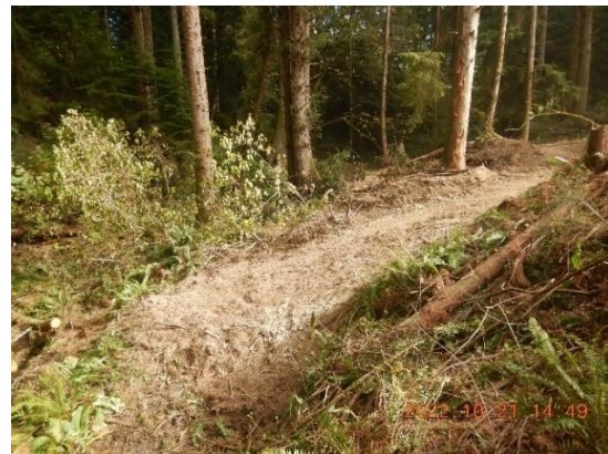
Figure 39. New road constructed to area D, included cut and fill from clearing to watercourse at WP979 for 48' from the crest to the stream.
