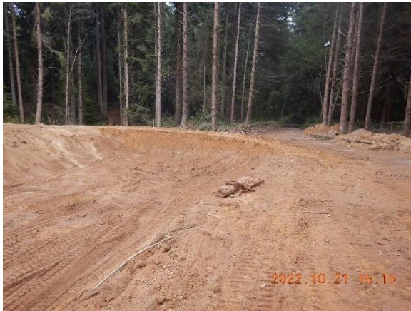
Figure 12. Looking downslope to pond berm.
