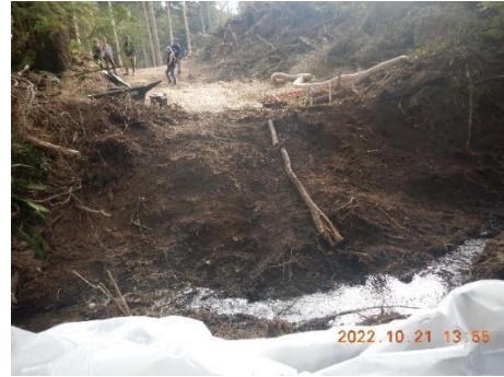
Figure 37. View of area A from right bank. The channel form has been impacted by the instream work to place and remove the stumps.
