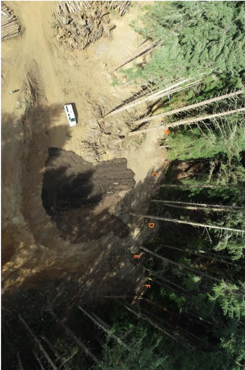
Figure 3. Drone image collected by SHN on day of inspection (10/21/22) and submitted on 10/23/22. Locations B-F correspond to the locations identified in Figures 1 & 2.
