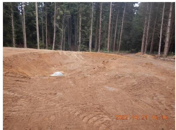
Figure 11. Overview of pond, looking downslope toward stream, with inlet pipe in foreground, with berm in
