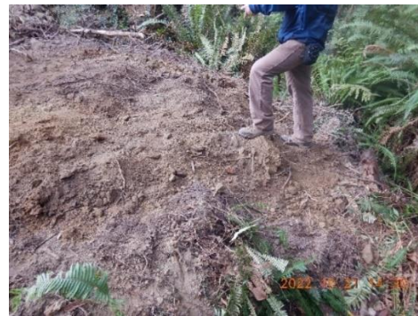
Figure 52. The fill at area F buried the channel for 14' long, and an estimated 3' deep.
