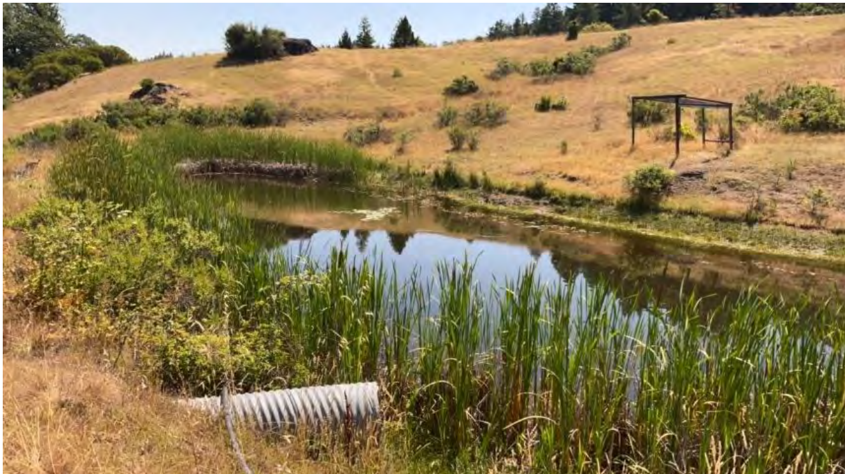
Figure 13. Polygon Feature 10 – onstream pond with piped outlet with approximately two feet of free-board at the berm.
