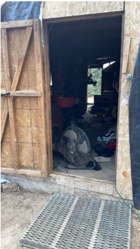
Figure 121. Building at location 4.
