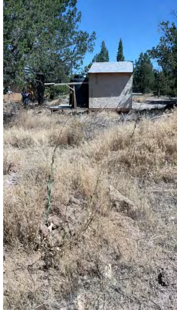
Figure 40. Toilet waste at location 7 is released via a line to the ground.
