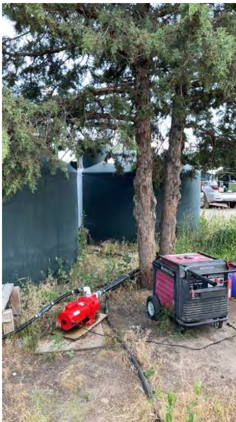
Figure 97. Water storage and pump at location 9.
