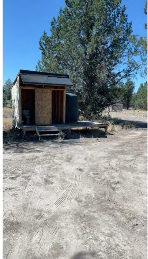
Figure 38. Toilet shed at location 7.
