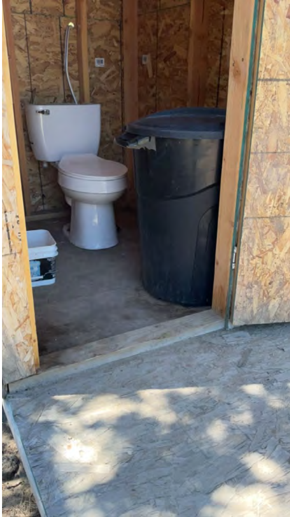
Figure 39. Toilet in shed at location 7.
