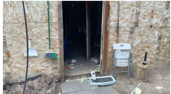
Figure 102. Dwelling building at location 3.
