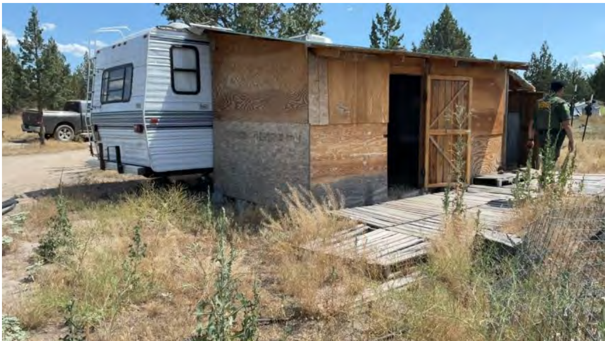
Figure 93. Building connected to an RV at location 6.
