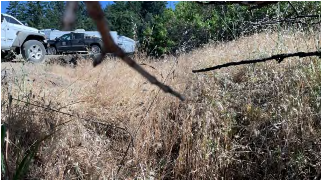
Figure 15. Line 8. Road-runoff delivers to a Class III watercourse.
