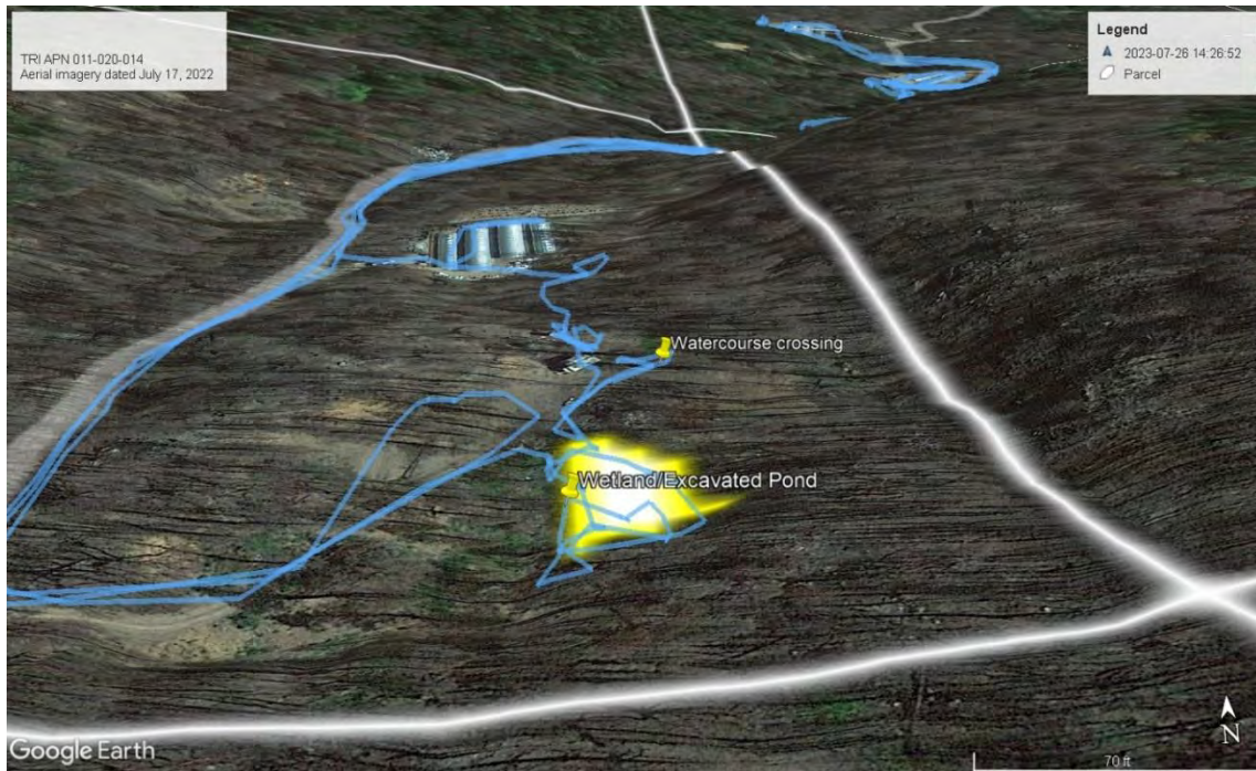
Figure 11. July 17, 2022 aerial imagery of southeast corner of the Property, with inspection track, with approximate area of wetland indicators, excavated pond, and watercourse crossing identified.
