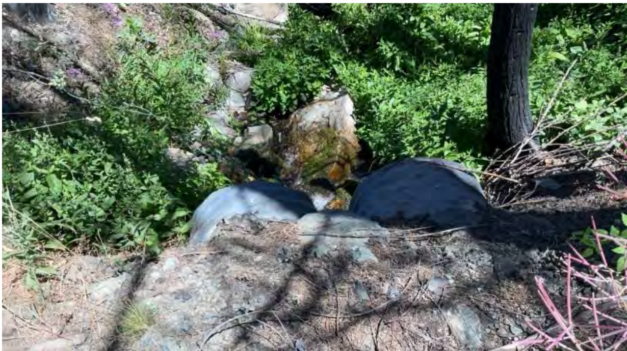
Figure 29. Point Feature 14 – Watercourse crossing comprised of two 24” culverts.
