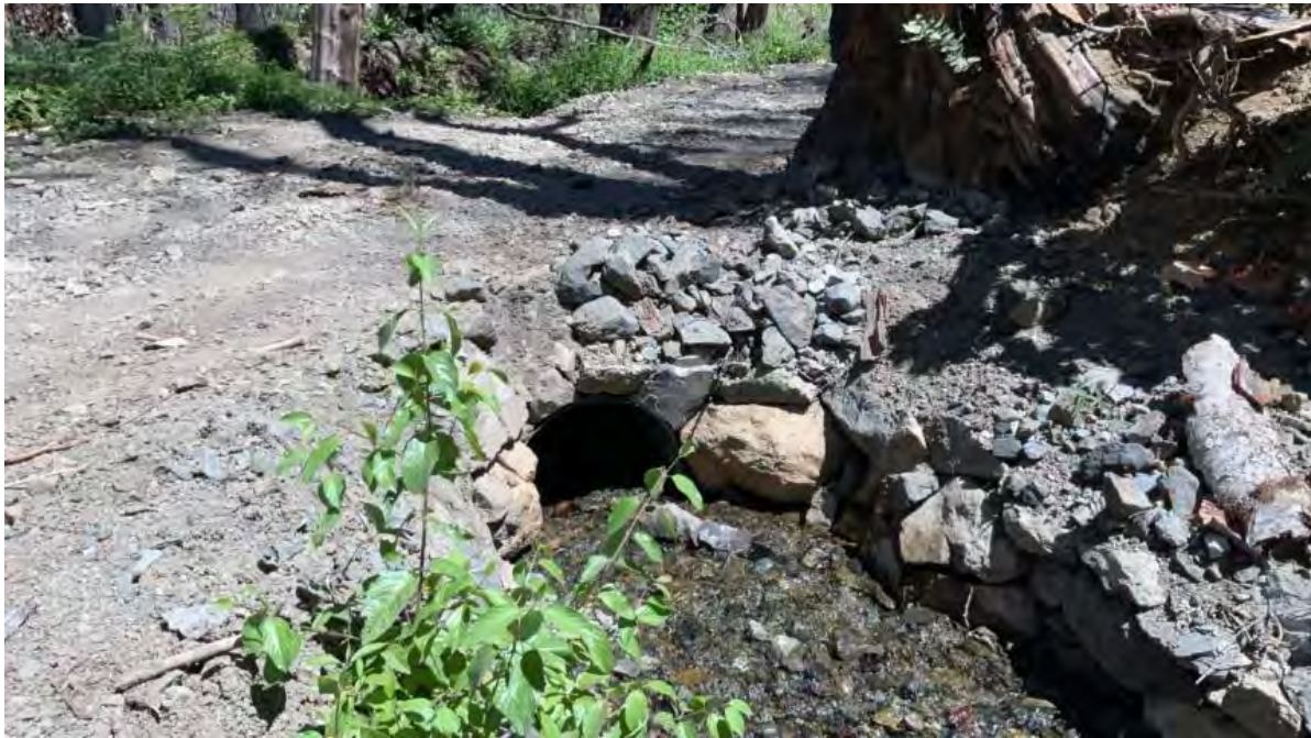
Figure 32. Point Feature 16 – inlet to watercourse crossing comprised of a half-filled 36” CMP.
