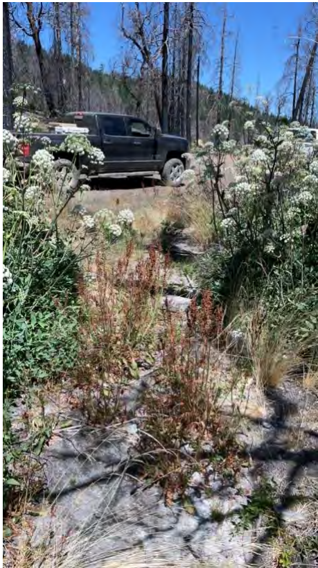
Figure 19. Line Feature 9 – outlet of pond to road ditch.
