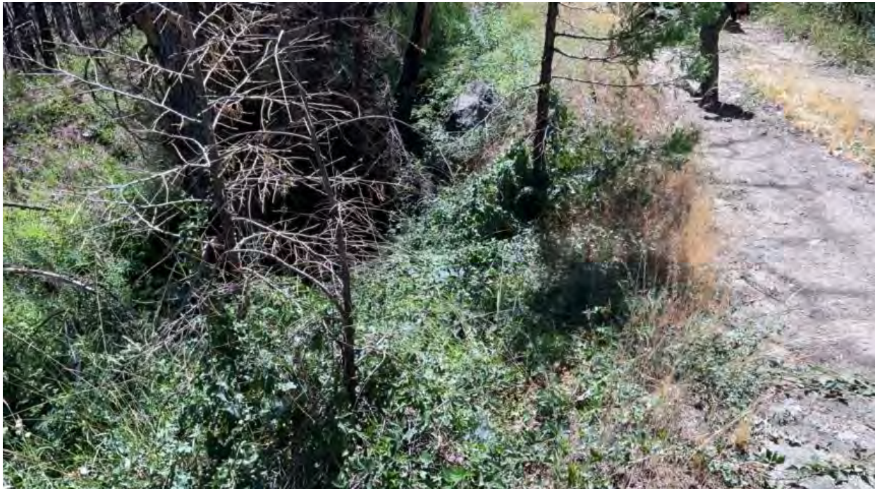
Figure 7. Point Feature 2 - Road surface next to Class II watercourse at crossing.
