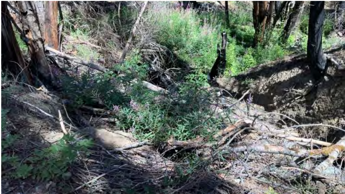
Figure 6. Point Feature 1 - Watercourse downstream of outlet of culvert.
