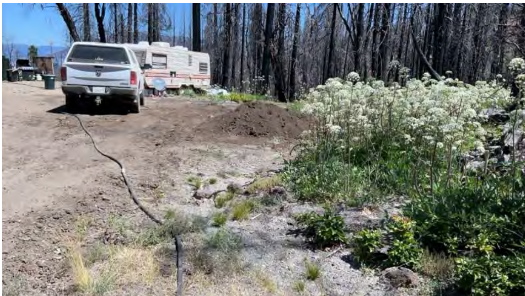
Figure 20. Line Feature 9 - Ditch from pond outlet.
