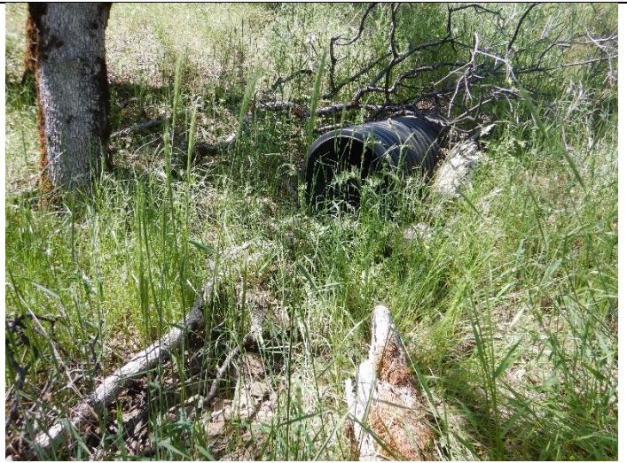
Photo 16: Outlet of a culverted watercourse crossing at WQ11
