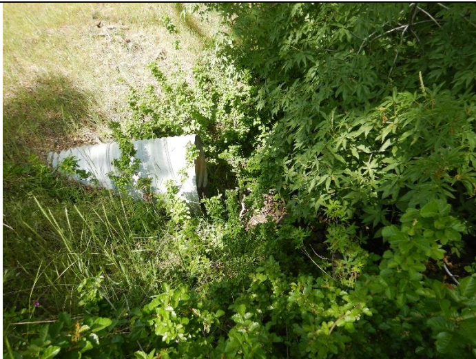
Photo 23: Outlet of a culverted watercourse crossing at WQ14
