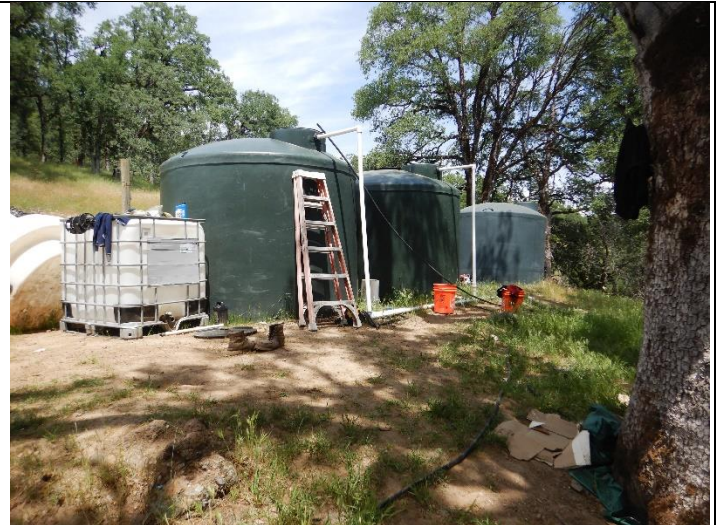
Photo 2: Water storage tanks at WQ3
