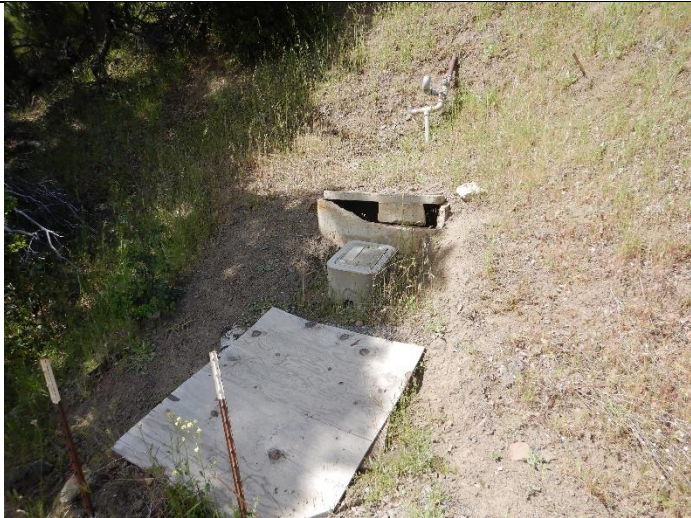
Photo 21: Water diversion structure at WQ13
