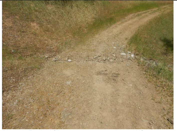
Photo 8: Rocked fill watercourse crossing at WQ5
