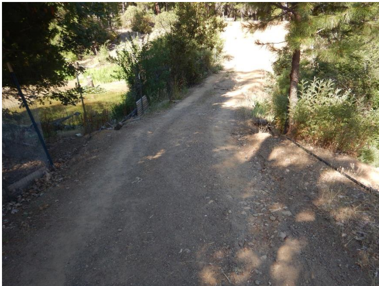
Photo 3 Bare dirt road leading to onstream pond.
