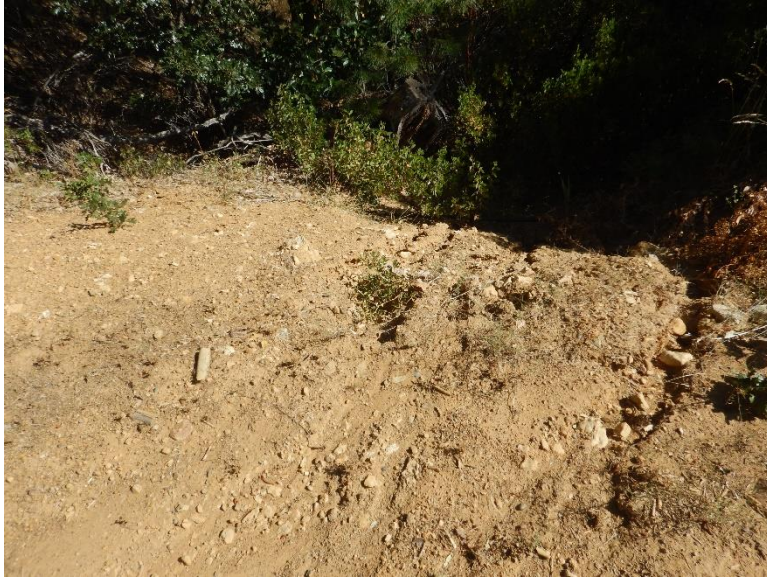
Photo 4 Loose fill from road discharging to stream below.
