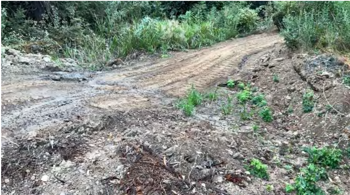
Figure 33. Point 17. Road crossing of wetland area.
