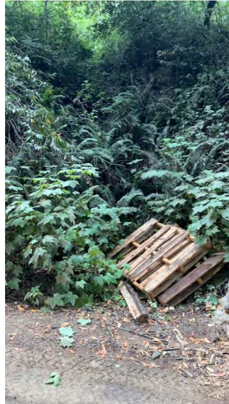
Figure 27. Point 13. Road crossing of small Class III with no conveyance structure.
