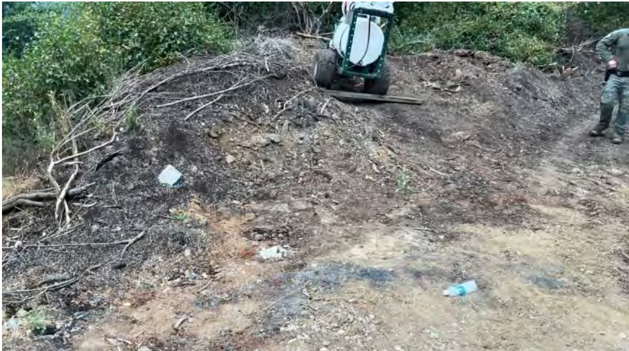
Figure 31. Point 14. Potting soil and spoils at top of steep road segment.
