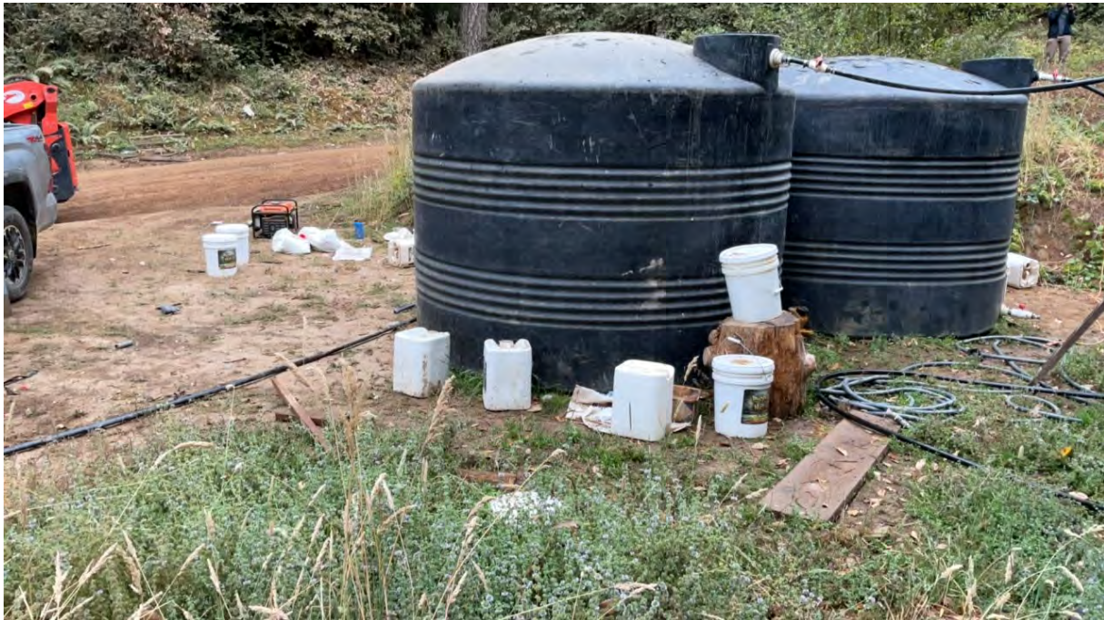
Figure 6. Point 2. Water tanks with fill line from well. Fertilizer and generators on ground.
