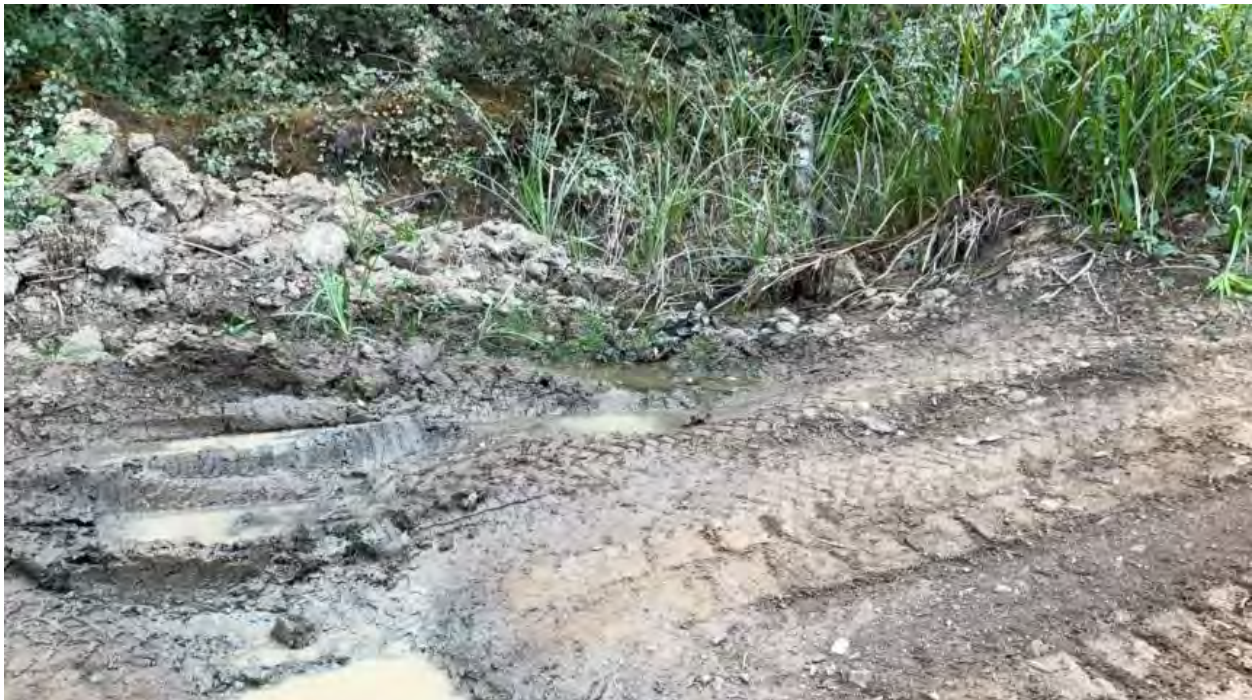
Figure 34. Point 17. Road crossing of wetland area.
