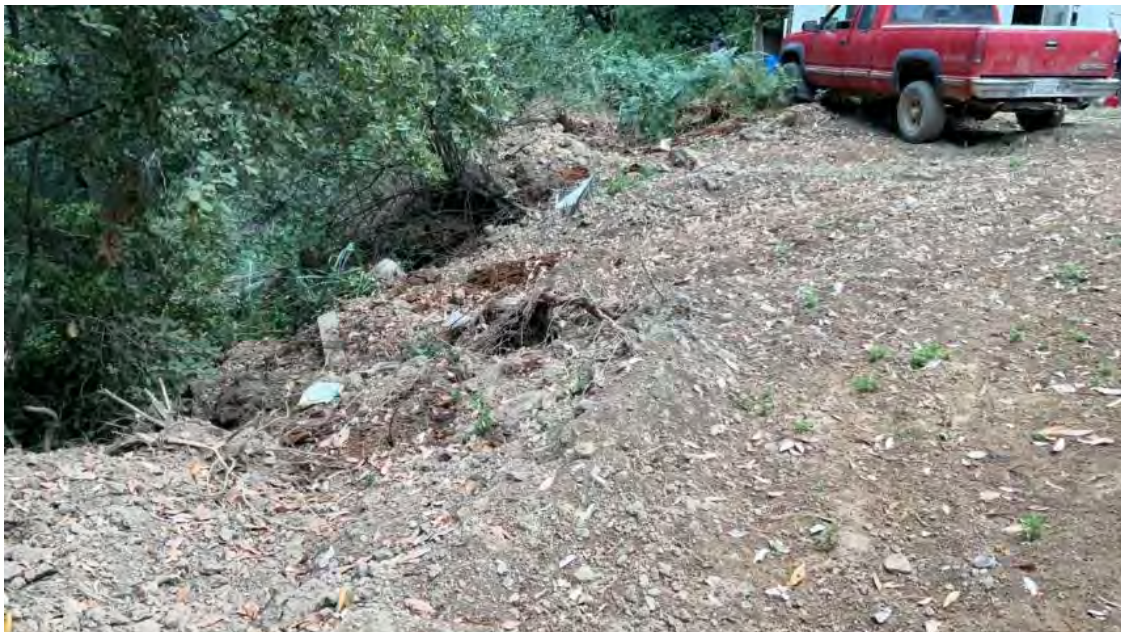
Figure 10. Point 4. Recent side-cast over steep slope from recent road work.
