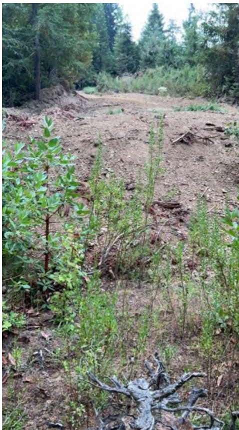
Figure 38. Point 19. Side cast spoils.
