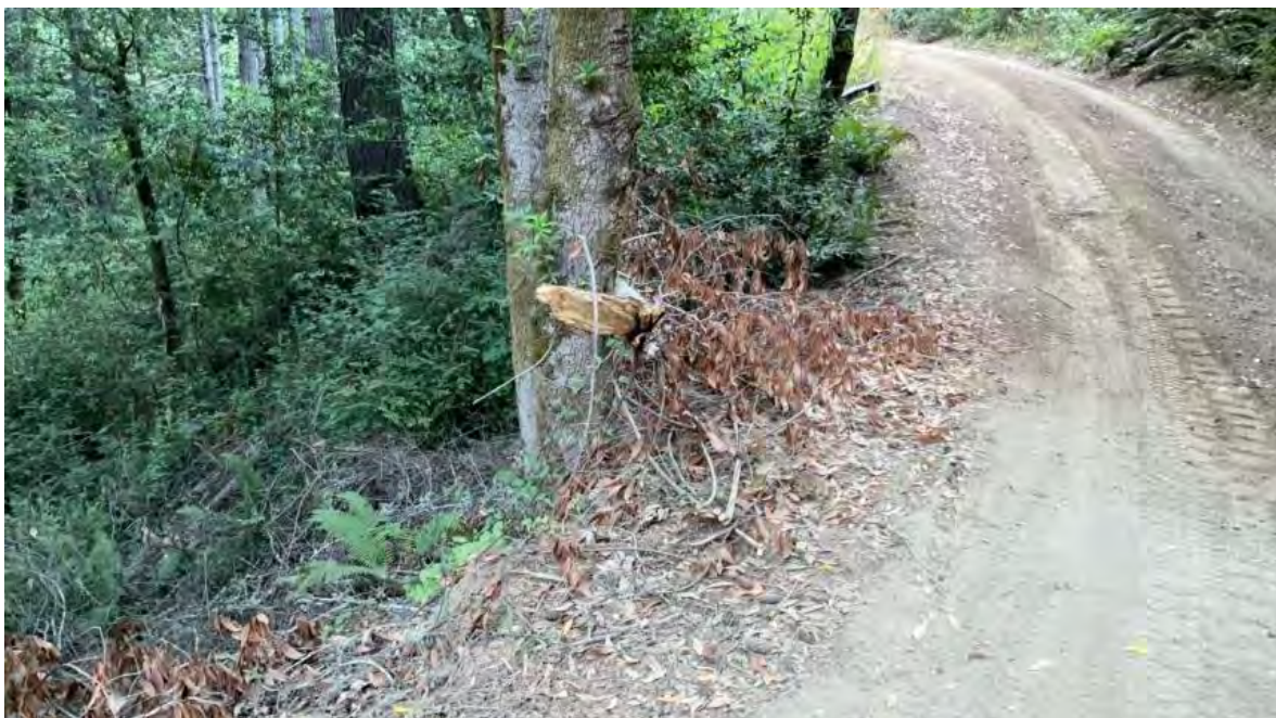
Figure 28. Point 13. Outboard edge of roadway at watercourse.
