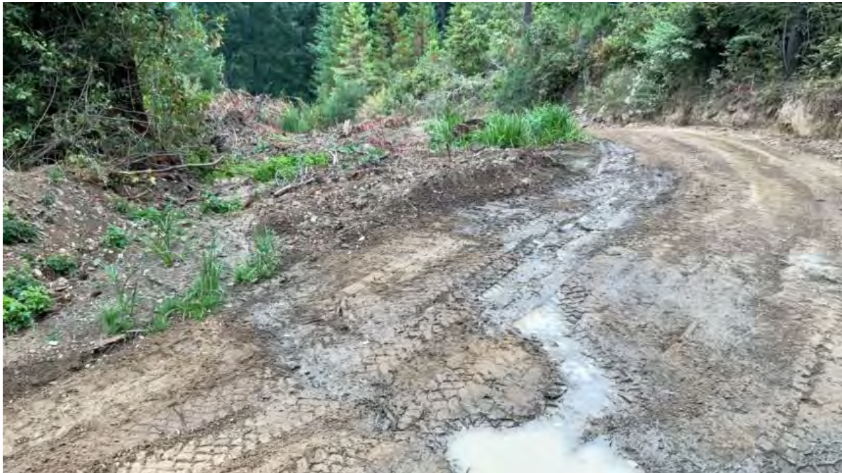
Figure 35. Point 17. Road crossing of wetland area.
