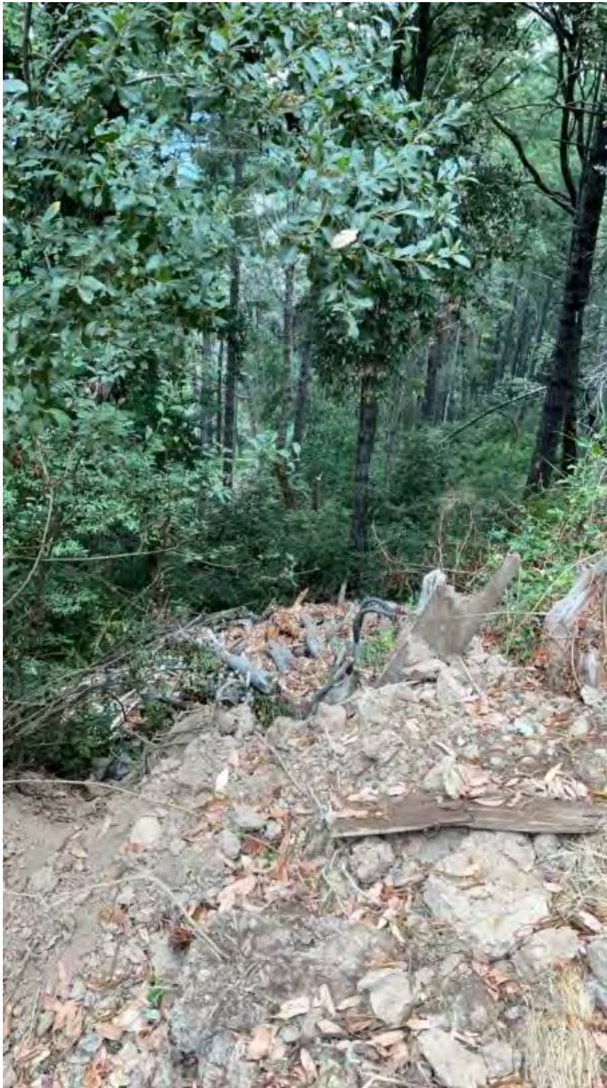
Figure 11. Point 4. Side cast over steep slope.
