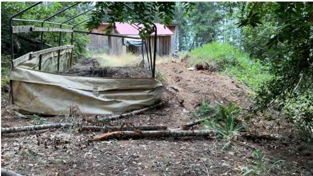
Figure 13. Point 5. Recent ground/soil disturbance.
