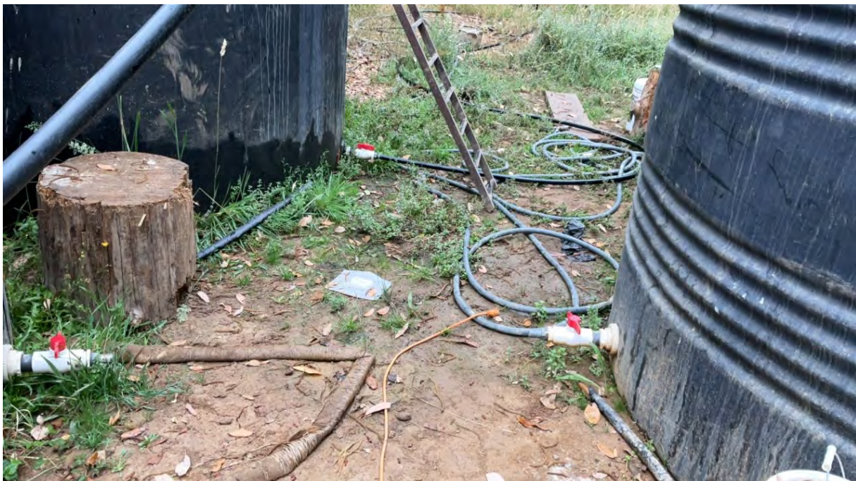
Figure 7. Point 2. Wet ground indicating overflowing.
