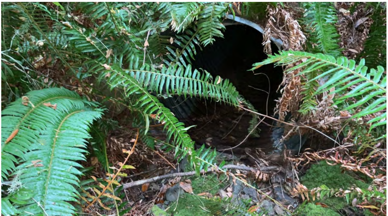
Figure 41. Point 21. Culvert inlet.
