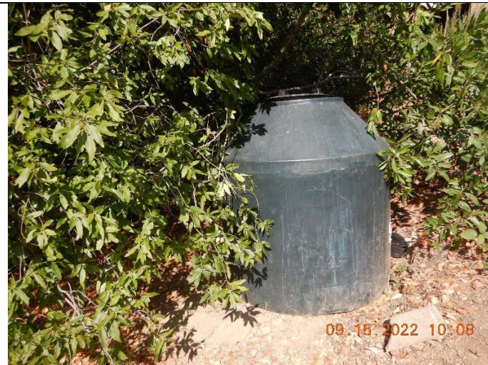
Photo 3: Water storage tank at inspection point WQ2
