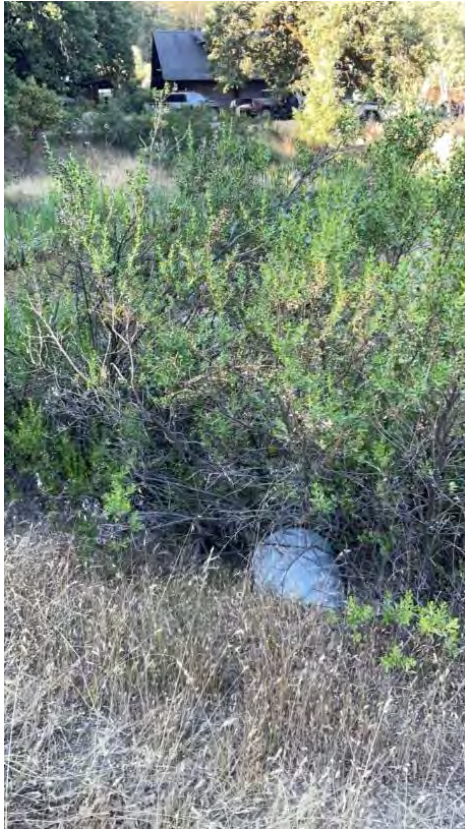
Figure 7. Polygon 1. Outlet pipe from pond is an 18" corrugated metal pipe (CMP).
