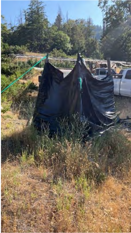
Figure 14. Pit privy with domestic waste discharge to ground is at Point Location 8.
