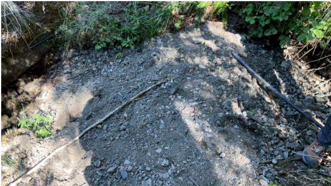
Figure 19. The berm at Point Location 10 is approximately eight feet wide, five feet long, and one foot deep.
