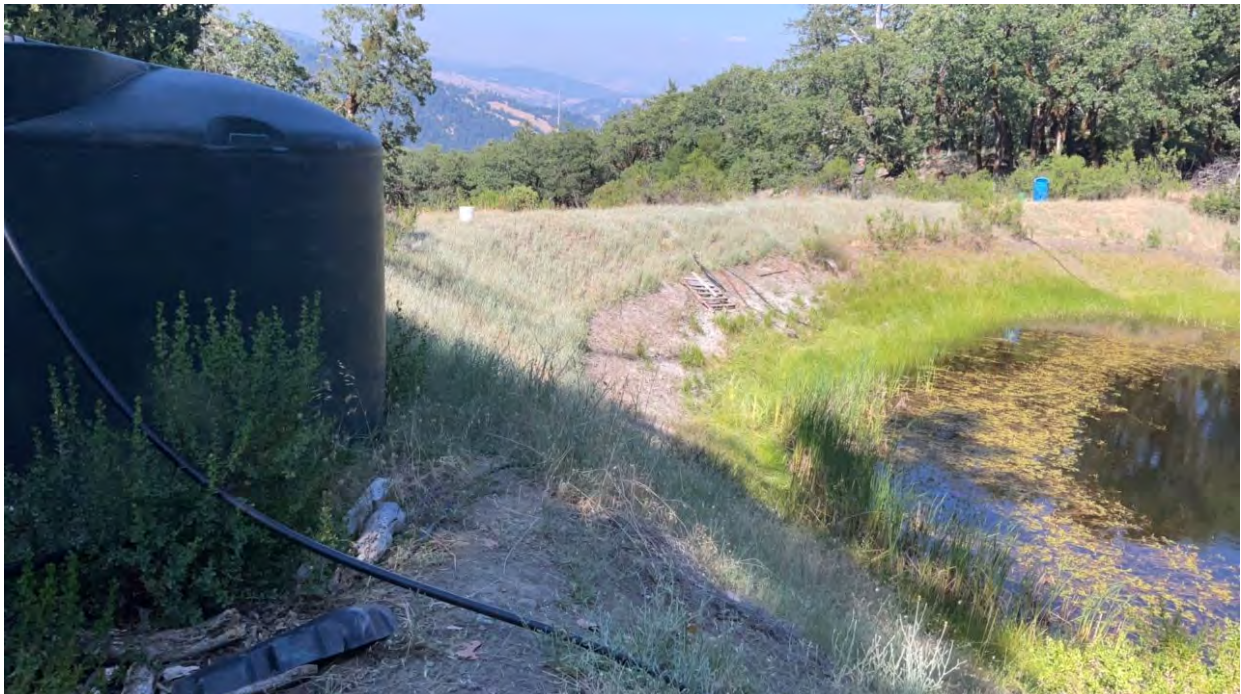
Figure 6. Earthen berm and water tank on the pond at Polygon Location 1.
