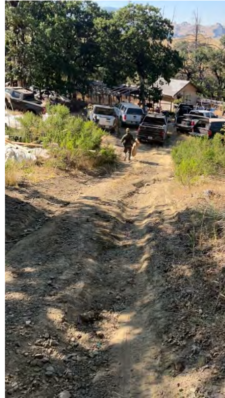
Figure 8. Road rills down the steep access driveway, aligned with Point Location 3, indicated concentrated stormwater runoff, erosion, and sediment transport downslope. The road lacked adequate drainage or surfacing.
