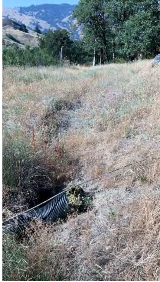
Figure 13. Looking downslope from Line Feature 7 along the flowpath that can carry concentrated stormwater, sediment and other contaminants downslope.
