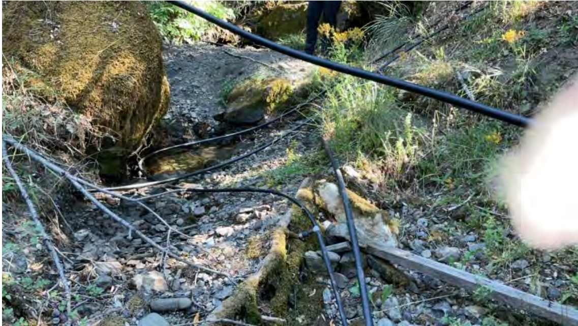
Figure 18. The berm at Point Location 10 is constructed across a narrow portion of the channel to impede one hundred percent of the surface stream flow and is comprised of gravel substrate that appears to be dug from the channel with a shovel. Surface flow is disconnected downstream of the berm.
