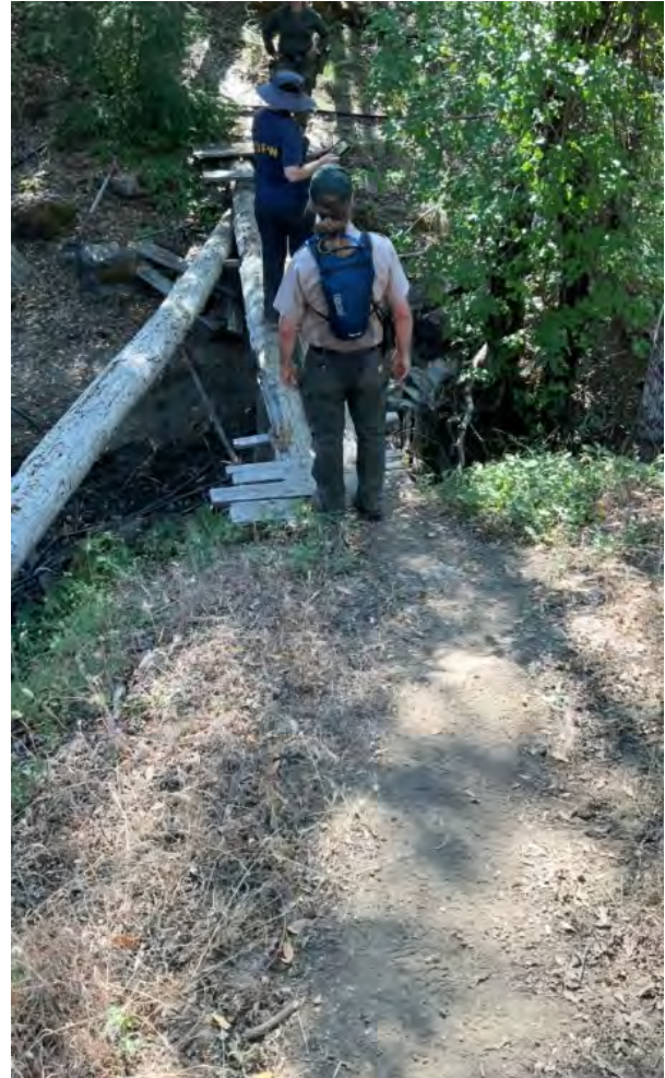
Figure 15. Watercourse crossing at Point Location 9 is a footbridge constructed with poles driven into the bed of a blue line stream. The piles impede free flow and woody material transport downstream.
