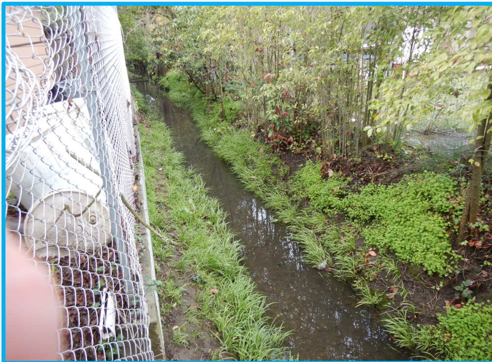
Photograph 7: Poppy Creek looking downstream showing vegetation and bamboo. Appeared high-water flooded the opposite bank backyard.
