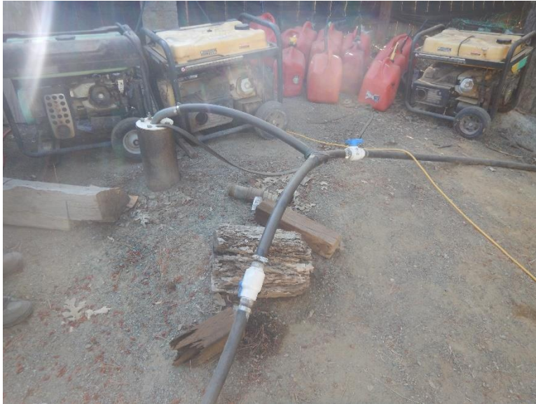
Photo 1: Well, generators, and gas cans without secondary containment.
