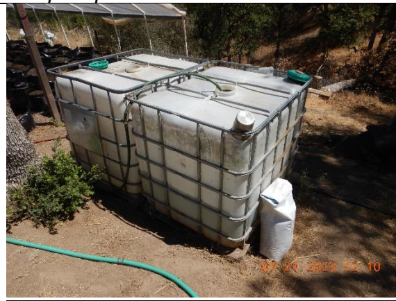
Photo 6 – Water storage tanks at WQ6
