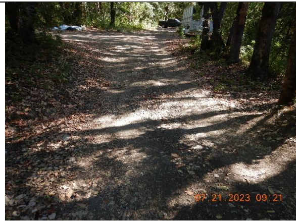
Photo 6 - partially rockered, fill watercourse
