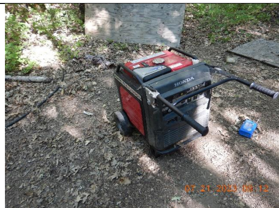
Photo 12 – A generator at WQ5
