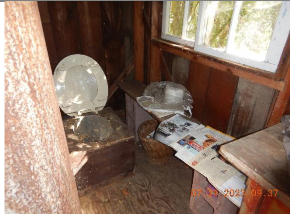
Photo 20 – outhouse toilet at WQ10
