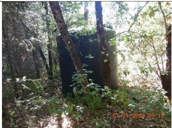
Photo10 – A water storage tank at WQ7
