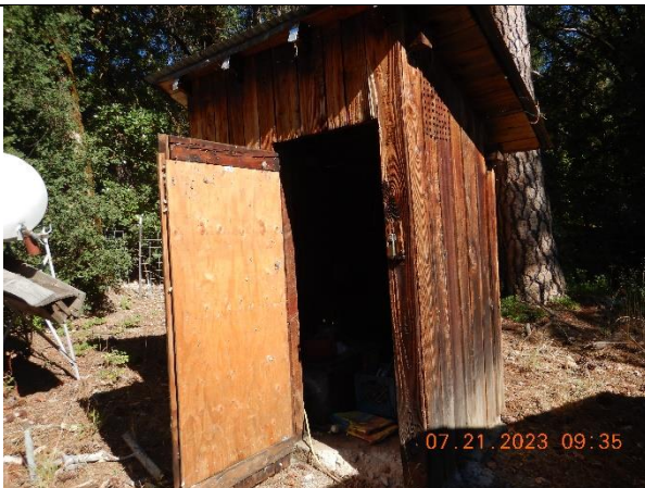
Photo 9 – What appears to be a groundwater well house at WQ11
