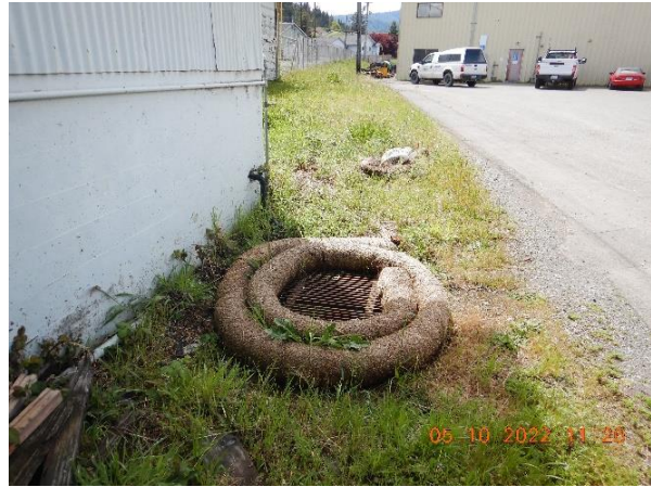
Pictures 12a, 12b: Looking southeast at storm drain inlets on north side of the facility in drainage area 3. Some of the fiber rolls installed around the inlets are old and in need of maintenance. Picture taken by Farzad Kasmaei.
