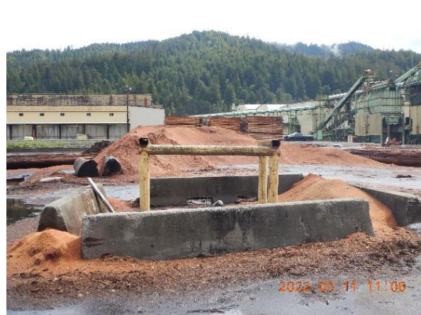
Pictures 1f and 1g: Storm drain inlets within drainage area 1 observed with no inlet protection BMPs and surrounded by wood waste material. Picture taken by Heaven Moore.
