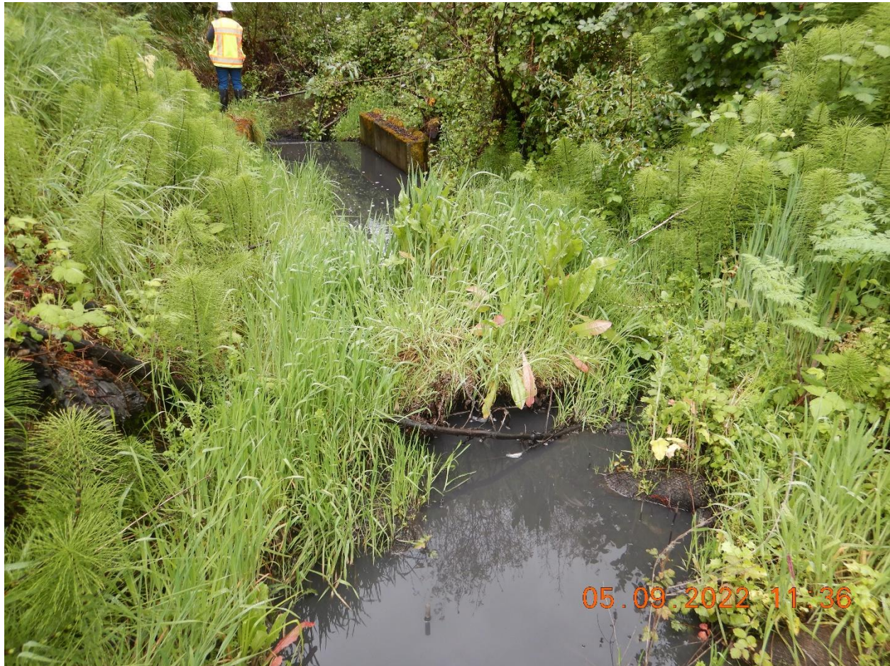
Picture 6f: Looking northwest at discharge point (outfall) from the main retention pond. The discharge water from the retention pond drains directly into Eel River which is just beyond the view of the picture. Picture taken by Farzad Kasmaei.
