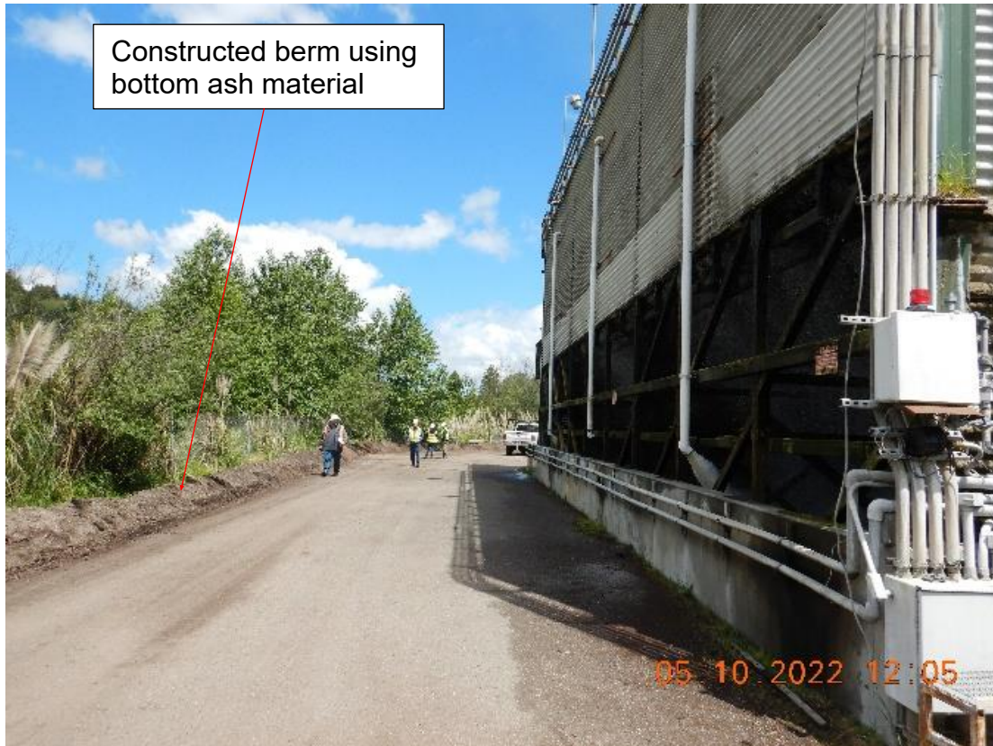
Picture 18a: Looking north at cooling tower and a constructed berm using the bottom ash materials along the west side of the Cogen along the edge of the Log Pond. Picture taken by Farzad Kasmaei.
