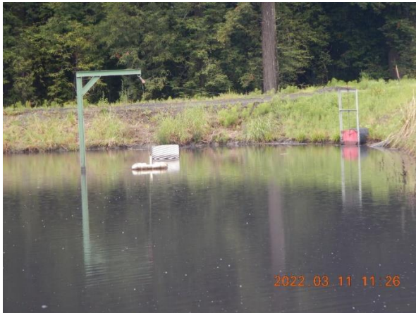
Pictures 6a and 6b: Picture of the outlet structures within retention pond to the Eel River. The outlet structure controlled by the pulley suspended by the green cantilever structure was open and discharging. The overflow with the red gate valve was closed at the time of inspection. The vertical corrugated metal riser pipe is a passive high flow bypass. Picture 6a taken by Heaven Moore. Picture 6b taken by Farzad Kasmaei.
