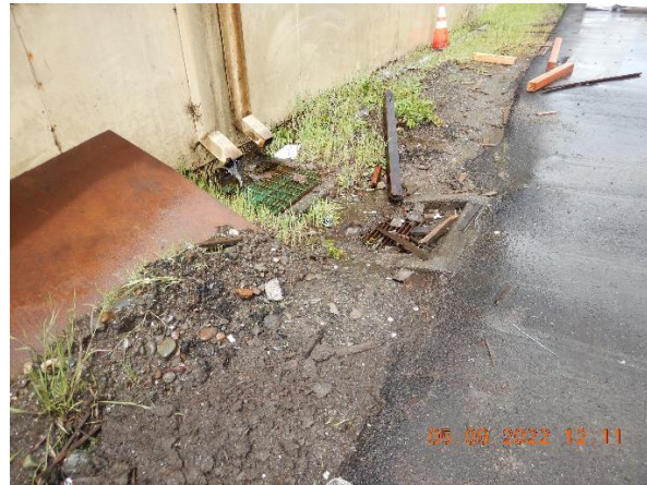
Pictures 8a, 8b: Unprotected inlet that receives runoff from the down spouts of the sawmill building and paved area within the drainage area 1. Picture taken by Farzad Kasmaei.
