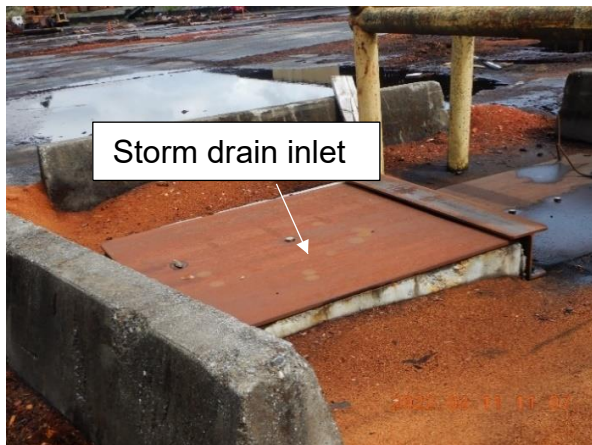
Pictures 1f and 1g: Storm drain inlets within drainage area 1 observed with no inlet protection BMPs and surrounded by wood waste material. Picture taken by Heaven Moore.
