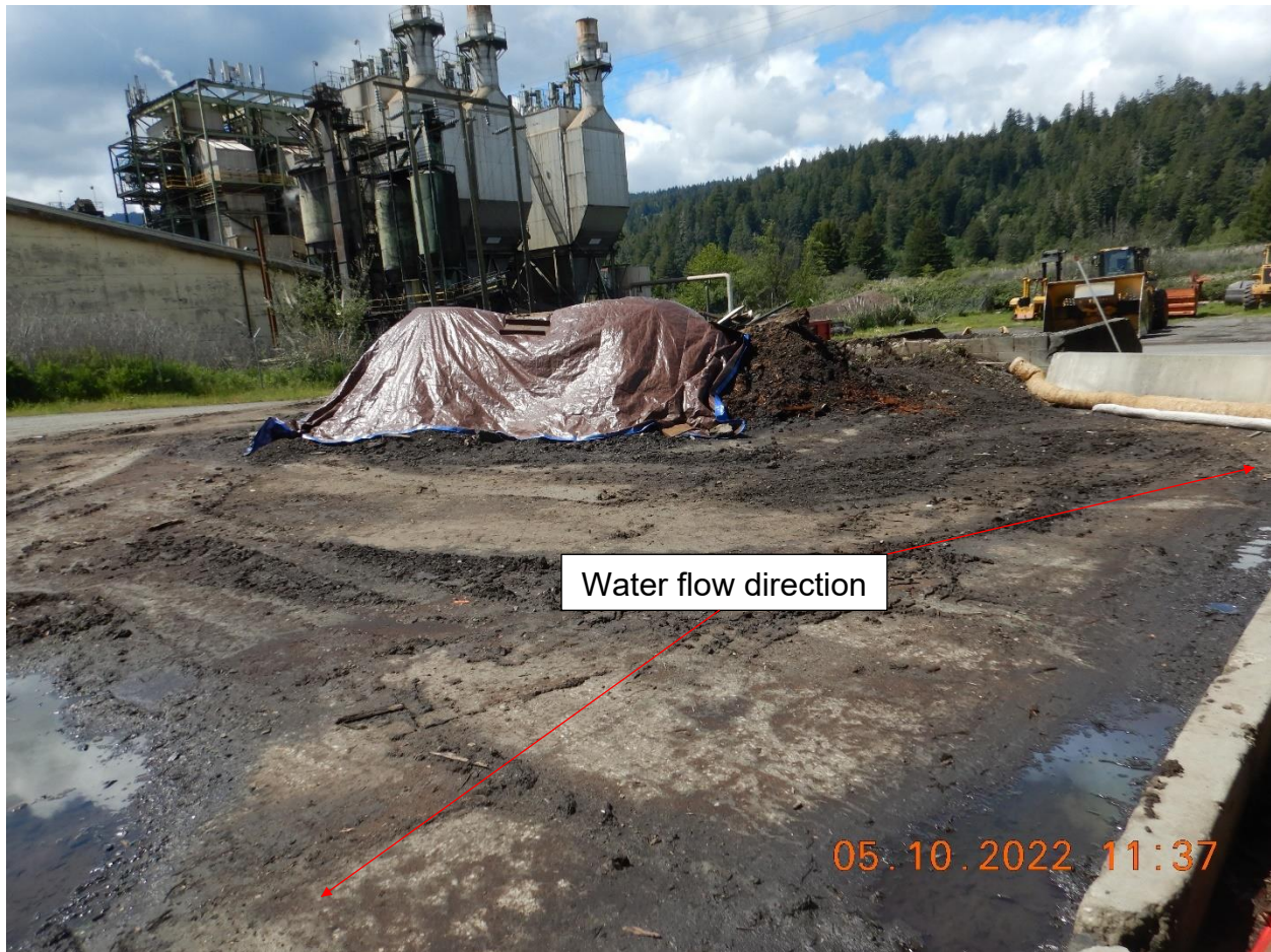
Picture 14b: Partially covered stockpile of the material that is washed from the equipment and vehicles is then stockpiled and removed as hazardous material every three to six months. Material is also present on the pavement. Water flow directions are shown with red arrows on the photo. Picture taken by Farzad Kasmaei.
