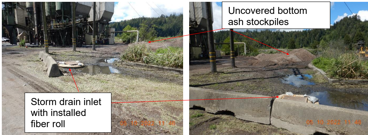
Pictures 16a, 16b: View of uncovered bottom ash stockpiles on the north side of the Cogen area and the storm drain inlet that receives runoff from this area. Picture taken by Farzad Kasmaei.
