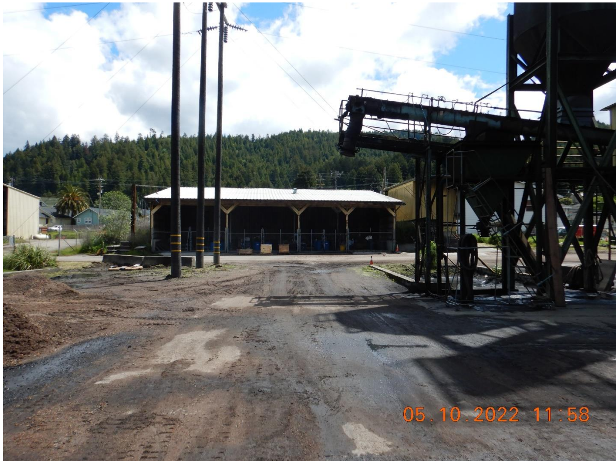
Picture 17c: Looking east at equipment shed within the paved cogeneration area. Observed sawdust and tracking on the ground, oil and hydrocarbon can be seen on the ground throughout this area and under the equipment. The area had a strong smell of hydrocarbons. The bottom ash stockpiles to the left of the image are unprotected and would also discharge into the Log Pond. The ponded stormwater from photo 17a can be seen behind the equipment on the right side of the picture and the storm drain inlet from photo 17b above is just beyond the date stamp to the right of this picture. Picture taken by Farzad Kasmaei
