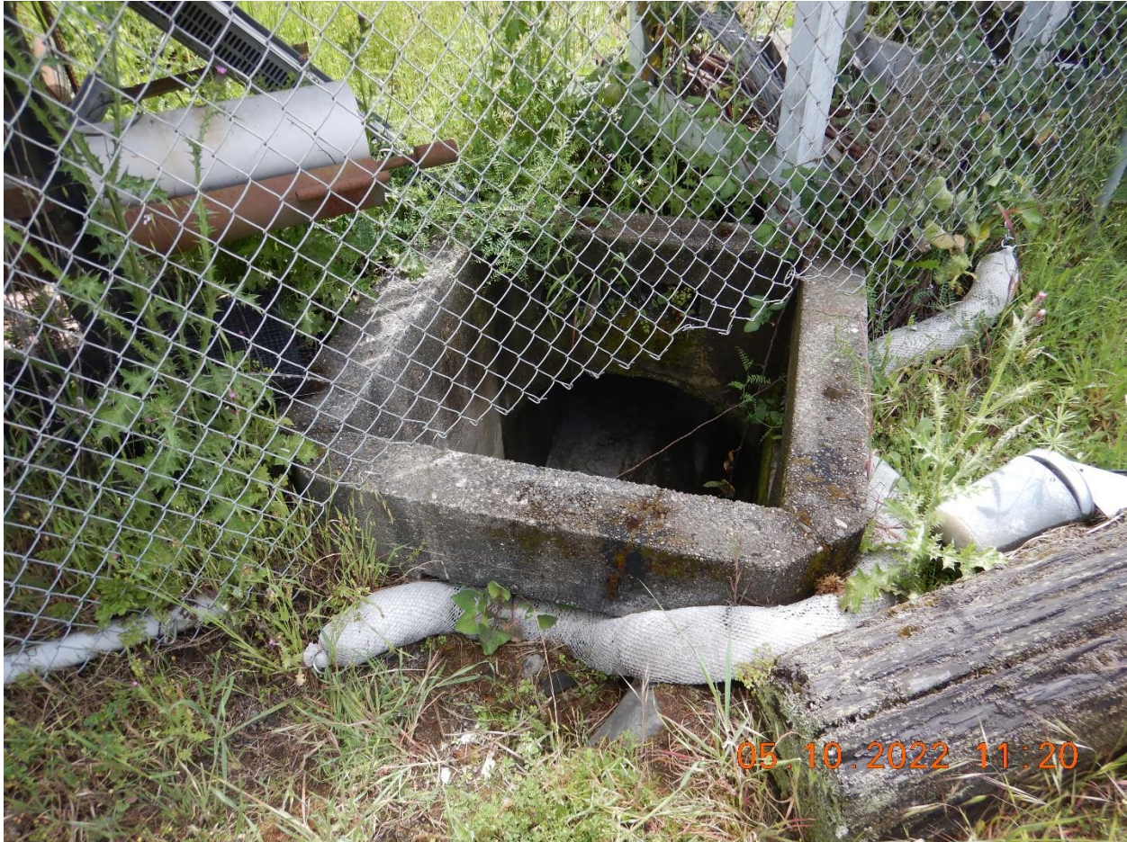
Picture 11: Looking east at catch basin 003 where the samples are collected. This catch basin receives facility's runoff from northern areas of the facility as well as highway runoff. The catch basin open spaces have been covered with Filtrexx. Picture taken by Farzad Kasmaei.
