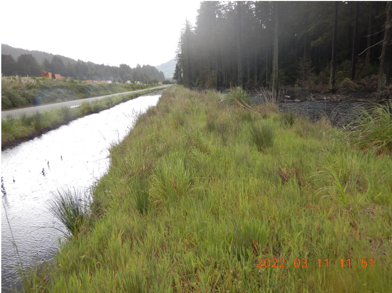
Picture 7c: Water that has been pumped from the retention pond with a portable pump and discharged into the tree plantation area, shown on the right of the picture, and the swale on the left of the picture. Picture taken by Heaven Moore.
