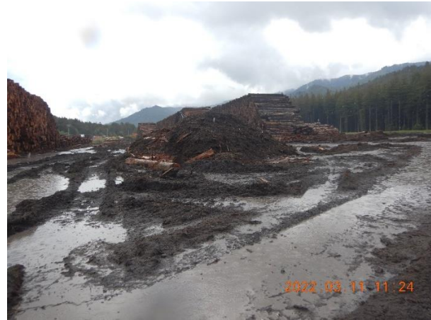
Pictures 2h and 2i: Large industrial waste material piles and stockpiles located within the log deck area of drainage area 1 exposed to rain. This paved area is covered with many inches debris, mud, wood fiber. No BMPs are present. Picture taken by Heaven Moore.
