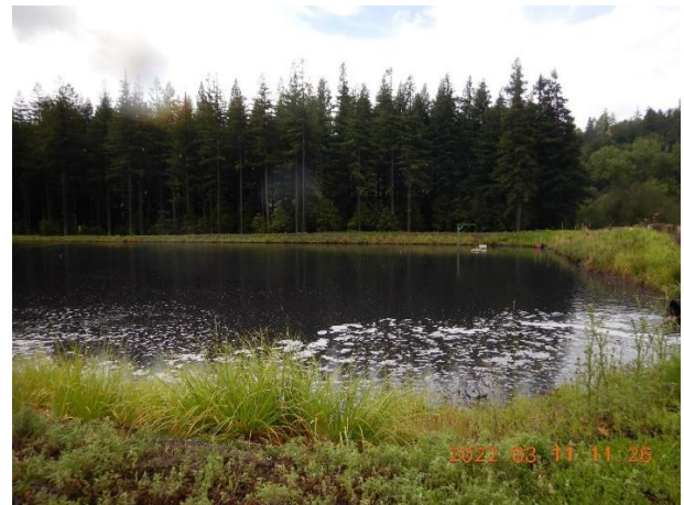
Pictures 5a and 5b: Picture of the retention pond that receives the majority of the runoff from Drainage areas 1 and 7 as well as Drainage area 5 on the north side of highway 101 prior to discharge to the Eel River. Picture taken by Heaven Moore.
