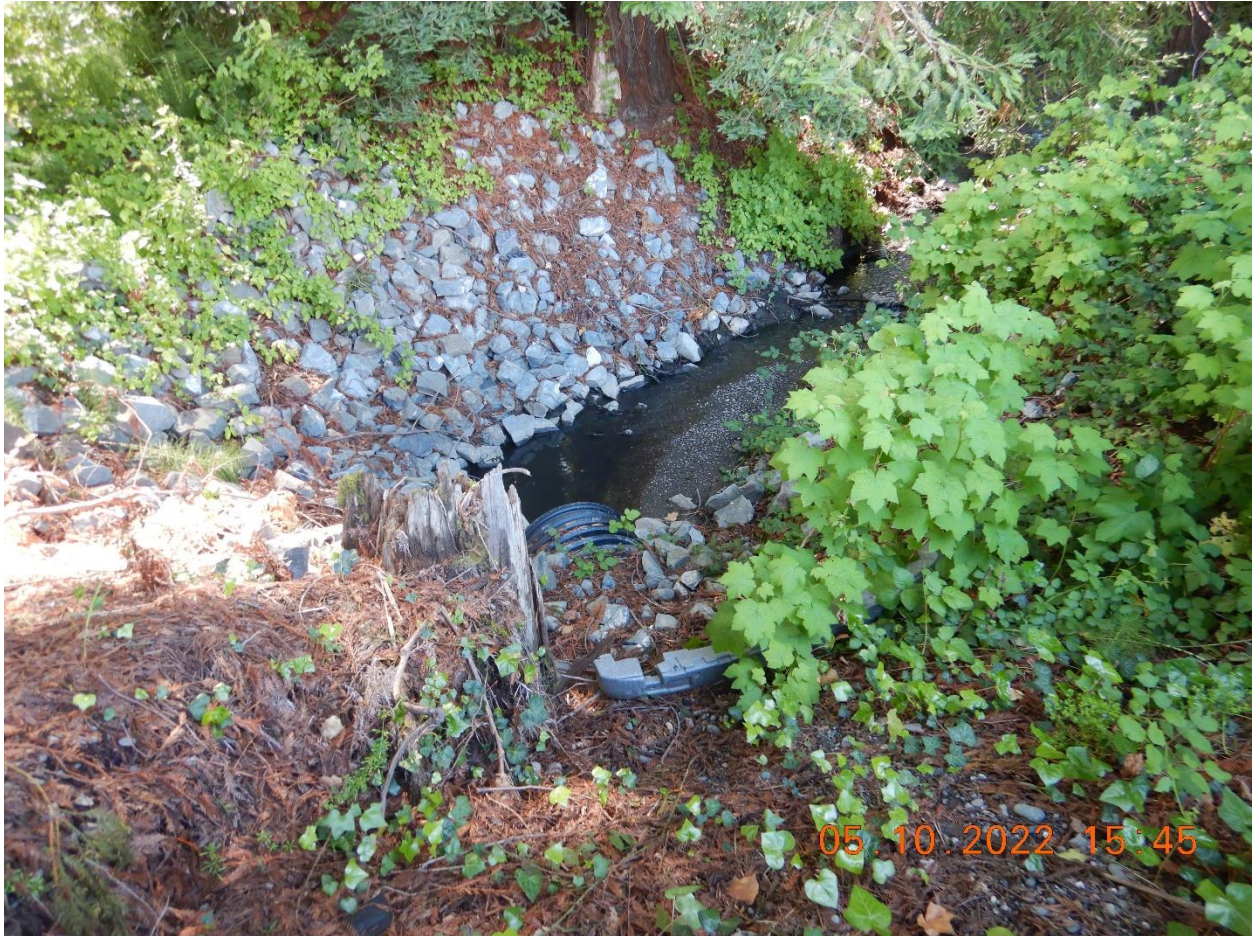
Picture 22. View of an off-site discharge point where the samples are collected (002). The facility's runoff that are captured by storm drain inlets within the Drainage Area 2 drains to Eel River via this outfall. Picture taken by Farzad Kasmaei.
