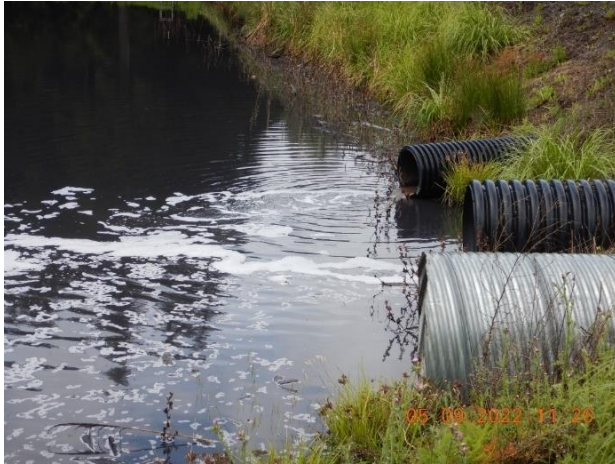
Pictures 5c and 5d: View of stormwater pipes discharging the runoff into the north corner of the main retention pond. These pipes mostly receive runoff from the diversion valve 001 and the DIs within drainage areas 1 and 7 as well as Drainage area 5 on the north side of highway 101. The water appeared to be highly turbid, dark, and had gray hue. Foam was observed on the surface. Picture 5c taken by Farzad Kasmaei. Picture 5d taken by Heaven Moore.
