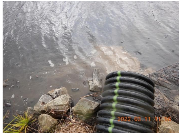
Pictures 5c and 5d: View of stormwater pipes discharging the runoff into the north corner of the main retention pond. These pipes mostly receive runoff from the diversion valve 001 and the DIs within drainage areas 1 and 7 as well as Drainage area 5 on the north side of highway 101. The water appeared to be highly turbid, dark, and had gray hue. Foam was observed on the surface. Picture 5c taken by Farzad Kasmaei. Picture 5d taken by Heaven Moore.
