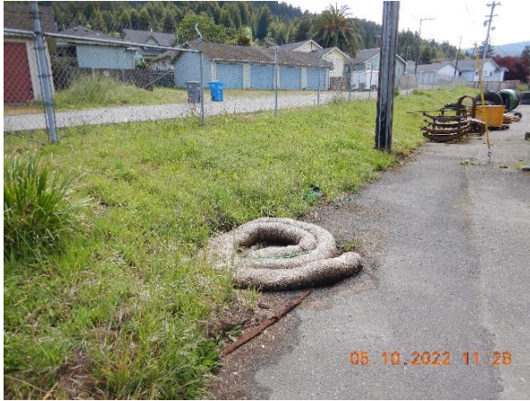
Pictures 12a, 12b: Looking southeast at storm drain inlets on north side of the facility in drainage area 3. Some of the fiber rolls installed around the inlets are old and in need of maintenance. Picture taken by Farzad Kasmaei.
