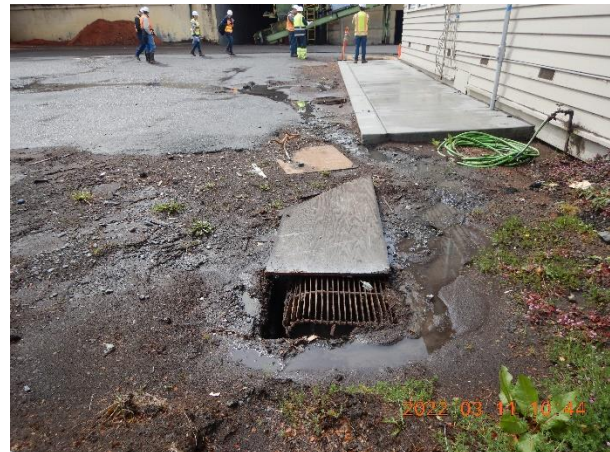
Pictures 1a, 1b: Storm drain inlets within drainage area 1 observed receiving very muddy discharge, many with observable oil sheen and had no inlet protection BMPs. Picture taken by Heaven Moore.
