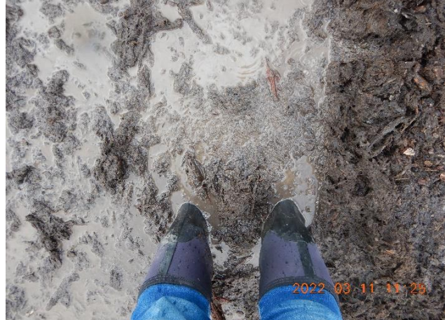
Pictures 4c and 4d: Closeup photos showing the depth of the mud, wood fiber, bark, and ponded stormwater on top of the paved log deck. The main retention pond receives runoff from this area. Picture taken by Heaven Moore.
