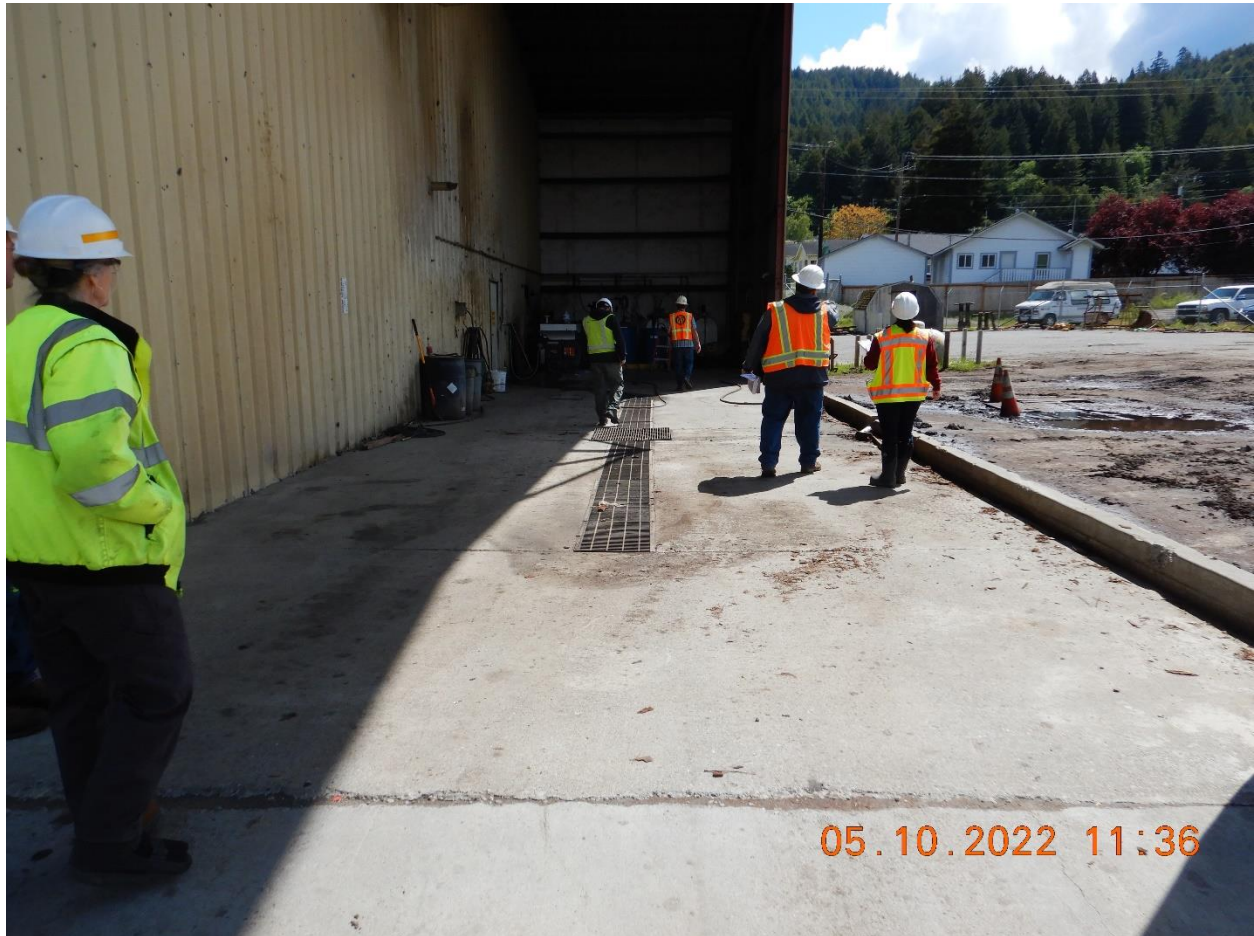
Picture 13c: View of covered vehicle wash area. Facility staff stated that drain within this area discharges to sewer. Picture taken by Farzad Kasmaei.
