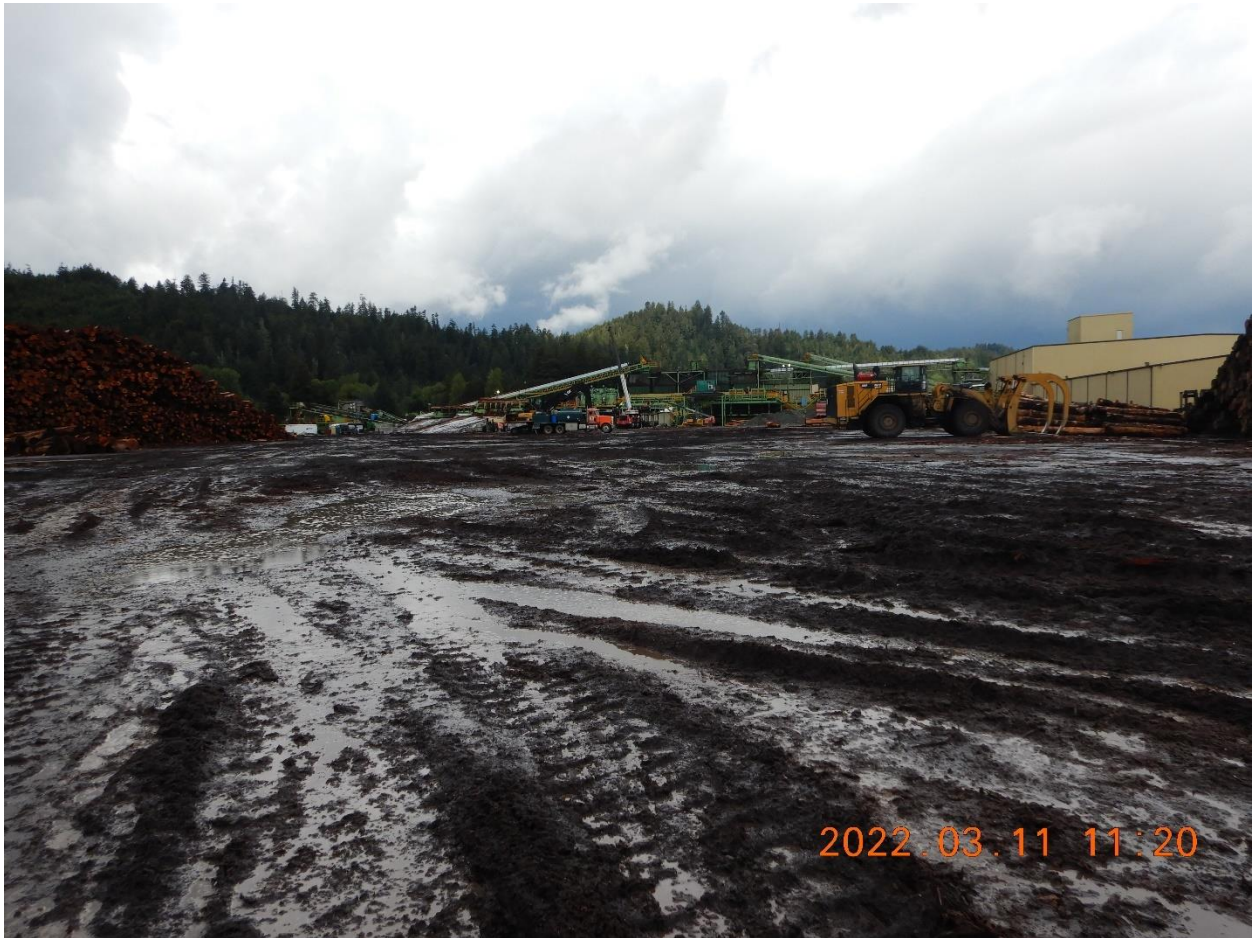
Picture 2c: Industrial equipment, materials, and waste located within the log deck area in drainage area 1 exposed to rain. This paved area is covered with many inches debris, mud, wood fiber. No housekeeping BMPs or inlet protection BMPs are present. Picture taken by Heaven Moore.
