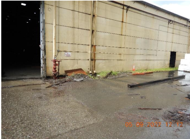
Pictures 8a, 8b: Unprotected inlet that receives runoff from the down spouts of the sawmill building and paved area within the drainage area 1. Picture taken by Farzad Kasmaei.
