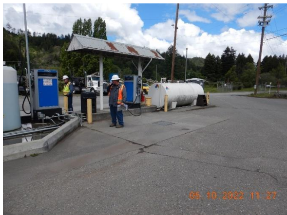
Pictures 10a and 10b: Onsite fueling station. Facility staff were unsure if the adjacent inlets were storm drain or sewer. Secondary containment not provided on all tanks/fuel. Accumulated water in concrete containment area diminished by accumulated stormwater. Picture taken by Farzad Kasmaei.
