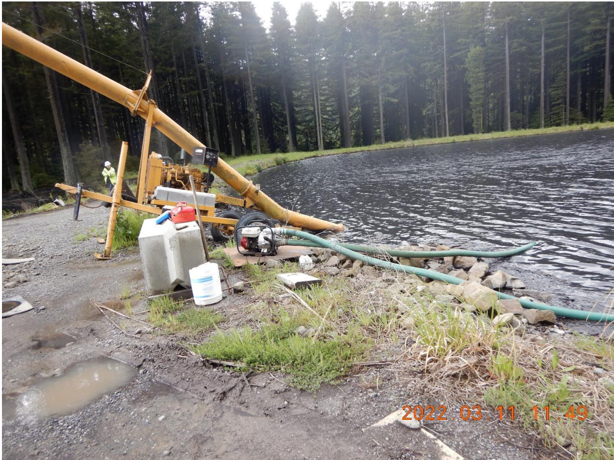
Picture 7a: Water being pumped from the retention pond with a portable pump and being discharged into the tree plantation area. Picture taken by Heaven Moore.
