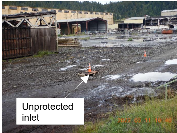
Pictures 1a, 1b: Storm drain inlets within drainage area 1 observed receiving very muddy discharge, many with observable oil sheen and had no inlet protection BMPs. Picture taken by Heaven Moore.
