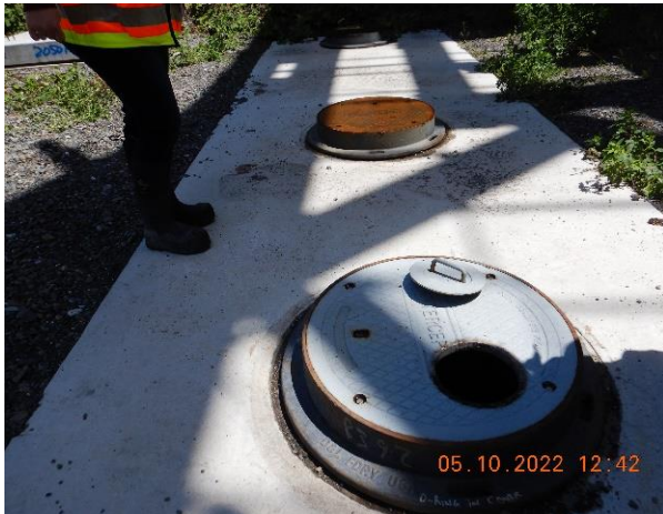
Pictures 21b, 21c: Newly installed clarifier on the south side of the Machine Shop building where the samples are collected (SWDB 3B). Picture taken by Farzad Kasmaei.
