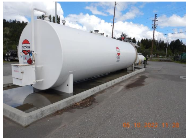
Pictures 10a and 10b: Onsite fueling station. Facility staff were unsure if the adjacent inlets were storm drain or sewer. Secondary containment not provided on all tanks/fuel. Accumulated water in concrete containment area diminished by accumulated stormwater. Picture taken by Farzad Kasmaei.
