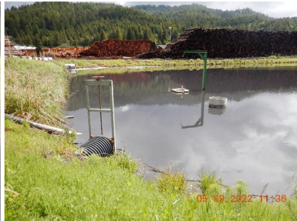
Pictures 6a and 6b: Picture of the outlet structures within retention pond to the Eel River. The outlet structure controlled by the pulley suspended by the green cantilever structure was open and discharging. The overflow with the red gate valve was closed at the time of inspection. The vertical corrugated metal riser pipe is a passive high flow bypass. Picture 6a taken by Heaven Moore. Picture 6b taken by Farzad Kasmaei.
