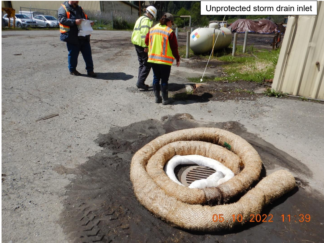
Picture 15: Storm drain inlets located behind the vehicle maintenance area, wash bay, and outdoor wash area. A fiber roll and Filtrex oil absorbing boom have been installed around the inlet in the foreground, but the inlet in the background is unprotected and propped open. Picture taken by Farzad Kasmaei.
