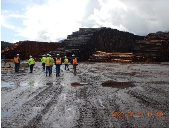
Pictures 3c and 3d: Large material stockpiles located within the log deck area of drainage area 1 exposed to rain. This paved area is covered with many inches debris, mud, wood fiber. No BMPs are present. Picture taken by Heaven Moore.
