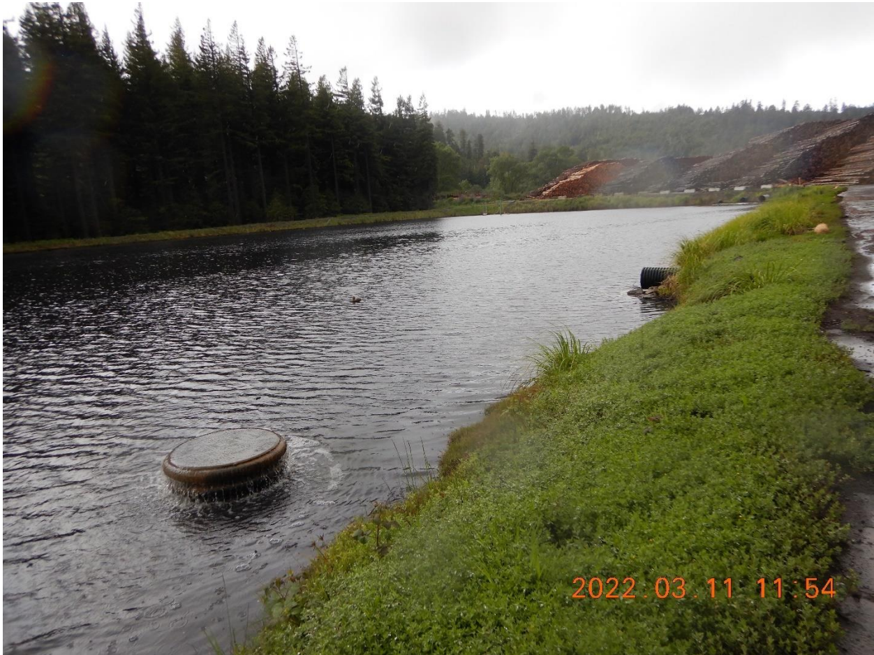
Picture : View of bubble-up stormwater pipe discharging runoff from Drainage area 5 on the north side of highway 101 into the retention pond. The water appeared to be highly turbid, dark, and had gray hue. Picture taken by Heaven Moore.
