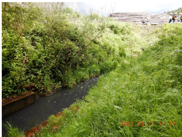
Pictures 6g and 6h: Picture discharge from the retention pond to the Eel River. The discharge appeared to be highly turbid, dark, and had a gray hue. Foam was observed on the surface. Pictures taken by Heaven Moore.
