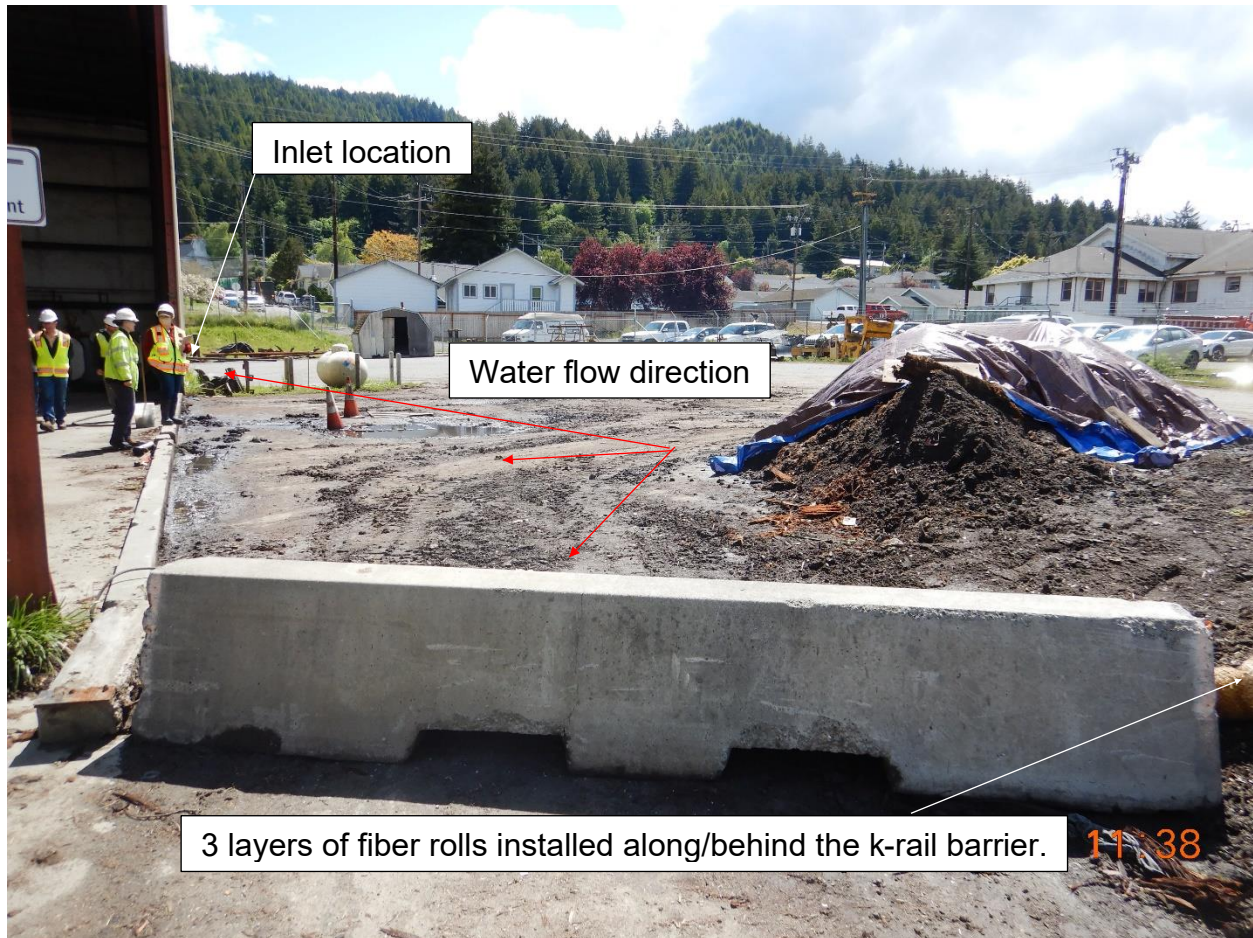
Picture 14a: View of area adjacent to vehicle wash bay area. Water flow directions are shown with red arrows on the photo. Note the storm drain inlet (Photo 15) behind the maintenance shed receives runoff from this area. Picture taken by Farzad Kasmaei.
