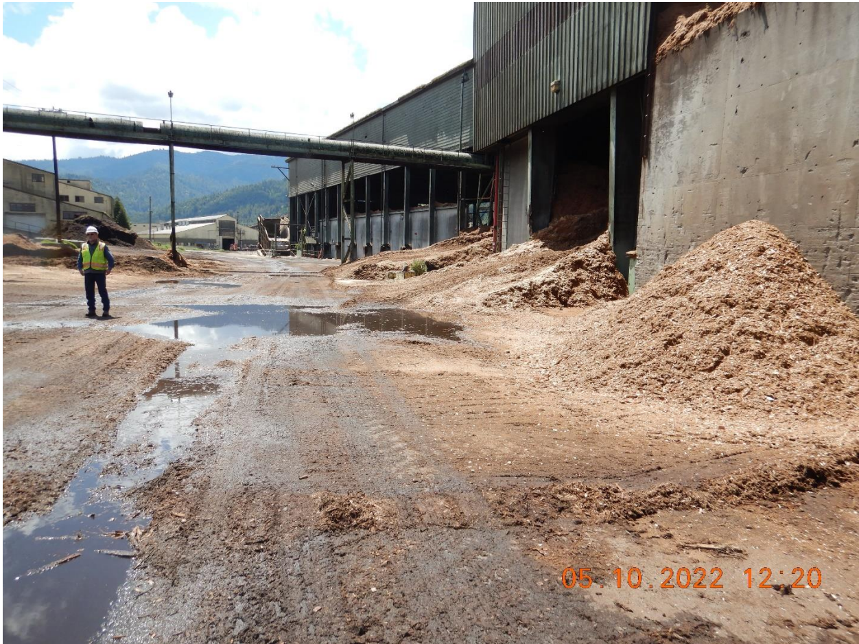
Picture 20a: Looking South at sawmill yard in Drainage Area 2. Wood chips and sawdust accumulations were observed outside throughout the yard as well as unprotected stockpiles. Picture taken by Farzad Kasmaei.
