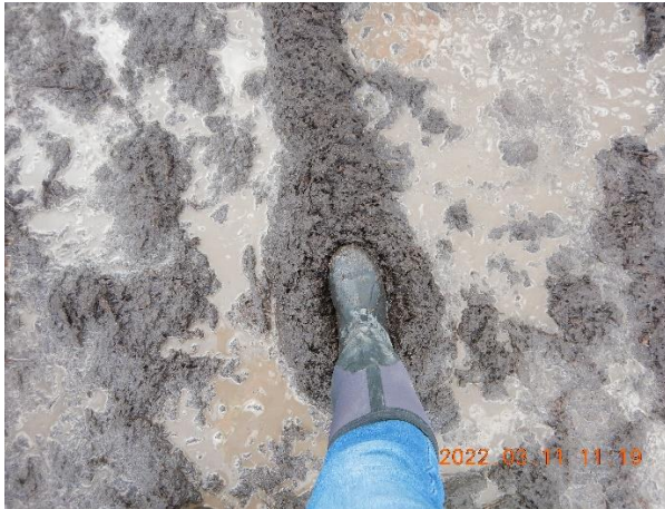
Pictures 4c and 4d: Closeup photos showing the depth of the mud, wood fiber, bark, and ponded stormwater on top of the paved log deck. The main retention pond receives runoff from this area. Picture taken by Heaven Moore.
