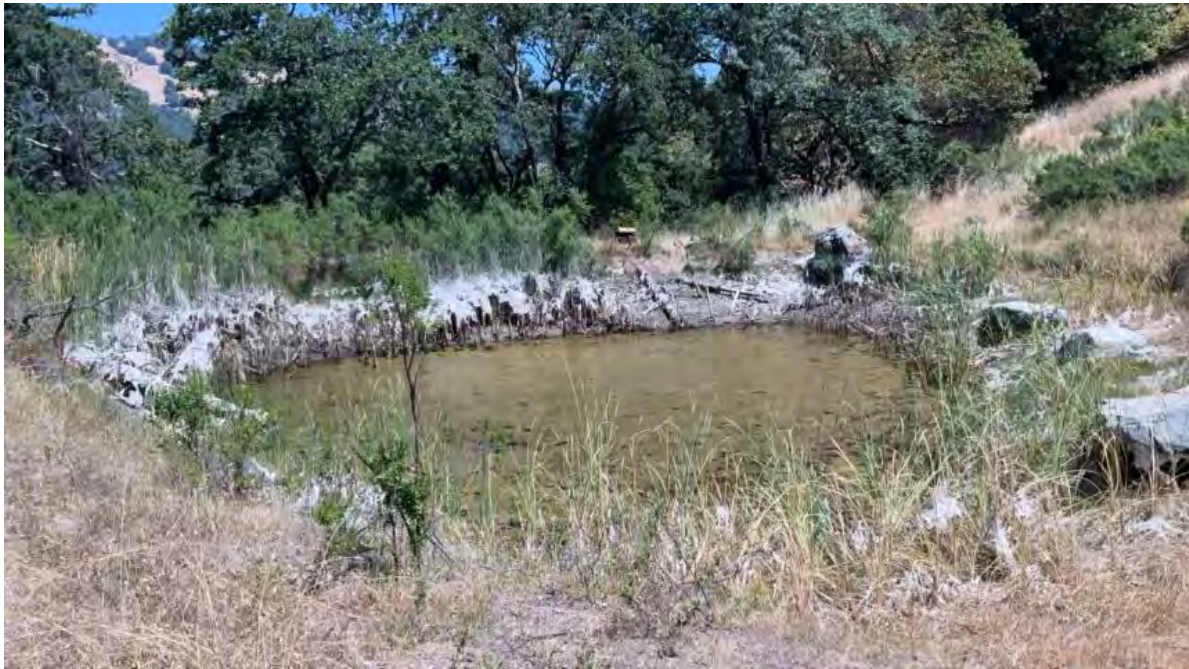
Figure 15. Polygon 3. Unlined excavated water storage pond with earthen berm. No discernable outflow structure. Built at edge of steep slope.
