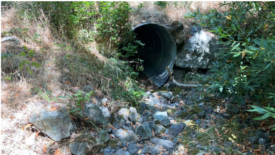
Figure 22. Point 5. Inlet of 52" culvert.
