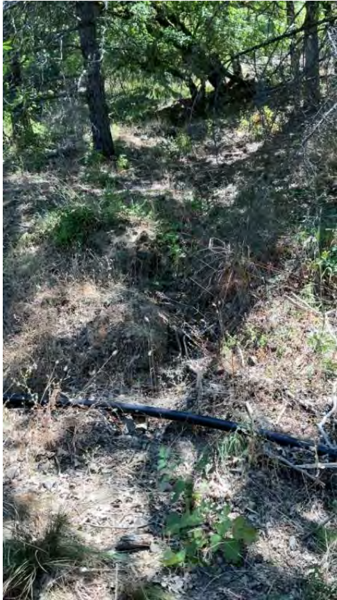
Figure 17. Point 4. A watercourse drains the slope above in a scoured channel, hits the road where there is no crossing, is rerouted down the slope, hits the cultivation flat at Polygon 2, and runs past the greenhouse. View is looking upslope.
