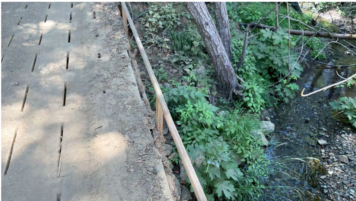
Figure 7. Point feature 1 – bridge over Class II.
