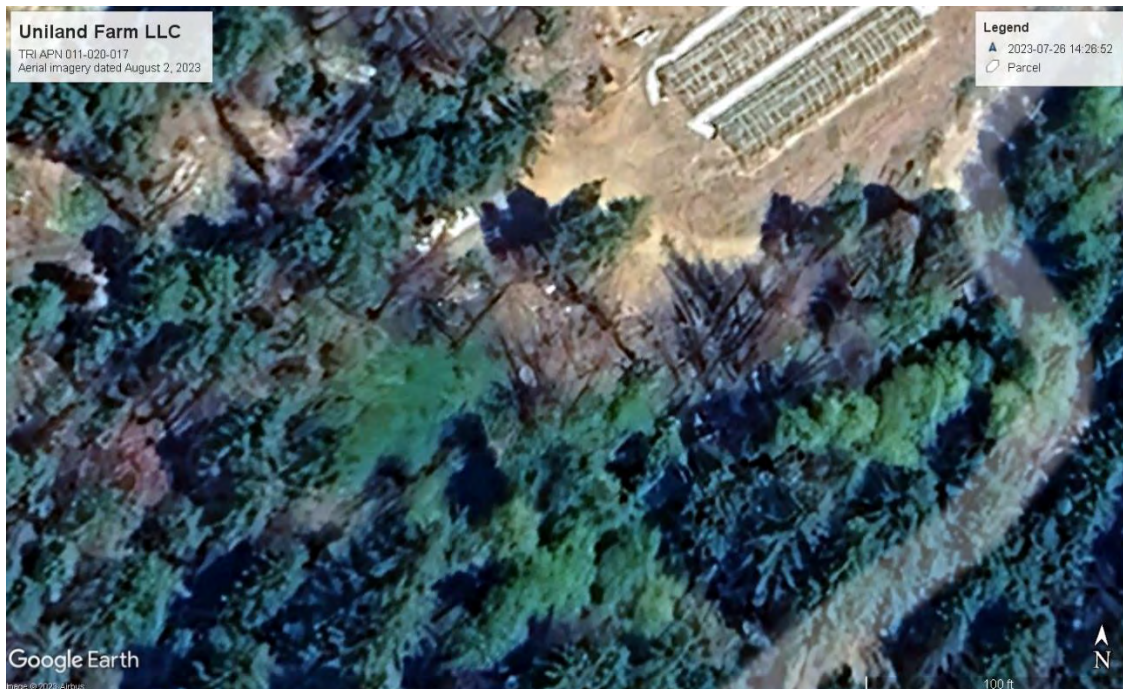
Figure 11. Point feature 2 is a trailer used as a residence with domestic waste and washing machine water being discharged into the edge of a wetland flat, visible as a lush green patch in the right center of the photo.
