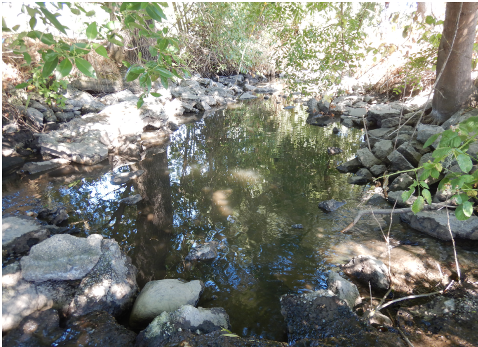
Photograph 4: Photographer is standing on the concrete apron and looking downstream at Santa Rosa Creek channel hardened with broken concrete.
