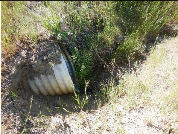
Photo 17– Outlet of the culvert at WQ12
