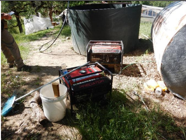
Photo 31 - Uncontained generators in the vicinity of WQ22
