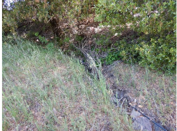
Photo 42 – a watercourse channel just below the trash at WQ15
