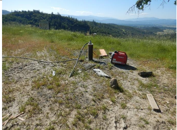
Photo 30 – Ground water well and uncontained generator at WQ4
