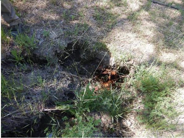
Photo 23 - Inlet of a culverted stream crossing at WQ28
