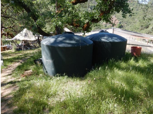
Photo 29 - Water storage tanks near WQ22
