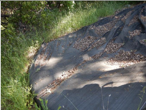
Photo 27 - Water bladder without containment at WQ11
