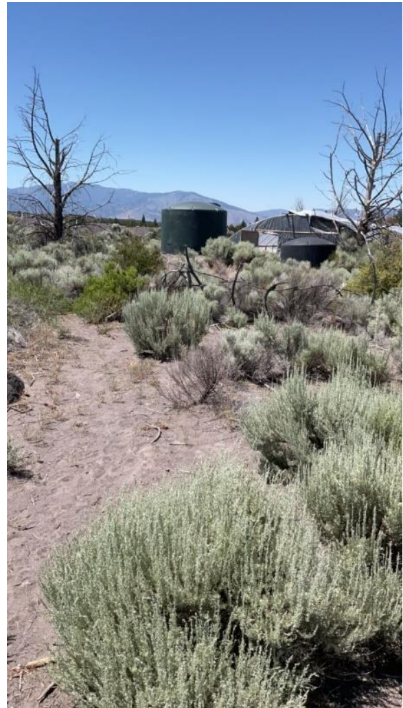
Figure 5. Water tank filled from well. A charged water line from the tank was going to an adjacent property, APN 100-453-070.
