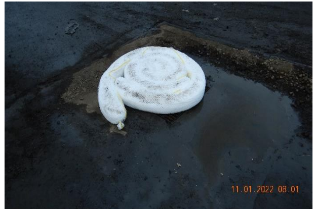
Picture 14a and 14b – View of the absorbent socks placed on top of a DI beneath the steel plate in the central portion of the facility. Picture taken by Farzad Kasmaei.
