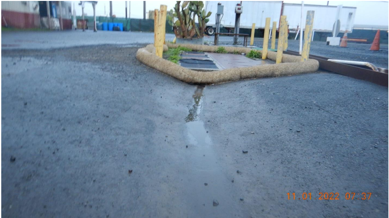
Picture 4 – View of the vditch that drains the facility runoff from the processing area into the filtration system. Picture taken by Farzad Kasmaei.
