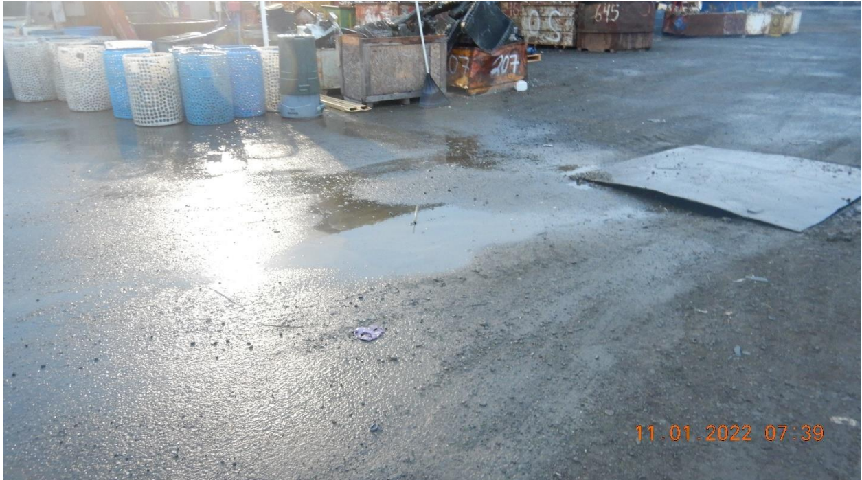
Picture 6 – View of sorted metals inside of the very old and rusty bins exposed to rain. The inlet under the steel plate receives the runoff and then it drains to filtration system. Picture taken by Farzad Kasmaei.
