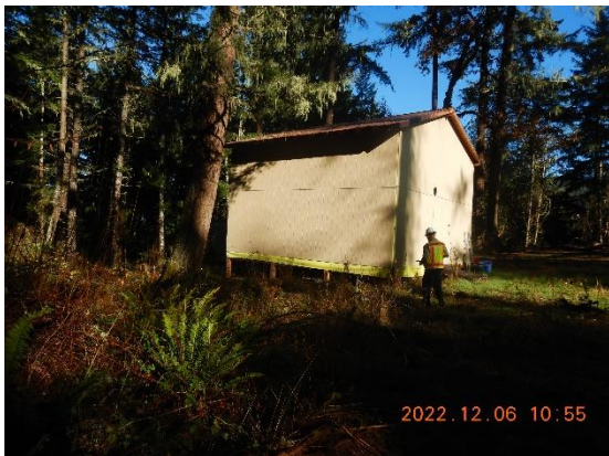
Figure 22. WQ9. Building in Class II setback.
