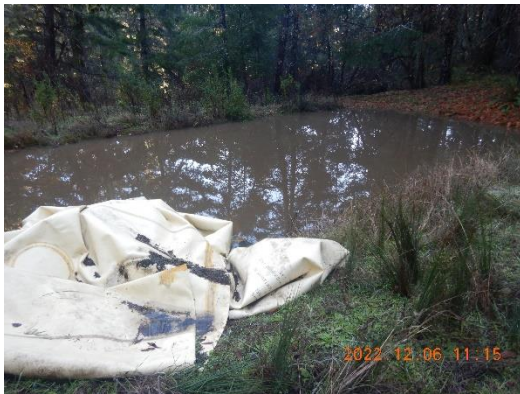
Figure 21. WQ8, bladder pad holding water. Overflow would go down road. Berm should be breached away from road.
