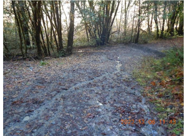
Figure 17. WQ6 - Left bank road approach to second and upper waterbar above WQ4.
