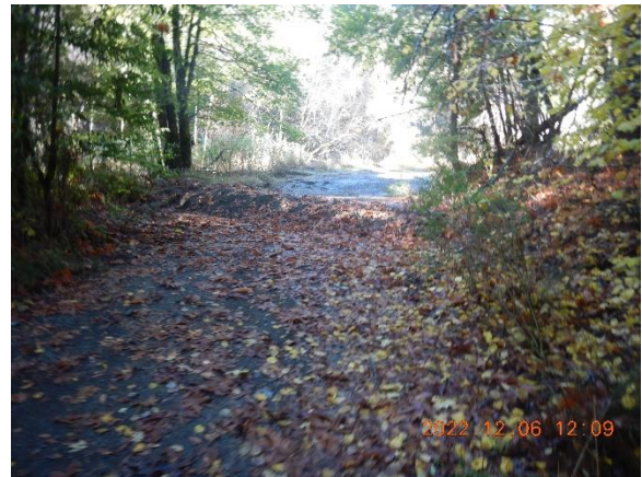
Figure 12. Water bar installed in 2022.
