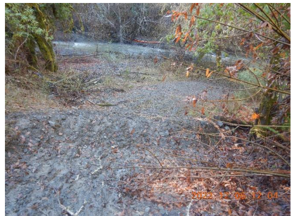
Figure 13. Waterbar on right bank above WQ4.
