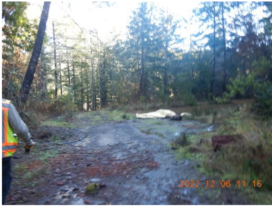
Figure 20. WQ8, bladder pad located next to roadway has berm around it and is holding water.
