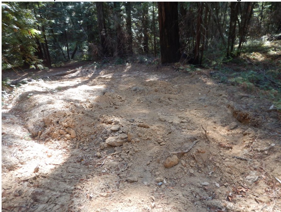
Photo Point 4.2 - Mineral soil blocking outlet of waterbar.
