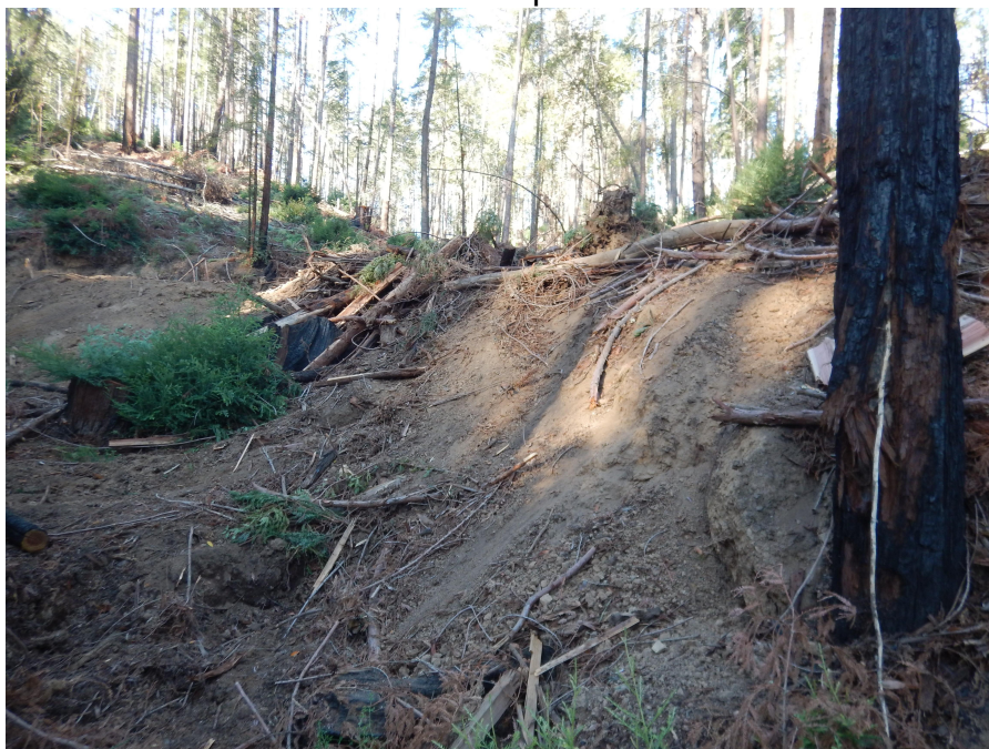
Photo Point 1.5 - Sidecast material from road perched above channel.
