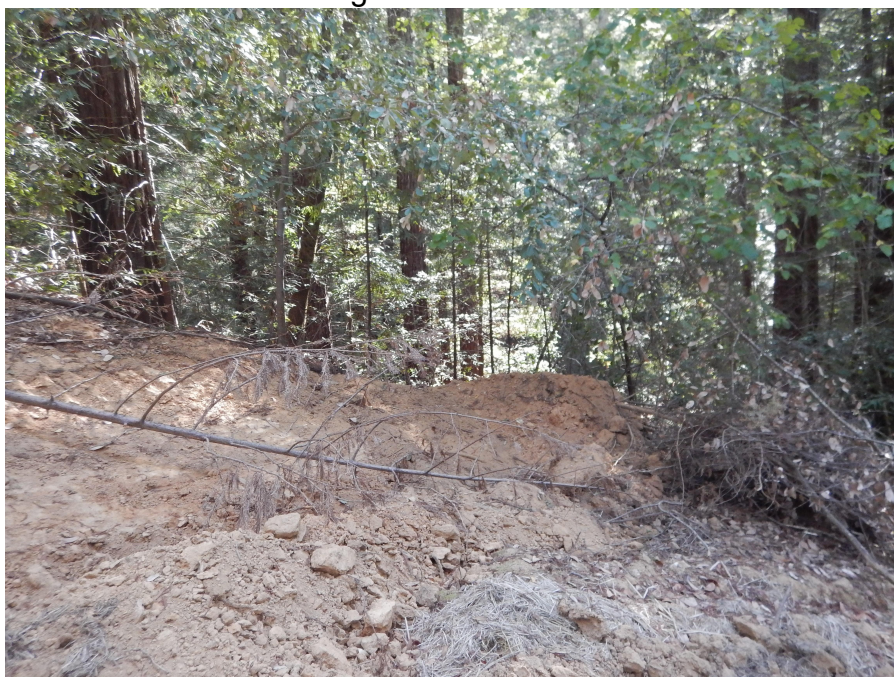
Photo Point 4.2 - Mineral soil blocking outlet of waterbar.
