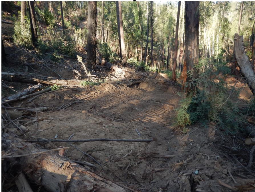
Photo Point 2.1 - Top of skid trail from landing.
