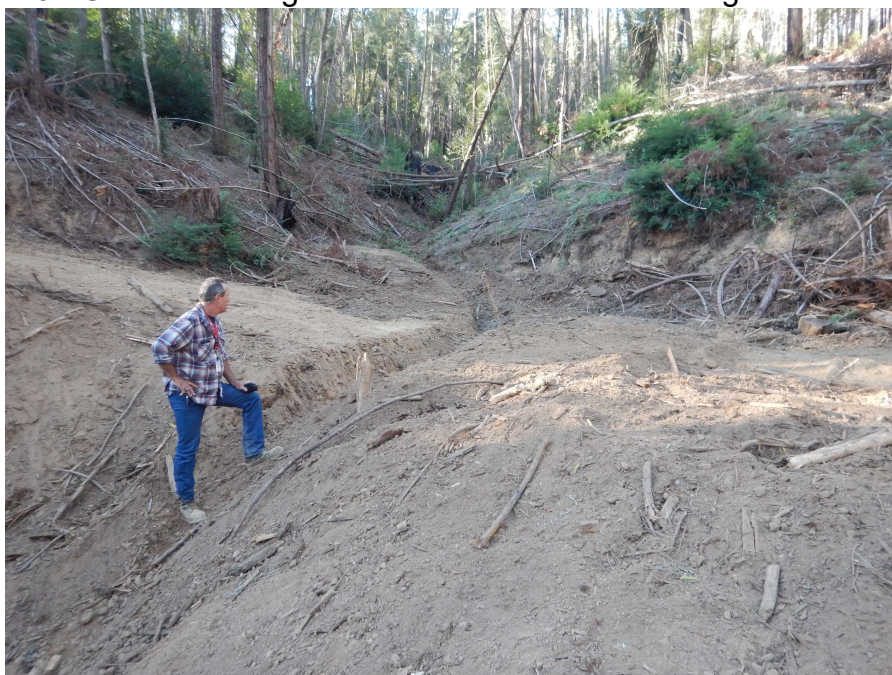
Photo Point 1.6 - Channel through road surface. Not to natural grade.
