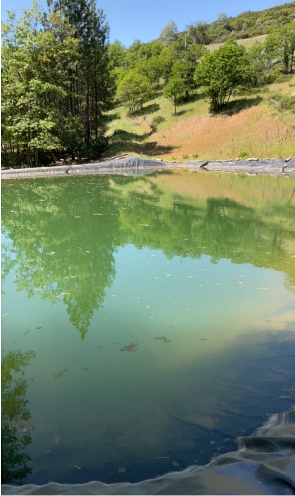
Photos 4 and 5: Pond with black plastic liner capturing hillside runoff. Evidence of overtopping and erosion on the corner nearest to Barker Creek.
