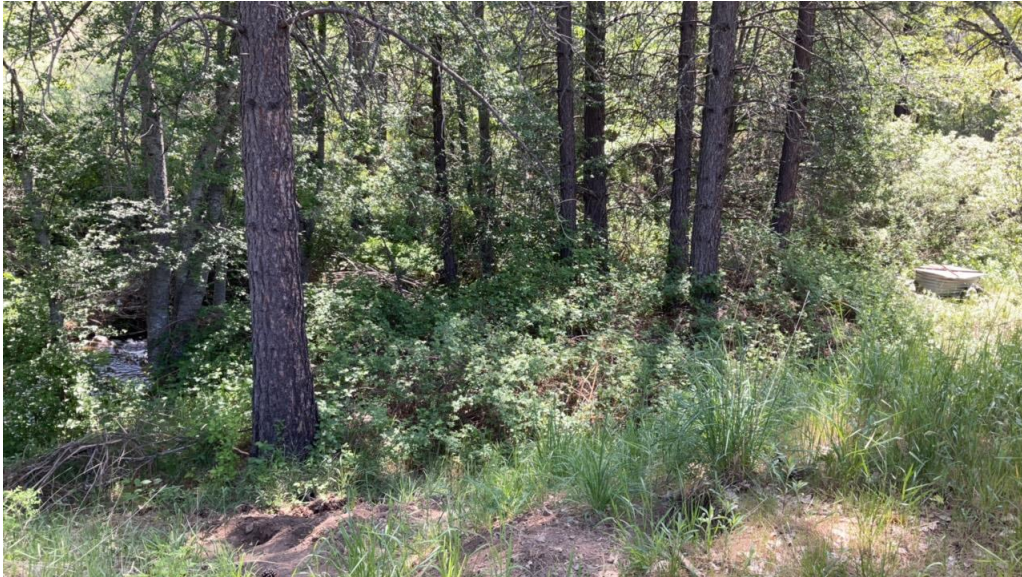
Photo 1: Metal water diversion structure on right side of photo adjacent to Barker Creek.
