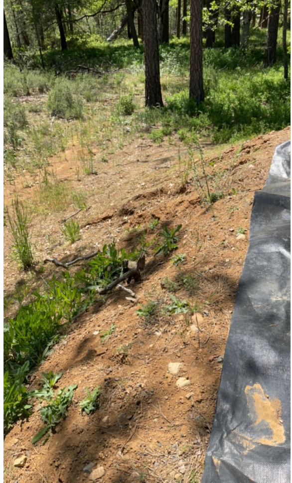
Photos 4 and 5: Pond with black plastic liner capturing hillside runoff. Evidence of overtopping and erosion on the corner nearest to Barker Creek.
