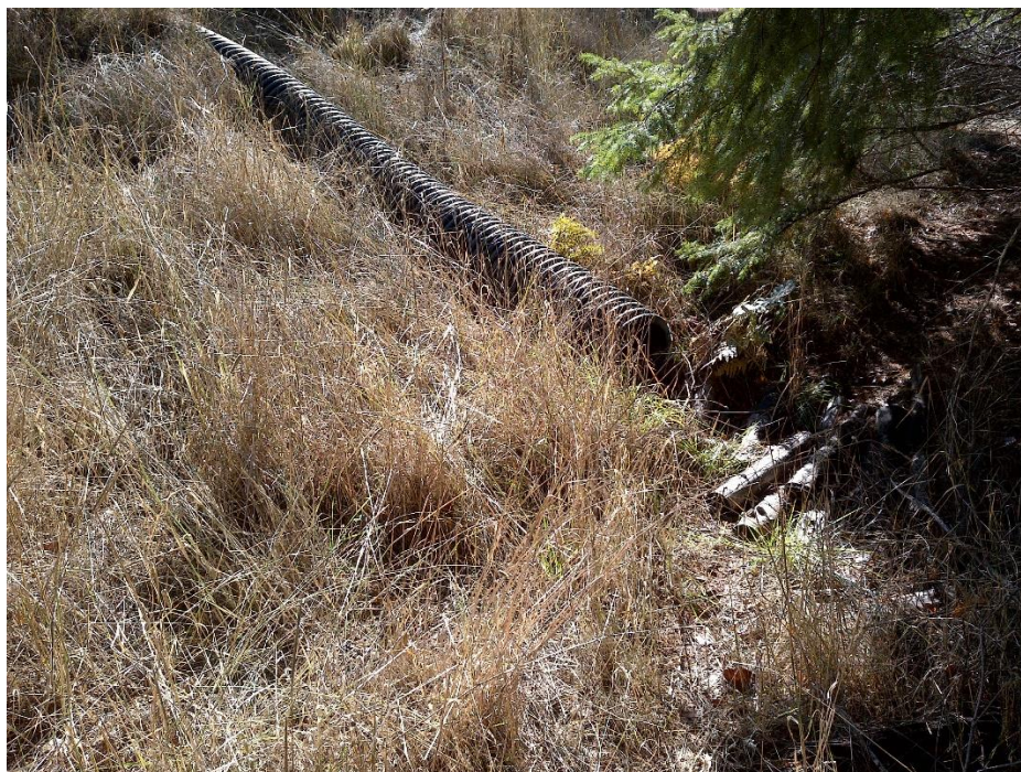
Photo 17—Reservoir outfall at WQ 11. Note the cut logs armoring the channel where the reservoir outfall delivers to the receiving watercourse.
