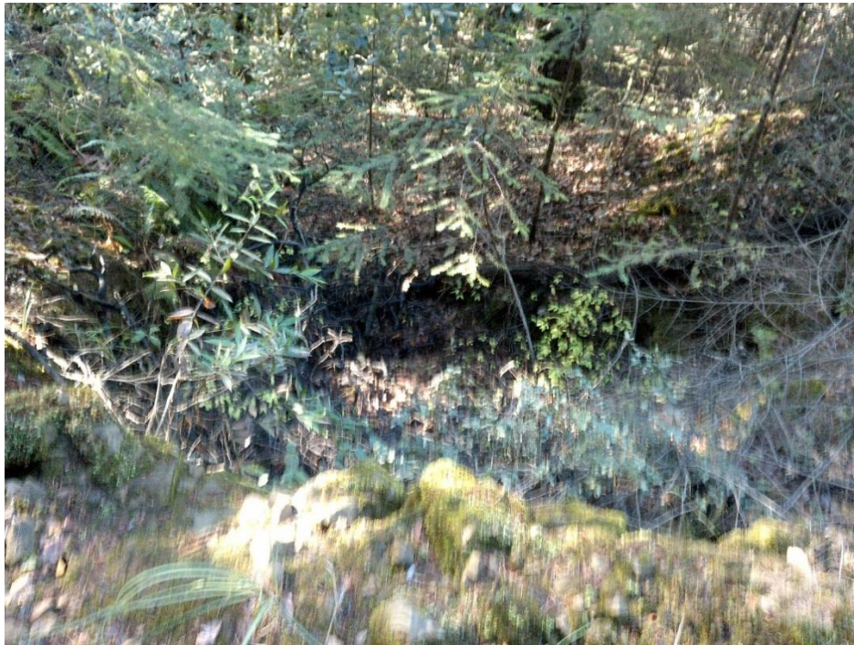
Photo 31—Looking west at receiving waters from culvert at WQ 18
