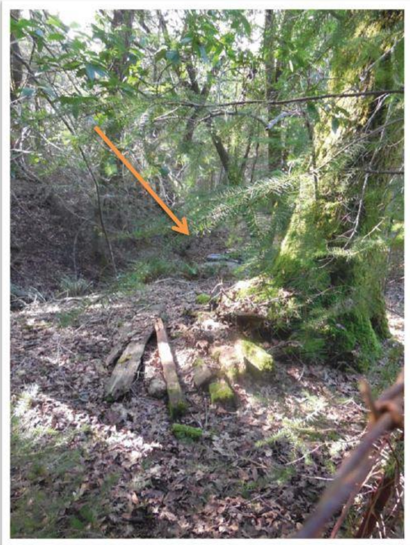
Looking towards the west over fence along access road; the orange arrow points to the tanks in the stream channel.
