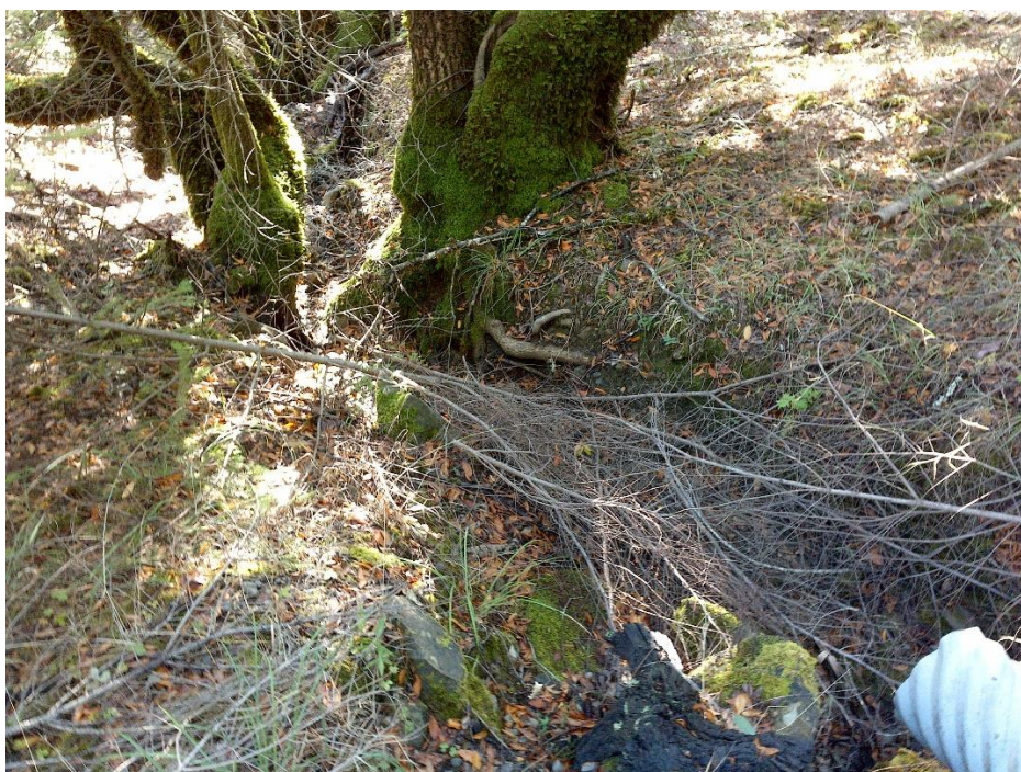
Photo 8—Looking west at culvert outlet at WQ 6.
