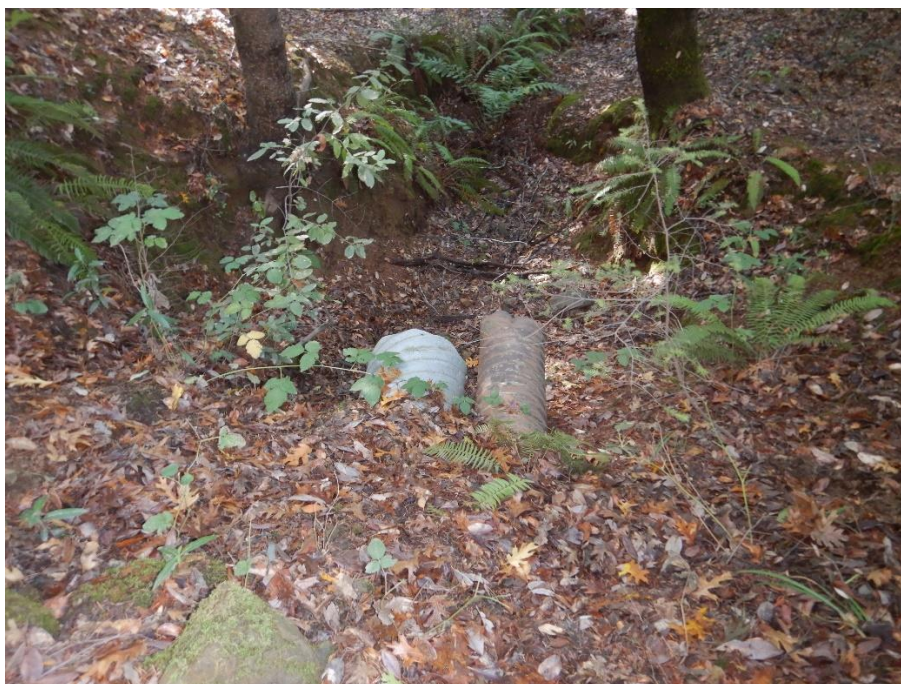
Photo 26—Looking downstream at two culverts, 12 inch and 18 inches in diameter, directed to an approximately five-foot-wide watercourse at WQ 16.
