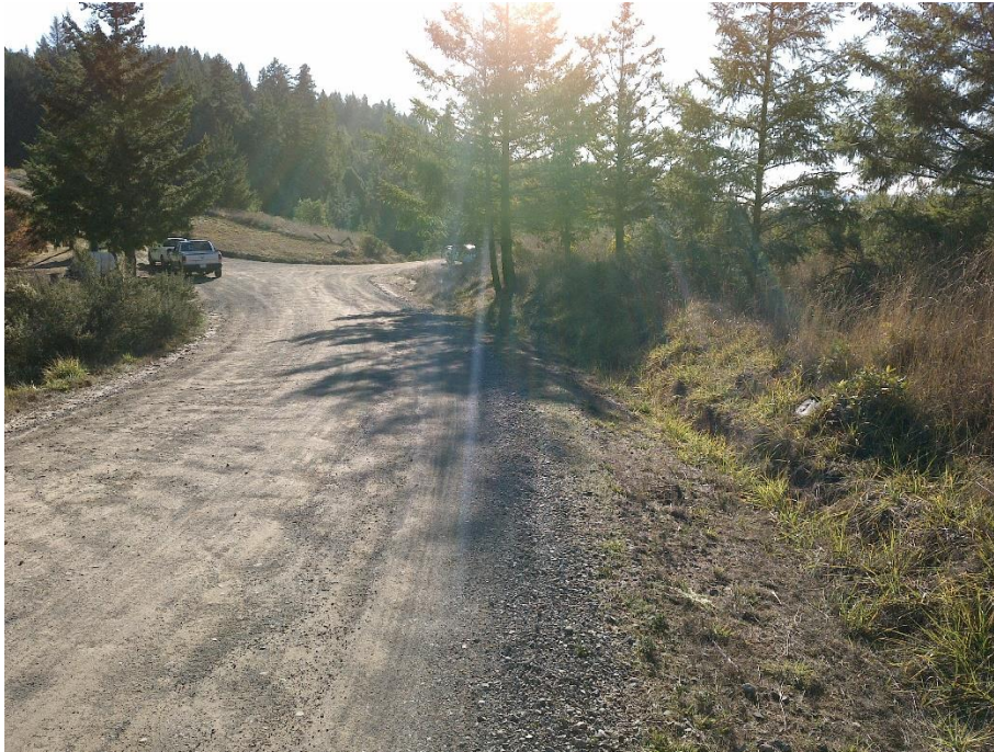
Photo 1—Looking south from WQ 1 toward WQ 2. Road collects stormwater and discharges to inboard ditch, shown in the right of the image before discharging into incising channel at WQ 2 pictured in the below photo.
