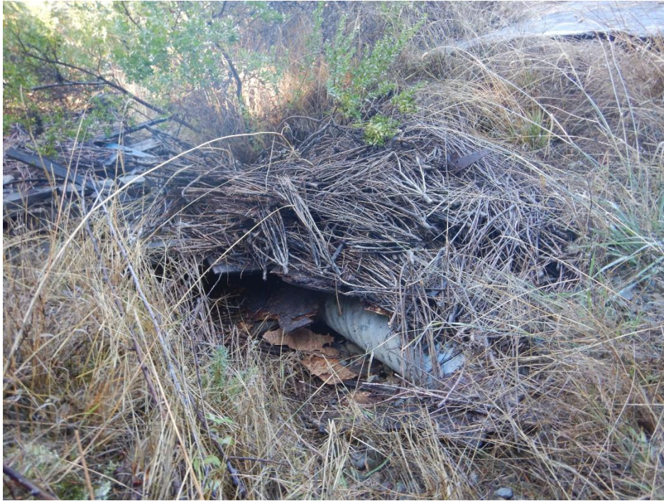
Photo 21—A buried culvert where a legacy road crosses the watercourse at WQ 13.
