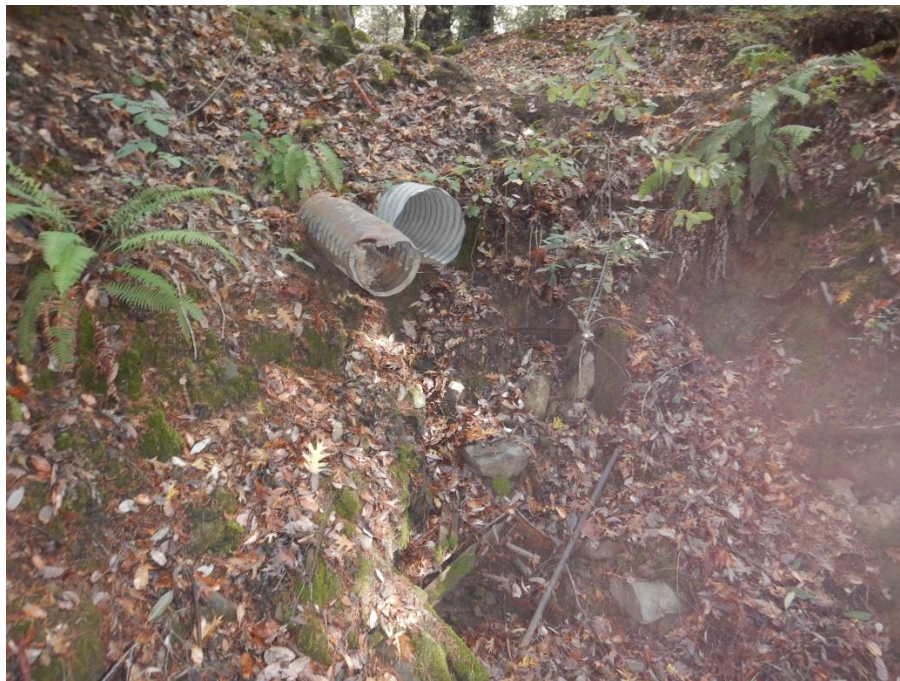
Photo 27—Looking upstream at the two culverts pictured in the previous image perched five feet above the receiving watercourse at WQ 16.
