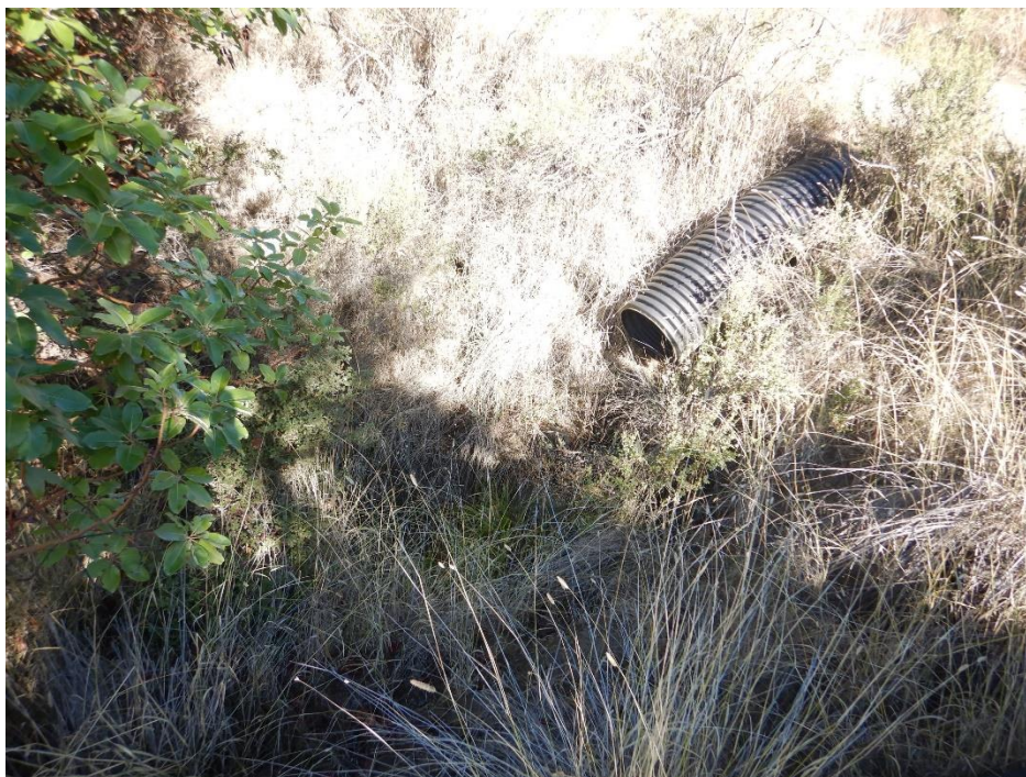
Photo 11—A 24-inch diameter corrugated plastic pipe extending from the road fill at WQ 9.
