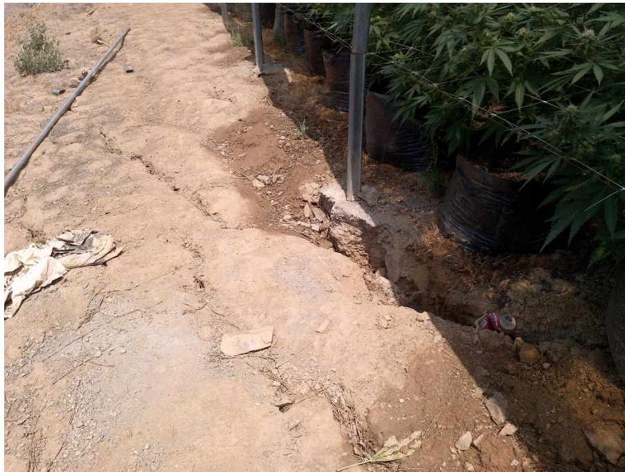
Figure 13—Photo showing the western edge of the cultivation pad located at WQ8. An erosional gully is visible adjacent to cannabis plants in the right of the image and tension cracks are visible in the left of the image.
