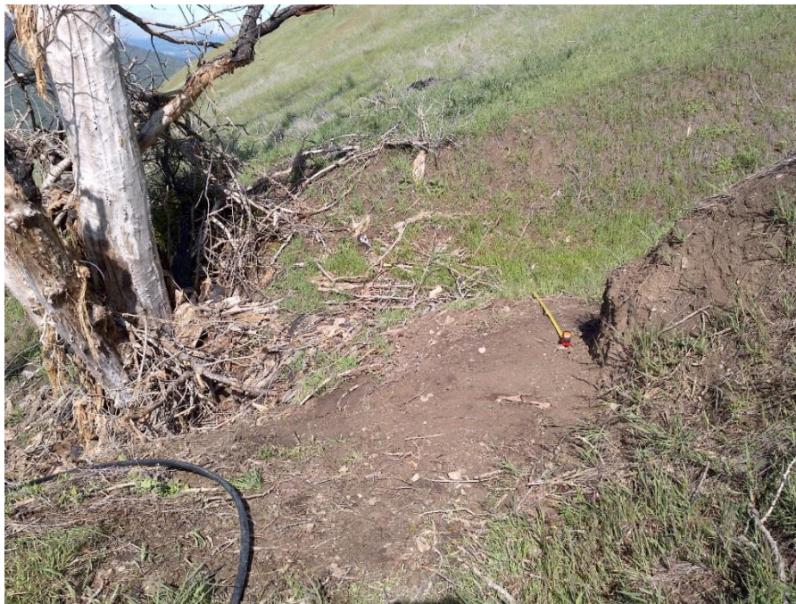
Figure 12—Looking west where an earthen pad extends into the watercourse at WQ5. The dead tree in the left of the image is also visible in the previous image. Approximately 18 cubic feet of earthen fill has been placed into the channel; a patch six feet square averaging six inches deep.
