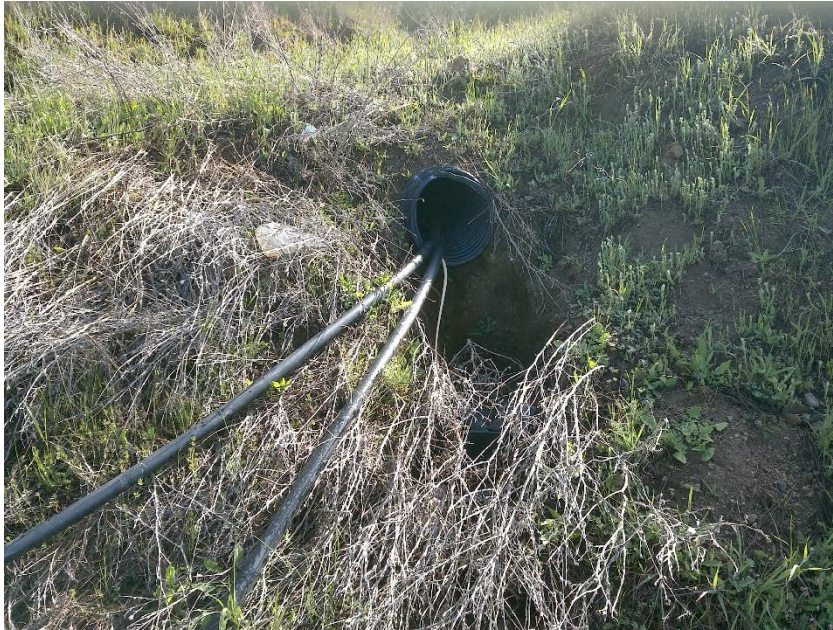
Figure 10—Looking north at culverted watercourse crossing at WQ4. The culvert is perched approximately two feet above the channel bed.
