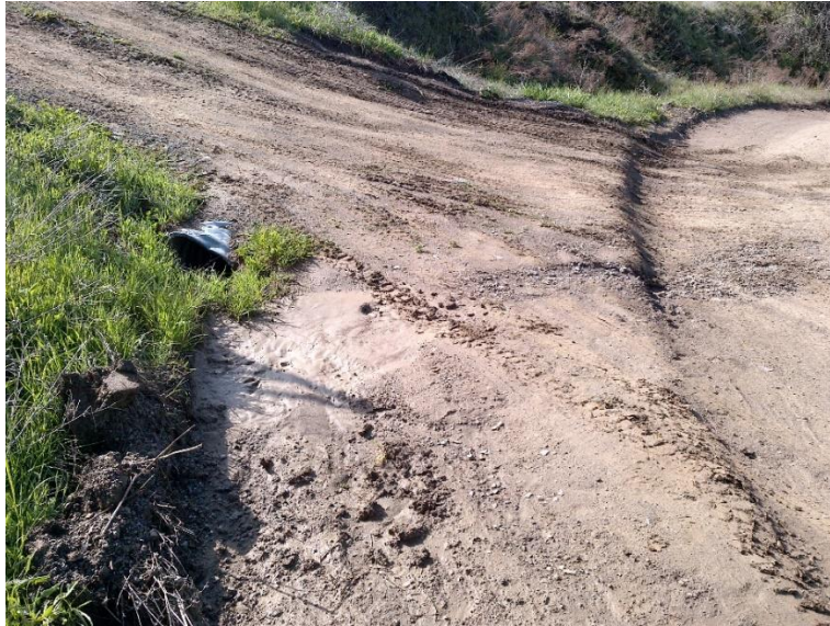
Figure 4—Looking south at WQ1 at the intersection of the gated access to the Property to the left and the shared-use access road to the right. The road has been graded such that stormwater will flow across the road instead of through the culvert pictured in the left of the image.
