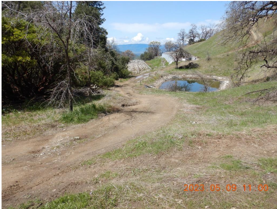
Figure 22—Looking west toward reservoir at WQ9 and greenhouses at WQ8. The topography is shaped such that flowing water from the stream behind the photographer would enter the road and flow into the reservoir in the upper right of the image.
