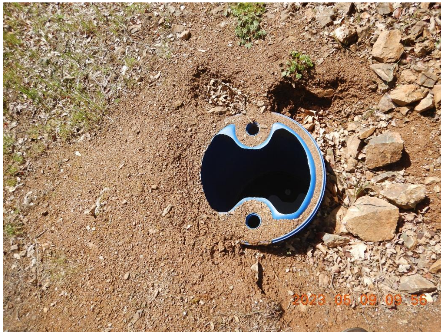
Figure 13— Buried plastic drum within area of large trash pile at WQ3.
