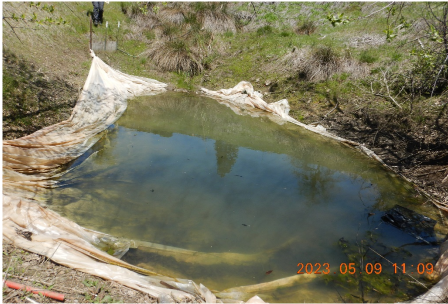
Figure 28—Plastic sheet covering dredged wetlands at WQ11.
