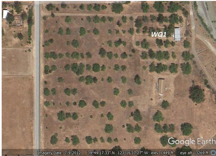
Figure 2—Aerial image of the Property taken on July 9, 2012, obtained from Google Earth. The image shows a structure but no greenhouses on the Property.
