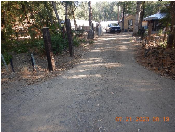
Photo 9 – photo taken of the road section at WQ10
