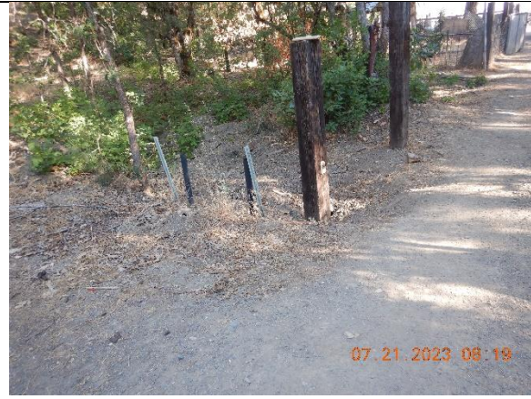
Photo 8 – Culverted watercourse crossing the inlet side at WQ10
