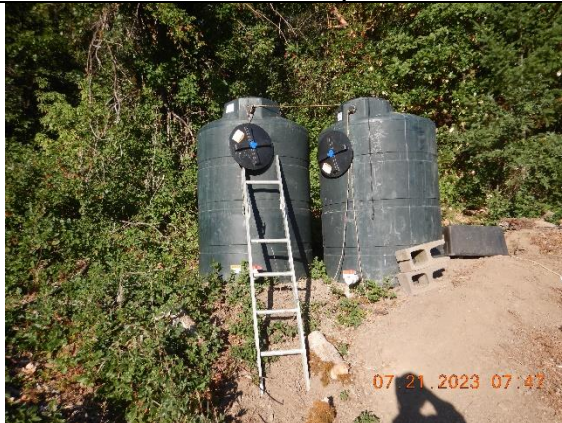
Photo 16 – Water storage tank on a steep slope at WQ4
