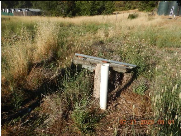
Photo 19 – Groundwater well at WQ8
