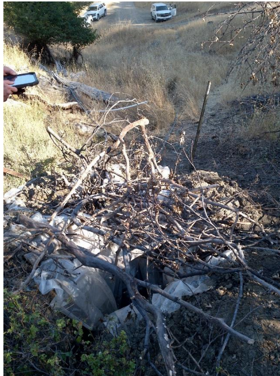
Figure 10—Photo showing a developed spring at WQ6. The spring has a four-foot-deep hole lined with plastic sheeting and one foot of standing water in the bottom.
