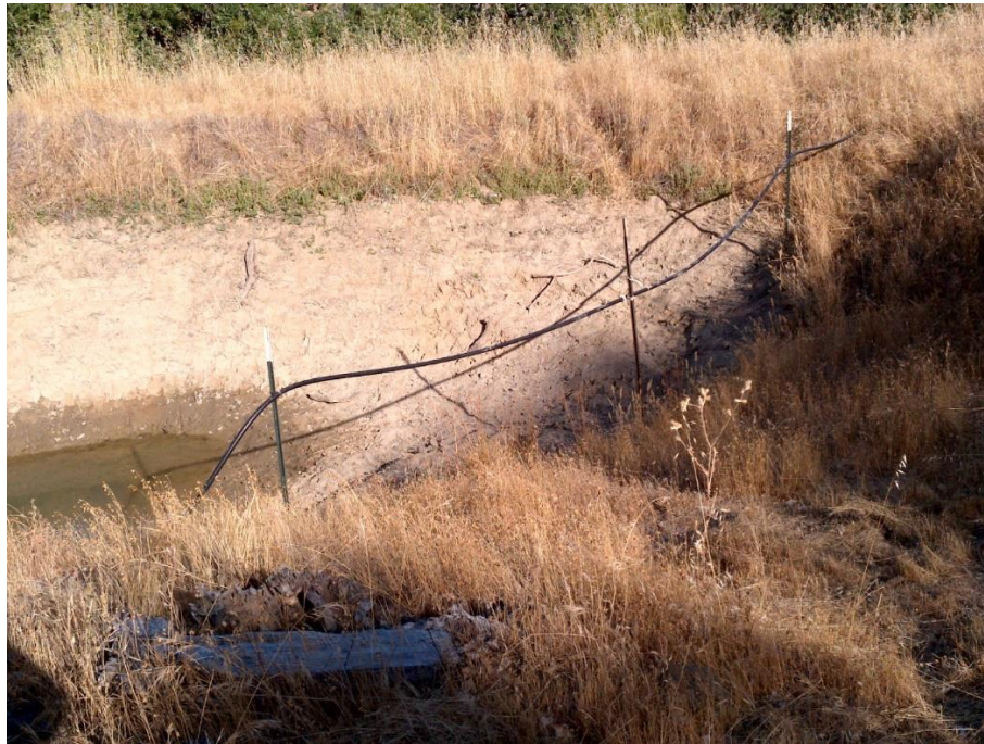
Figure 12—Photo looking north at eastern edge of pond located at WQ7.
