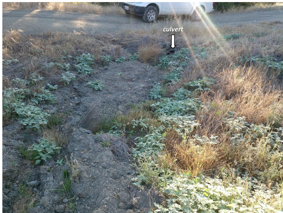
Figure 5—Photo looking east and downslope towards WQ3 from the same location as the previous image. Lobes of sediment are visible between the photographer and a culvert inlet marked by an arrow in the top middle of the image.
