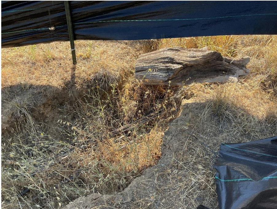
Figure 7—Bottom of fence pictured in the previous image at WQ2. A channel is visible passing under the fence.
