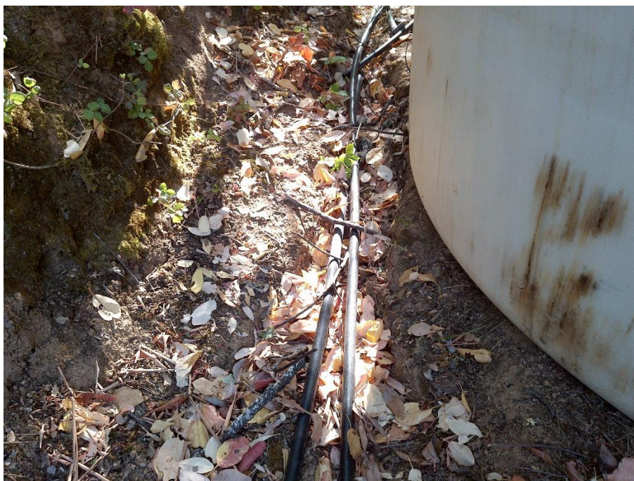
Figure 5—Photo looking at the ground adjacent to water tanks at WQ1. A channel/rill is visible with black plastic tubing laying in the rill.
