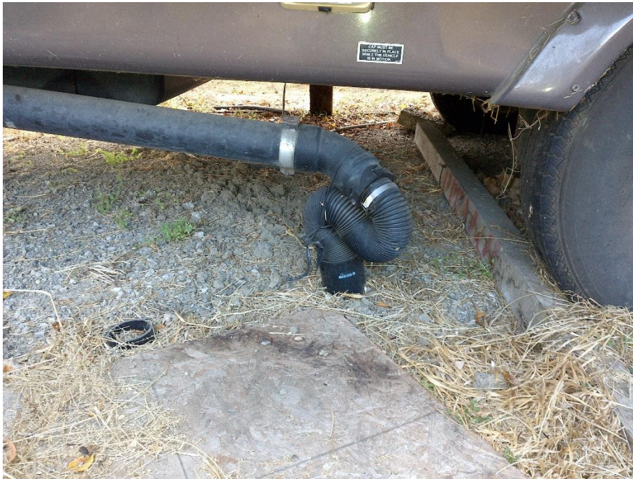
Figure 20—A photo showing the sewage drain line from a trailer being directed into a pipe in the ground at WQ7.
