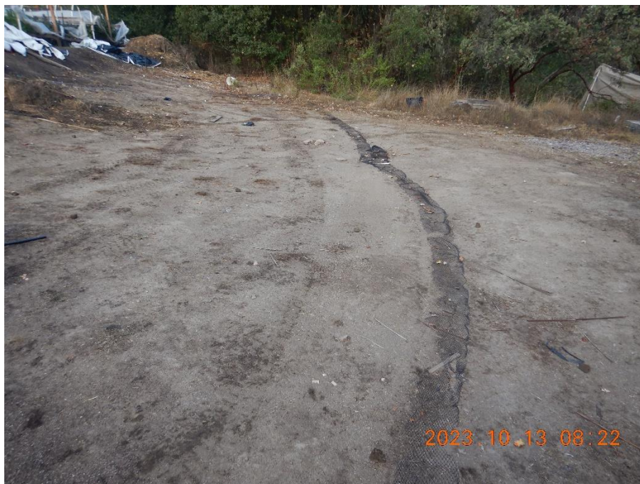
Figure 18—A photo looking west at an area of bare earth south of WQ6. The greenhouses at WQ1 are visible in the top left of the image and empty black plastic netting is visible in the middle of the image.
