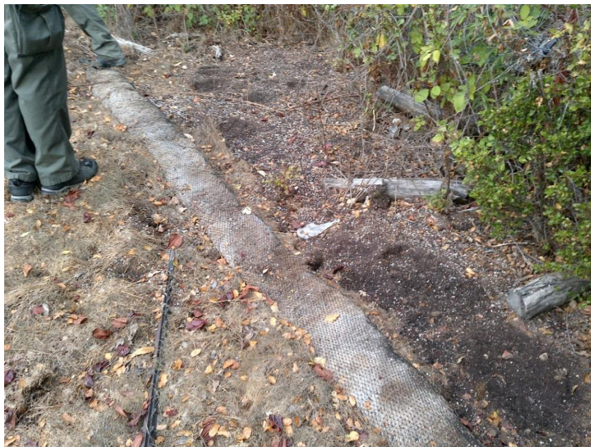
Figure 17—A photo looking northwest at the thin wattle pictured in the previous image at WQ5. The cultivation pad is to the left of the wattle and Salt Hollow Creek is to the right of the wattle. Imported potting soils, identifiable by the white speckles of perlite and dark color, are also visible on the right side of the wattle. The wattle has degraded such that stormwater may flow over the wattle.
