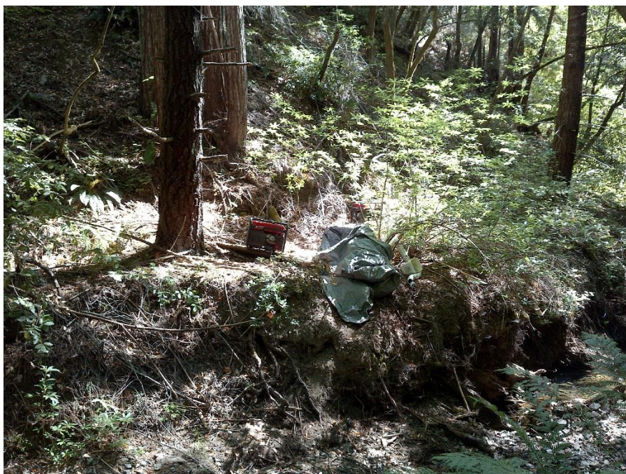
Figure 11—Photo showing two petroleum powered generators without secondary containment. The generators are located adjacent to a watercourse visible in the lower right of the image.
