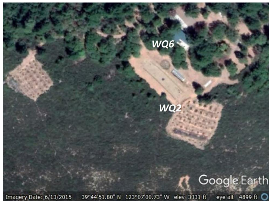
Figure 5—Aerial image of the Property taken on June 13, 2015, obtained from Google Earth. The image shows a cleared area south of WQ6 with a rectangular frame at the location of where a hoop-type greenhouse was observed during the August 23, 2023 inspection.
