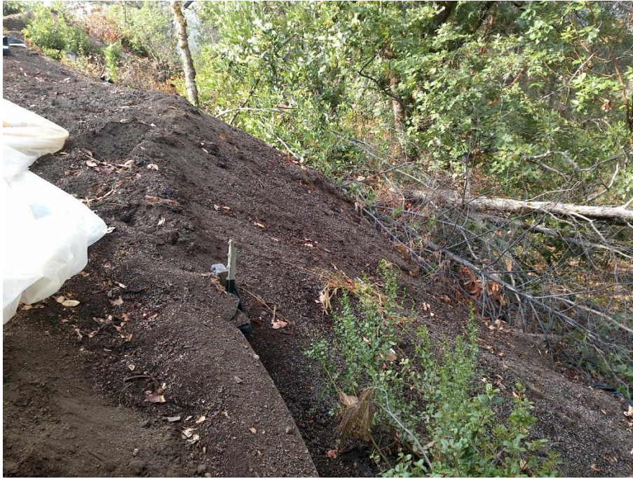
Figure 20—Photo of the western edge of the cannabis cultivation pad located at WQ8. Waste potting soils, identifiable from the white speckles of perlite contained in the soils, cover the downslope side of the pad.
