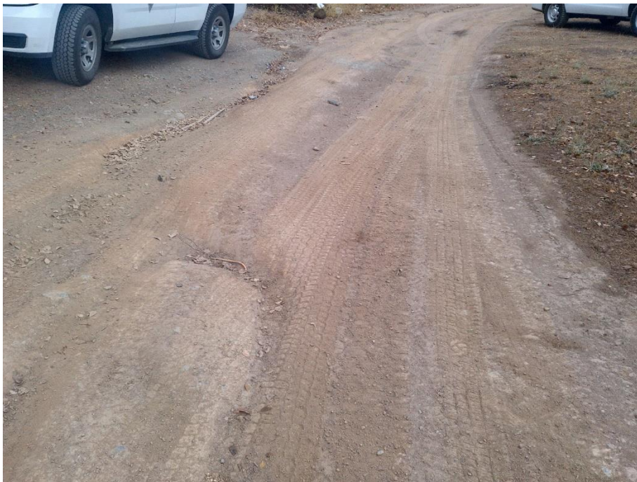
Figure 7—Photo of the dirt road in the vicinity of WQ1. Erosional rills are visible on the road surface.
