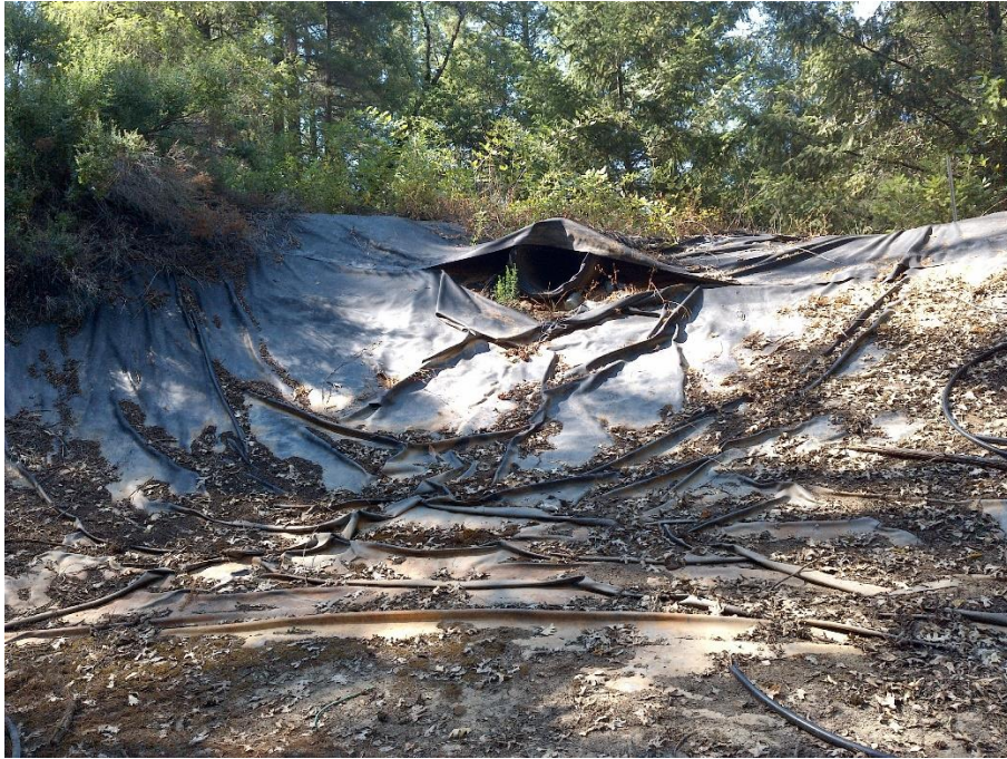
Figure 8—Photo looking north at reservoir outlet at WQ1.
