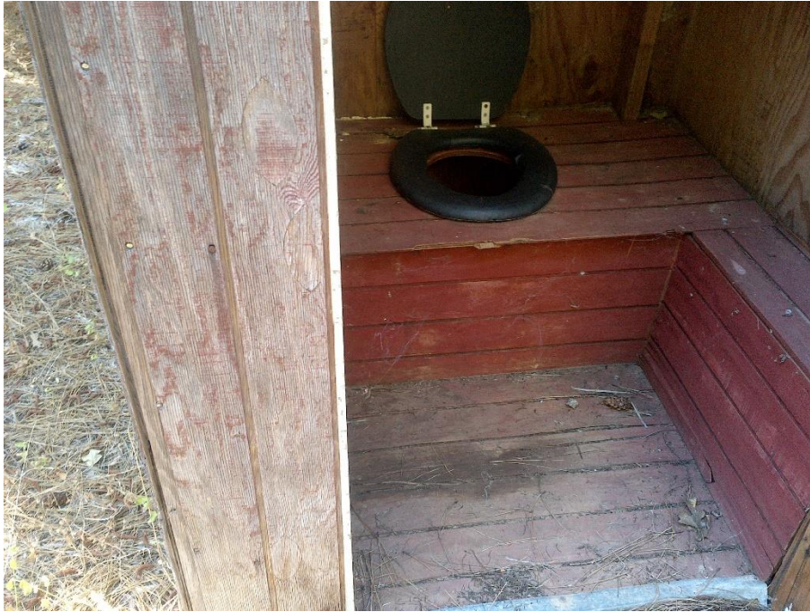
Figure 16—Photo showing small structure with pit-toilet located near to a residential structure at WQ5.
