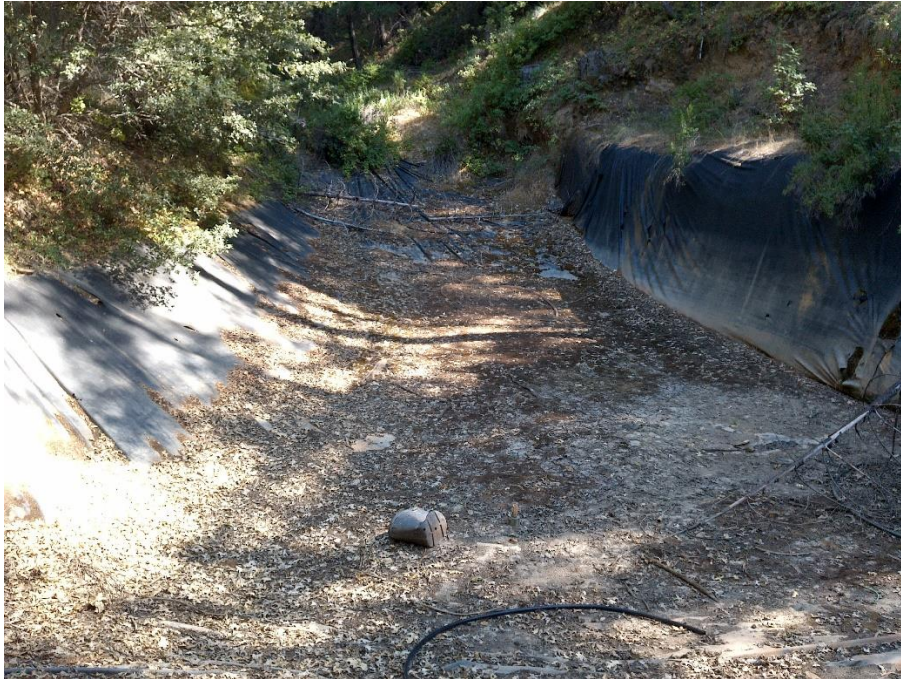
Figure 6—Photo looking south at onstream reservoir located at WQ1. The reservoir is dry and lined with a black material.
