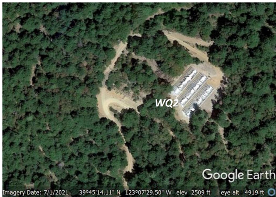
Figure 5—Aerial image of the Property taken on July 1, 2021, obtained from Google Earth. The image shows a cultivation pad with three hoop-type greenhouses at WQ2
