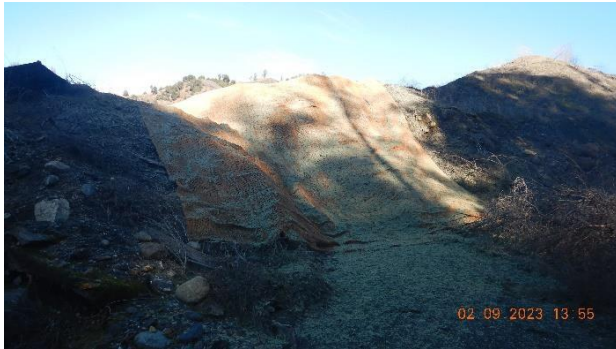
Pictures 6a, 6b – View of the erodible creek slope stabilized with BFM and netting in accordance with the CAO requirements. Picture taken by Farzad Kasmaei.
