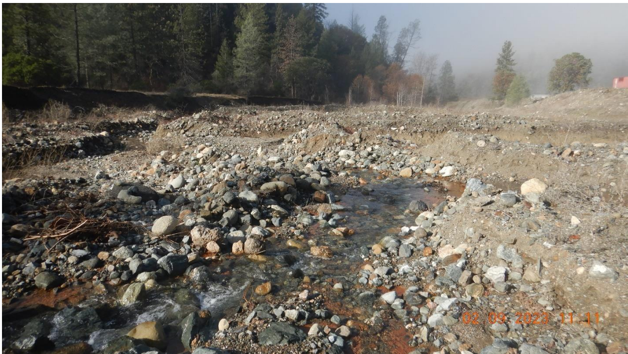
Picture 3- View of large berms that were installed by Facility staff in Oregon Gulch on the south side of the facility. Picture taken by Farzad Kasmaei.
