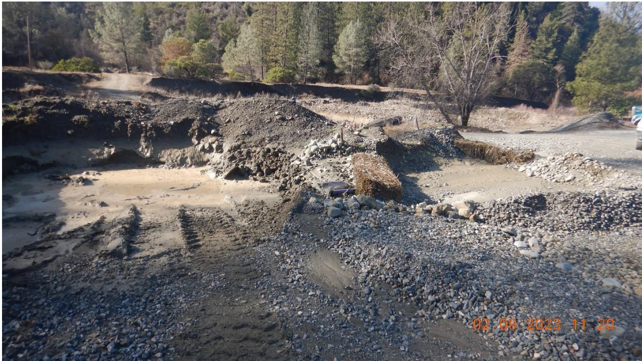
Picture 2- View of sediment traps in vicinity of the discharge point (DP-4) located at southeast corner of the existing concrete ready mix. Picture taken by Farzad Kasmaei.
