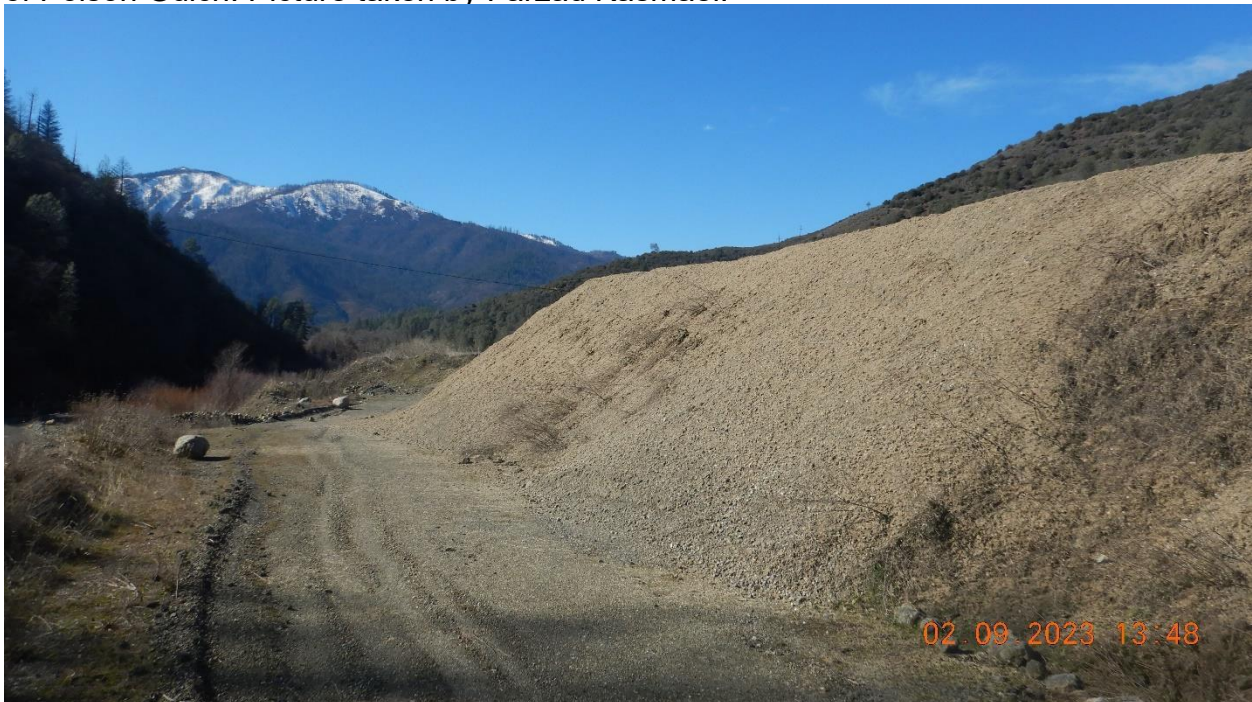
Picture 5 - Looking west at the office area berm that has been stabilized temporarily with BFM materials in accordance with the CAO requirements. Picture taken by Farzad Kasmaei.
