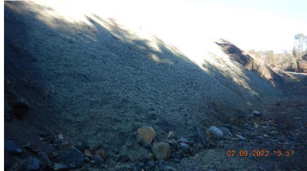
Pictures 6a, 6b – View of the erodible creek slope stabilized with BFM and netting in accordance with the CAO requirements. Picture taken by Farzad Kasmaei.
