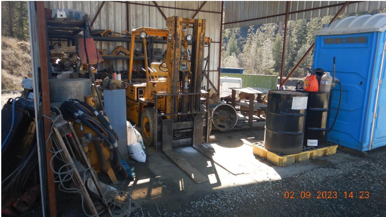
Picture 8 - View of the fueling storage area that was maintained. Significant improvements made to this area since last inspection and no spills were observed on the ground. Picture taken by Farzad Kasmaei.
