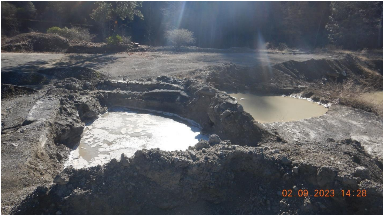
Picture 9- Looking east at couple of unlined concrete wastewater ponds on the west side of the facility. Picture taken by Farzad Kasmaei.
