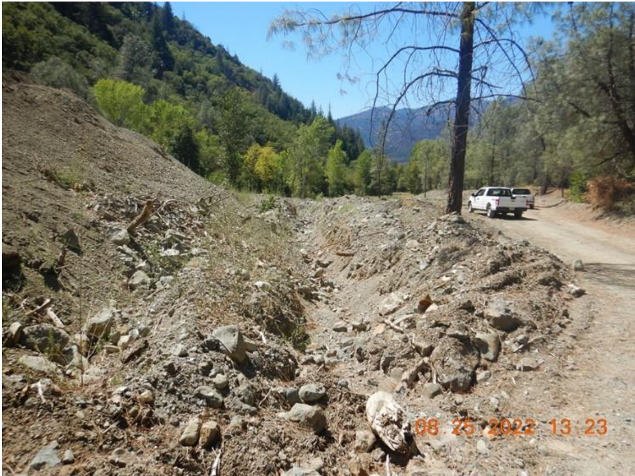
Photo 14a: Access road drainage crossing, facing downstream.
