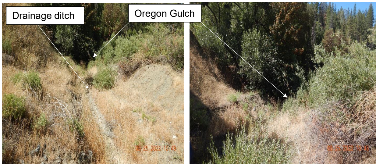
Photo 4a, 4b: Looking southwest at a shallow drainage ditch that drains into Oregon Gulch. Potential discharge point. Picture taken by Farzad Kasmaei.
