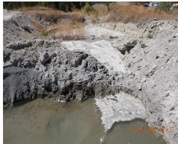
Photos 13a, 13b: looking east at existing concrete washout ponds that are not lined. Picture taken by Farzad Kasmaei.
