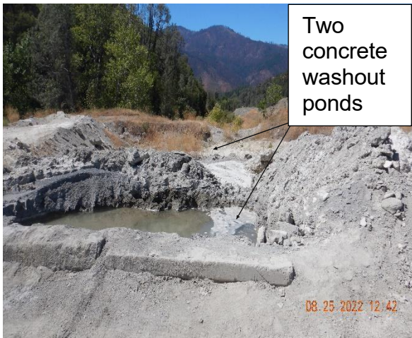
Photos 13a, 13b: looking east at existing concrete washout ponds that are not lined. Picture taken by Farzad Kasmaei.
