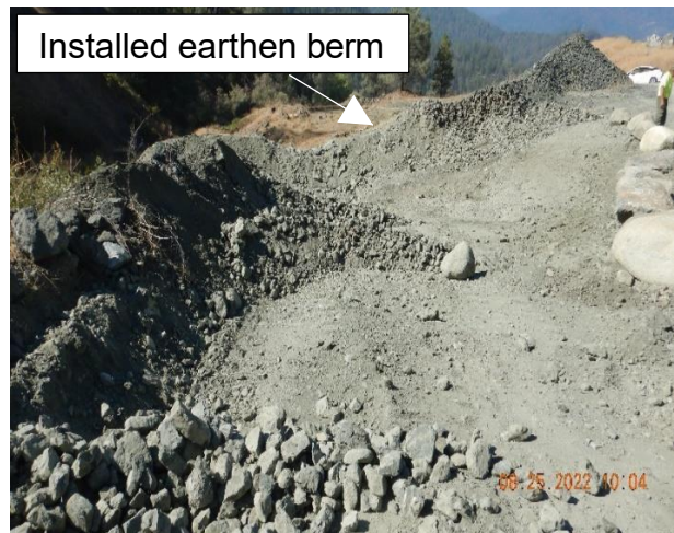
Photo 2a, 2b: Looking northeast at the check dams installed along the earthen berm where the stormwater samples are collected (DP-6) prior to discharging into Oregon Gulch. Picture taken by Farzad Kasmaei.
