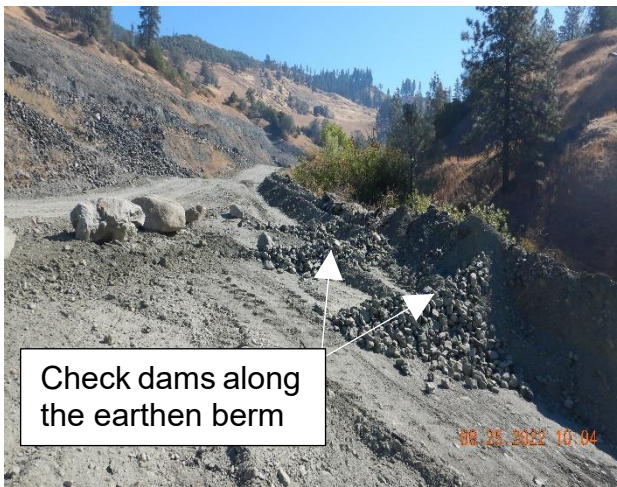
Photo 2a, 2b: Looking northeast at the check dams installed along the earthen berm where the stormwater samples are collected (DP-6) prior to discharging into Oregon Gulch. Picture taken by Farzad Kasmaei.
