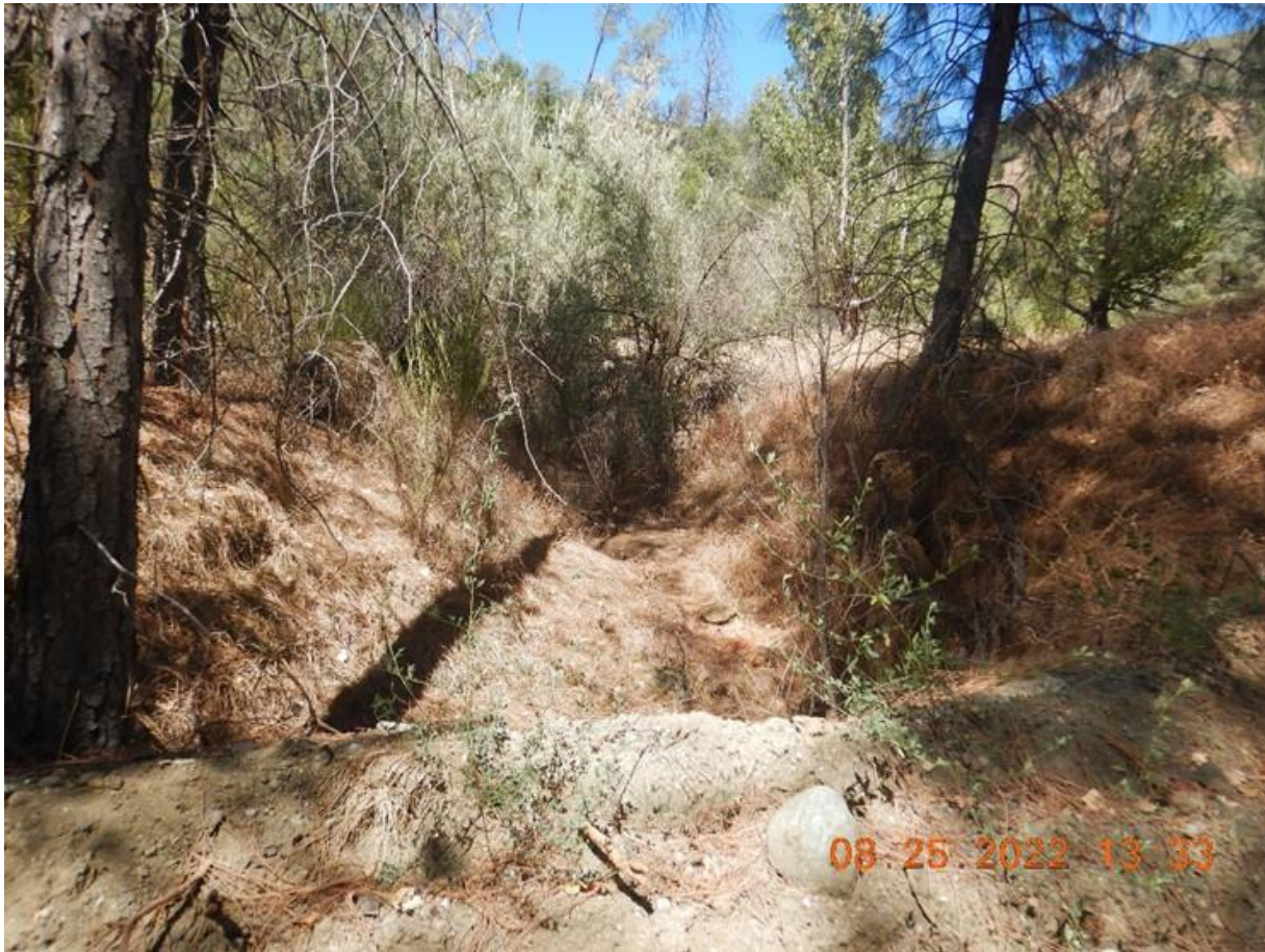
Photo 14b: Drainage swale with road crossing material in foreground.
