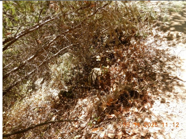
Photo 19 Concrete culverted watercourse crossing outlet at WQ17, installed slightly high in the fill
