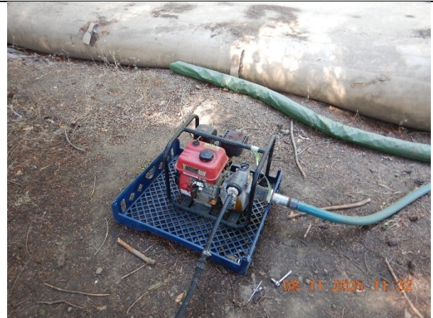
Photo 46 A water pump near WQ18 connected to water storage bladder
