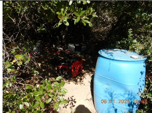
Photo 45 A generator and petroleum product containers without secondary containment or cover near WQ9
