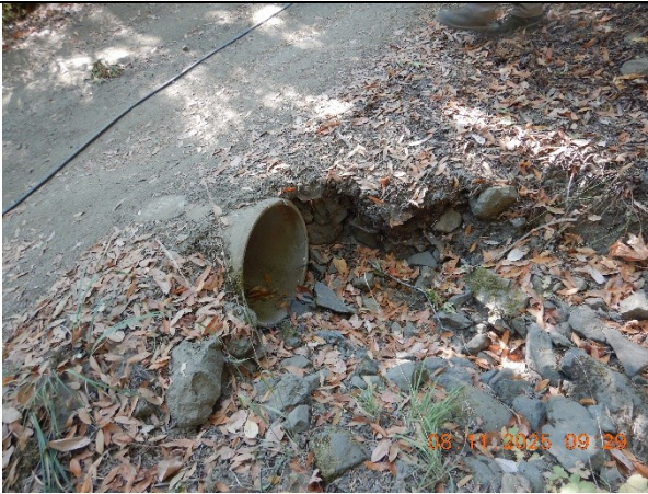
Photo 11 Concrete culverted watercourse crossing inlet at WQ3
