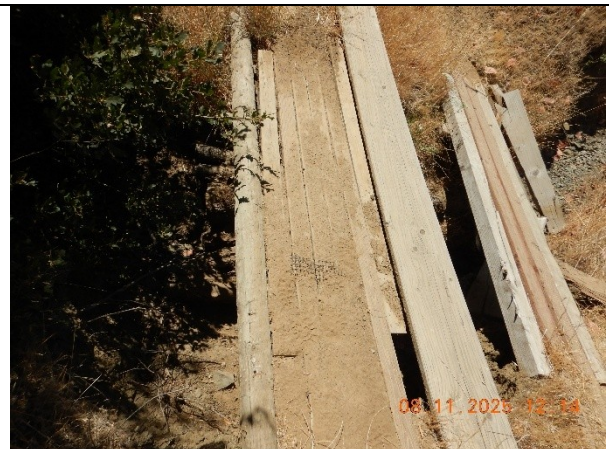
Photo 22 Showing logs placed under the wooden bridge at WQ23
