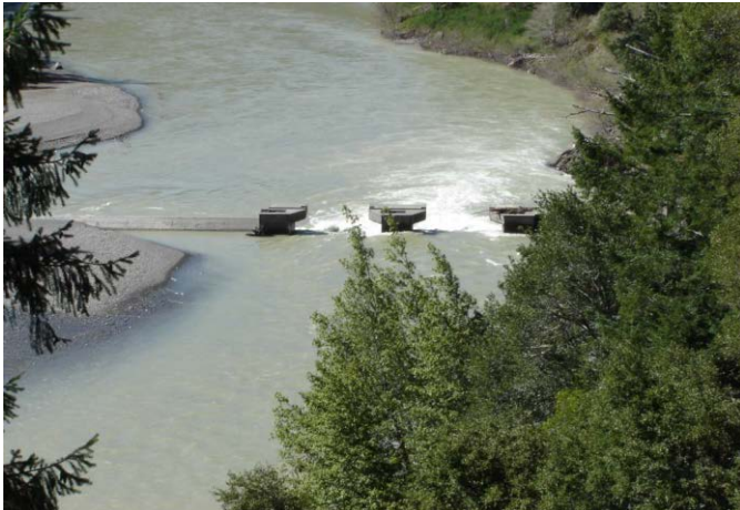
Benbow Dam during flows of approximately 10,000 cfs, March 2011. The river overtops the dam crest at approximately 12,000 cfs. Photo by courtesy of Questa Engineering.
