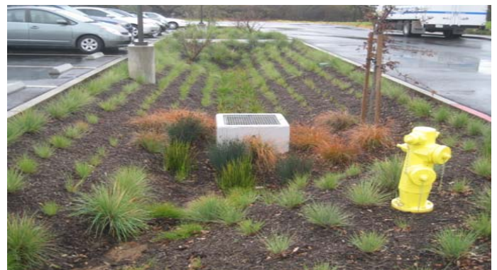
Healdsburg Office Building ~Bio-Retention Swale. Photo by Paul Keiran.
