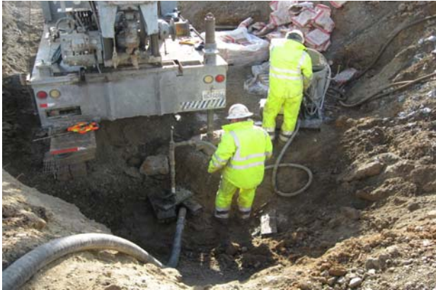
Destruction of a contaminated mill supply well occurred as part of the site remediation. Photo by Cody Walker
