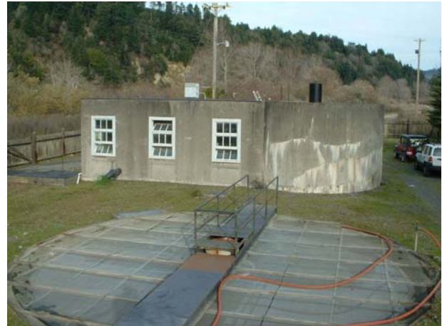
Scotia Wastewater Treatment Facility, Operations Building, and Secondary Clarifier
