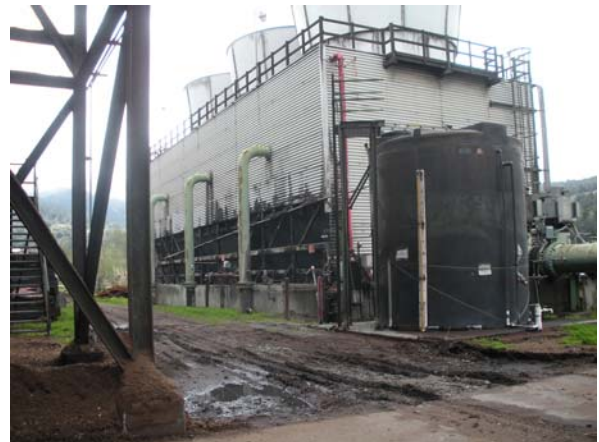
RED-Scotia Power Plant, Cooling Tower B
