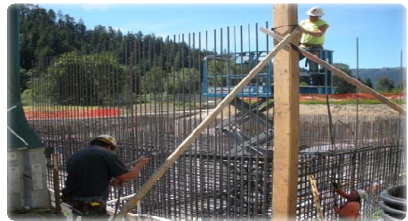
Exterior Construction Aero-Mod Treatment System June 2012. Photo Credit: Lisa Bernard
