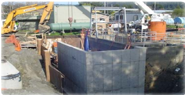
New Headworks Construction March 2010. Photo Credit: Lisa Bernard
