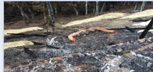
Figure 2. BMP controls installed downslope of a burned structure.
