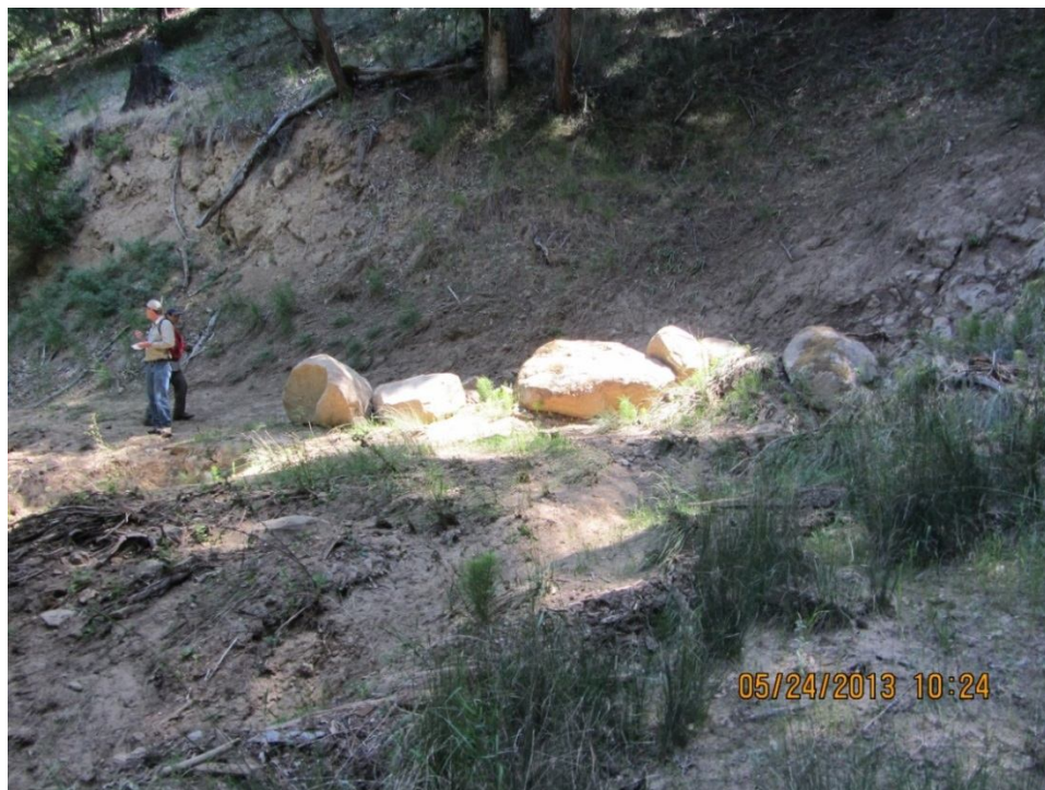
Image 11, May 24, 2013, the road shown in the previous photo at the watercourse crossing. Note the boulders deposited by the flood on the road bench and the extensive flood debris field.
