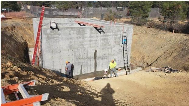
The construction of the Aeromod activated sludge process unit. The Aeromod treatment unit has had all the forms removed and is currently being water tested. Photo by Roy O'Connor.
