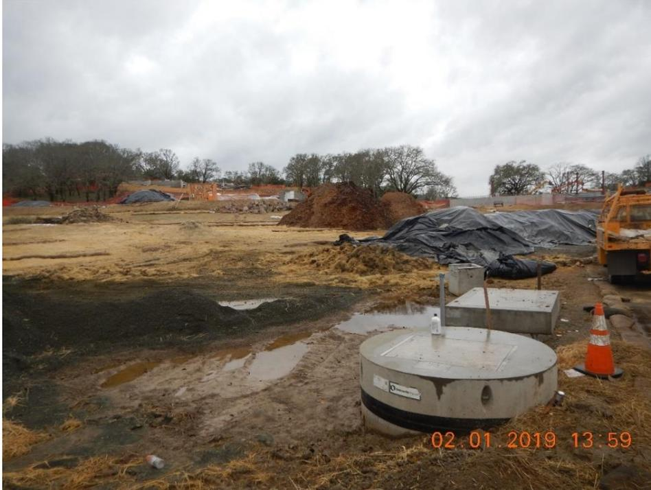
*Figure 28. Stockpiles, some covered, some uncovered. Discolored water. Heavy equipment tracks in the mud.*
