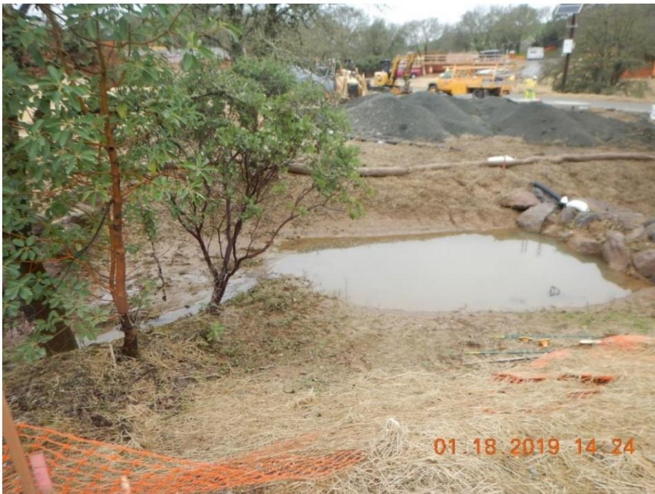
*Figure 21. Uncovered stockpile near top of a stream/drainage channel bank. Creek in the foreground.*
