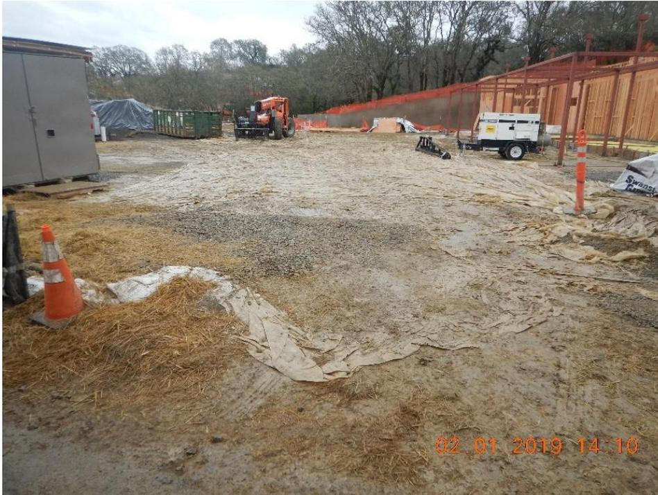
Figure 31. Ineffective erosion and lack of sediment controls in this inactive area.
