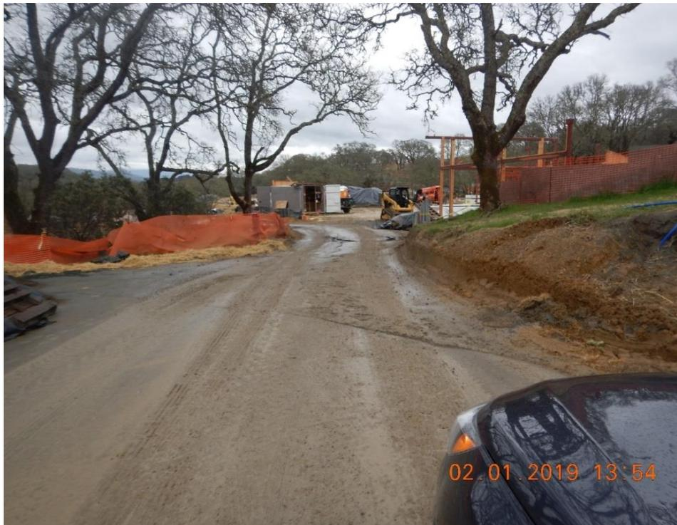
*Figure 34. The cut slope adjacent to the roadway lacks erosion or sediment control measures either on the slope or at its toe.*
