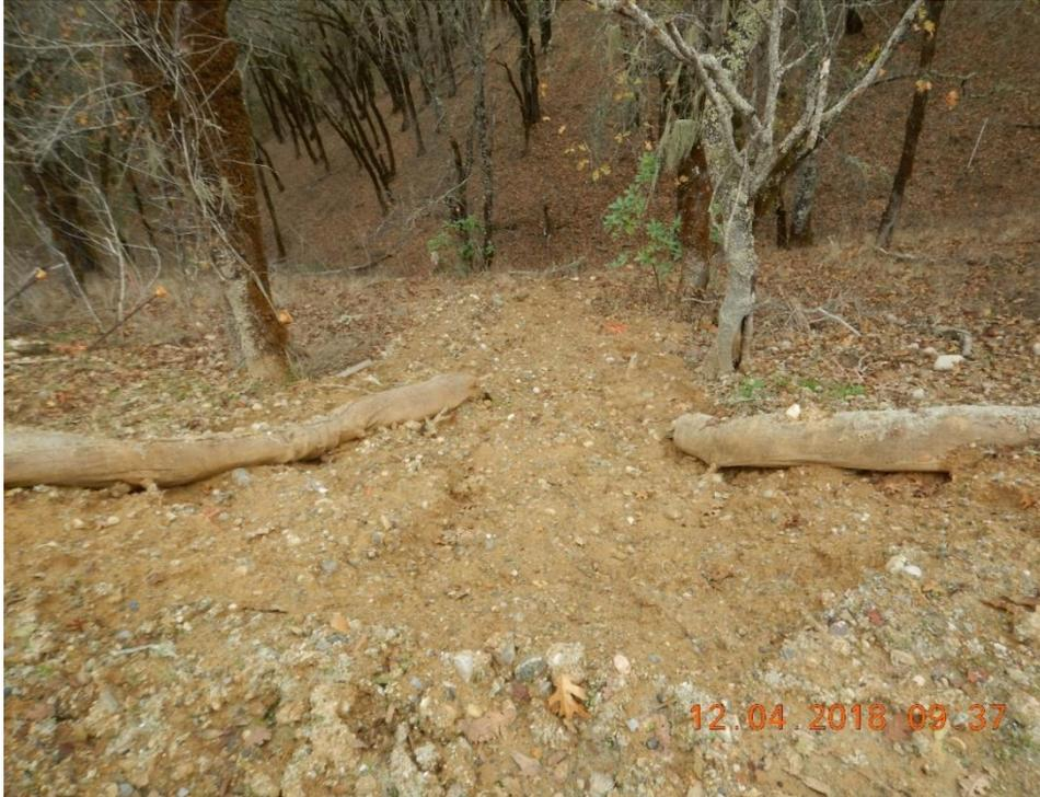
*Figure 8. Sediment from Road 5 has breached the single perimeter wattle and discharged to the hillslope below. An unnamed tributary to Foss Creek is located approximately 75 feet downslope.*
