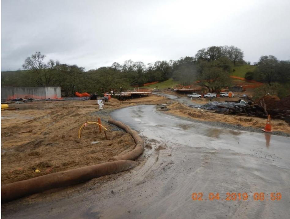
*Figure 36. Poor maintenance of BMPs, and lack of BMPs to keep the paved roads clean continues to result in discharges of sediment-laden runoff to the drainage system.*
