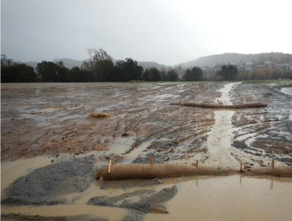
*Figure 6. Ineffective Sediment control BMPs resulting in turbid, sediment-laden storm water runoff.*
