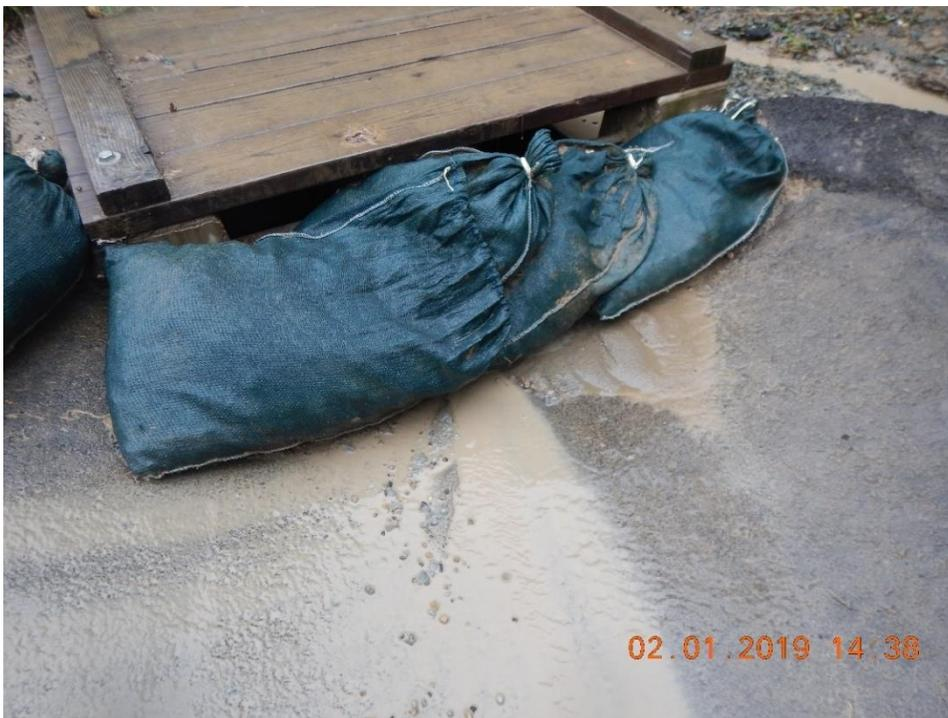
*Figure 35. This check dam is not correctly positioned to effectively capture or remove pollutants from storm water runoff.*
