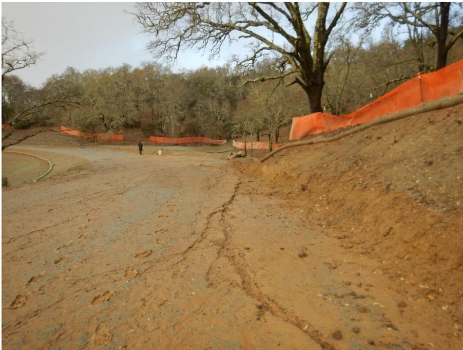
*Figure 10. No linear sediment controls along the base of this roadside slope. Signs of gullying on the road.*
