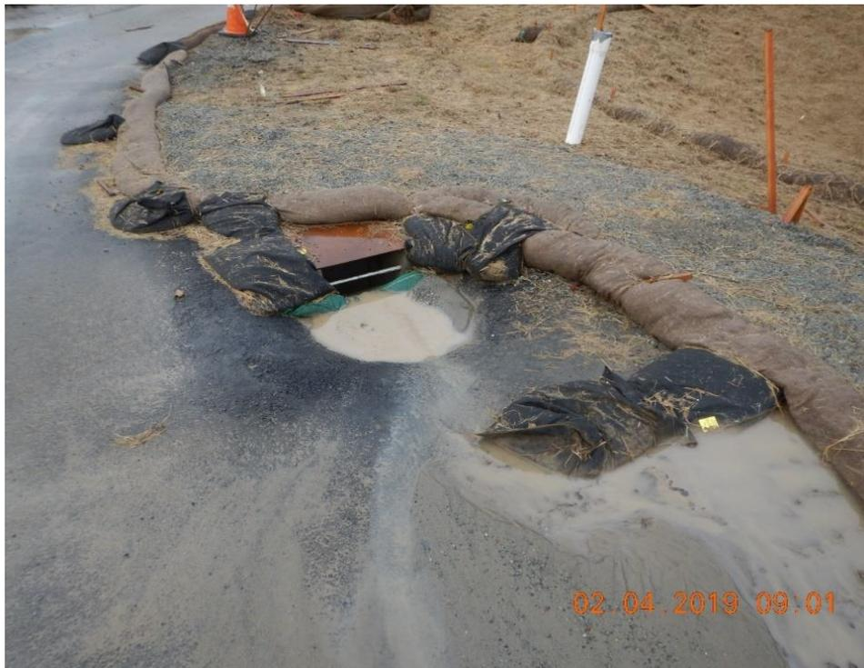
*Figure 39. Sediment controls near the drainage inlet are not effectively reducing or preventing pollutants in storm water discharges.*
