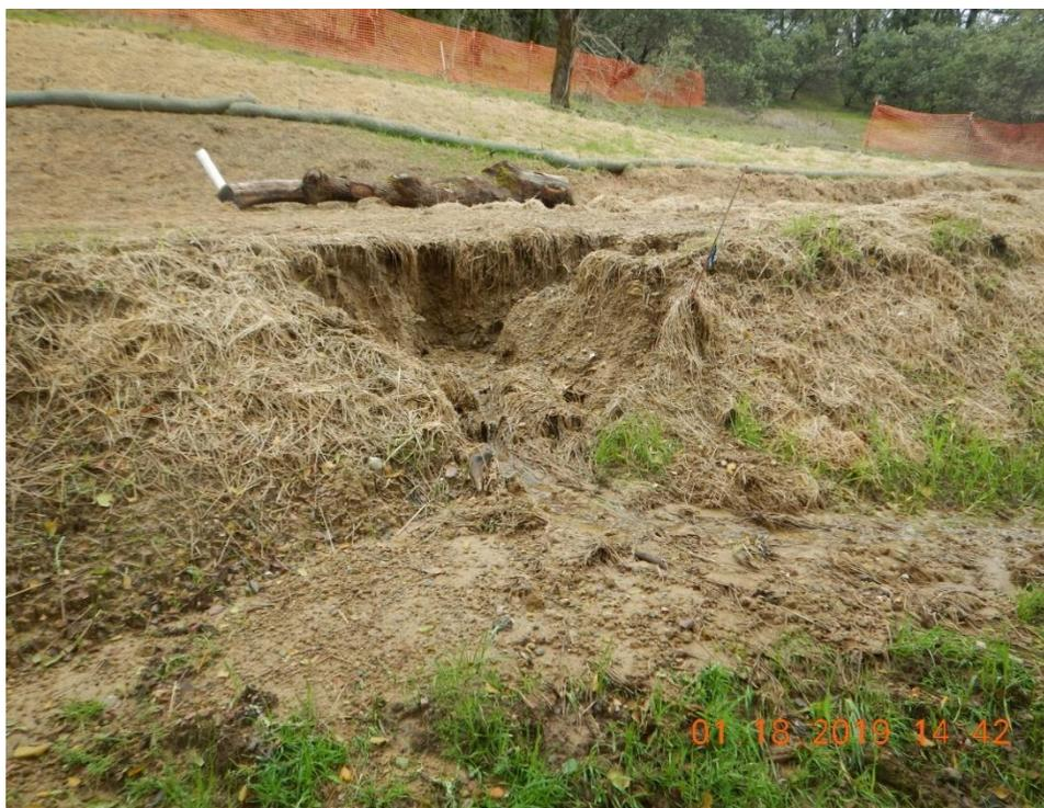
*Figure 23. Ineffective erosion and sediment controls on slope resulting in bank failure and evidence of sediment transport in the foreground.*
