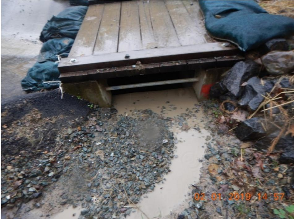
*Figure 27. Turbid storm water runoff entering drain inlet that discharges to Foss Creek*
