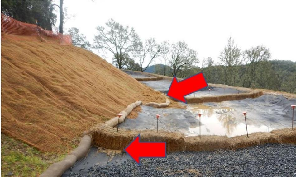
*Figure 41. Note slumping slope on roadway. Turbid water is visible emerging from the left side of the first straw bale berm in the foreground. This turbid water eventually discharged to an unnamed tributary to Foss Creek.*
