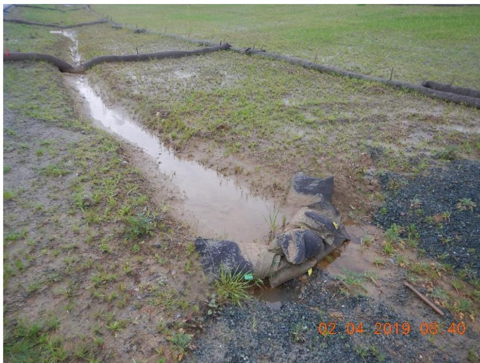
*Figure 37. Erosion controls (hydroseed and straw soil cover) are not adequate or established enough to prevent sediment-laden runoff to the storm drain system that discharges to Foss Creek.*
