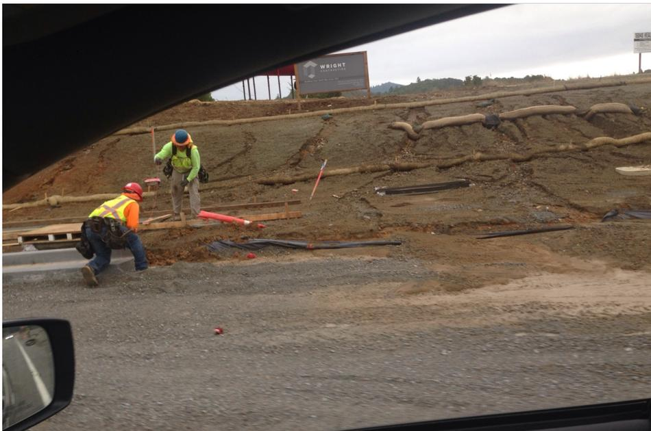
*Figure 2. View of failed BMPs. Insufficient ground cover, and sediment in street (Healdsburg Avenue) after storm event. Photograph taken on October 3, 2018.*
