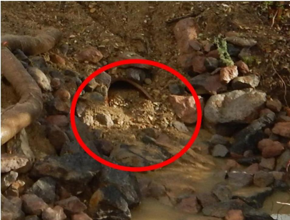
*Figure 15. Significant sediment discharge at the culvert outfall that drains the upper resort area.*
