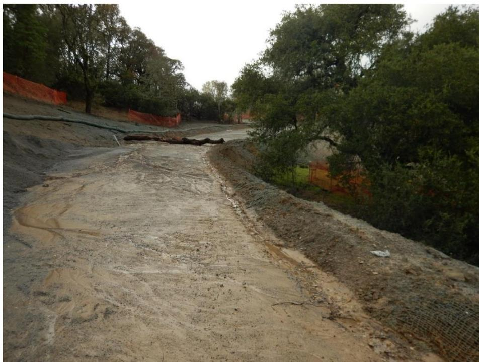
*Figure 13. Road segment with adjacent unprotected slope and signs of uncontrolled runoff.*
